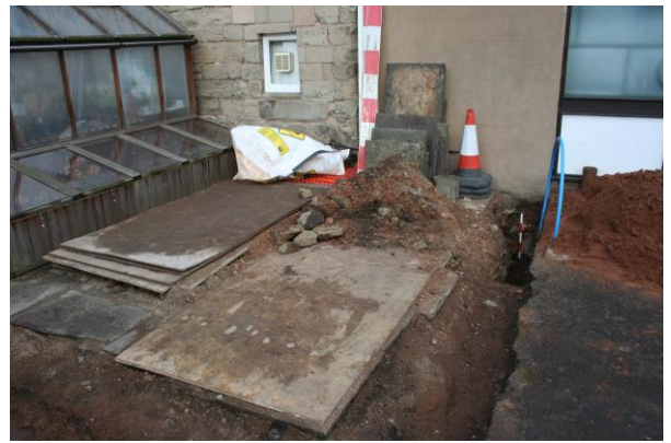
Fig. 5: Wall 9 location looking north-east
