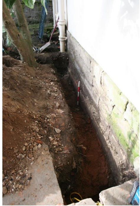
Fig. 3: Wall 8 location looking south-west
