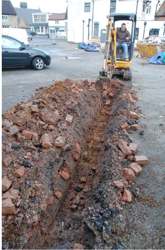
Fig 5: Service trenches looking north
