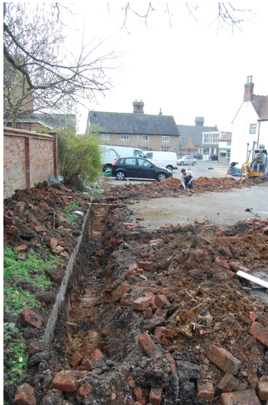
Fig 6: Service trenches looking west
