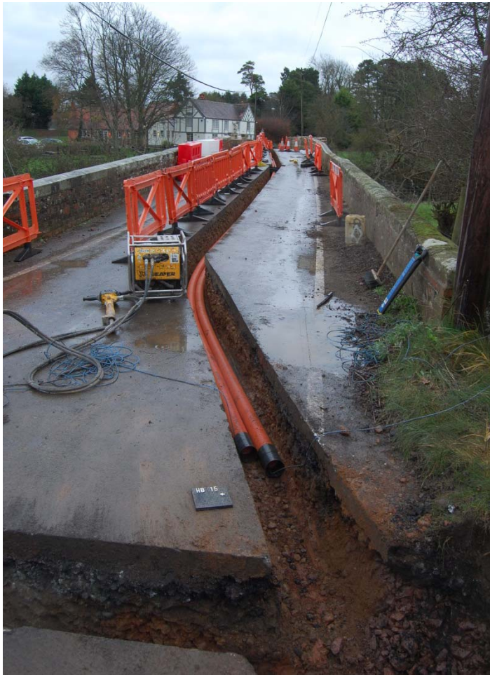
2. Service trench with conduits in place
