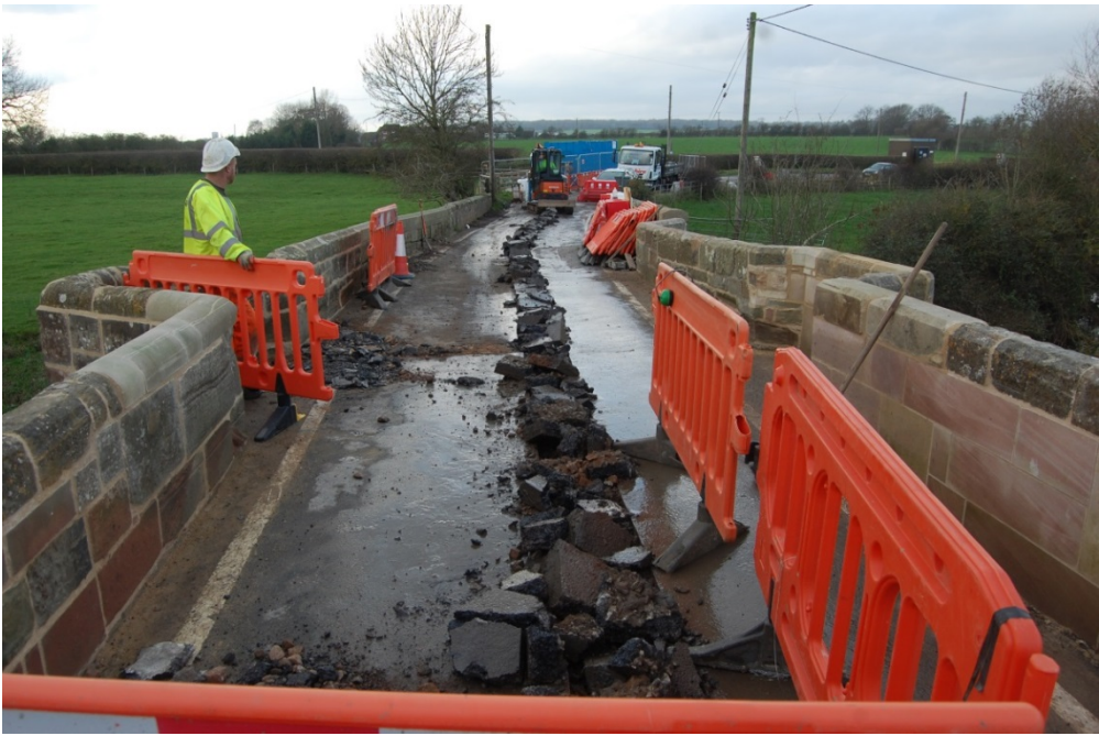
1. Breaking through the tarmac surface
