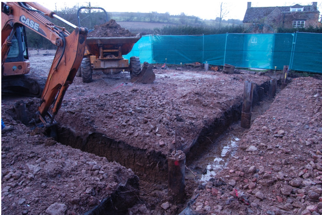
Fig 3: Ground beam trenches
