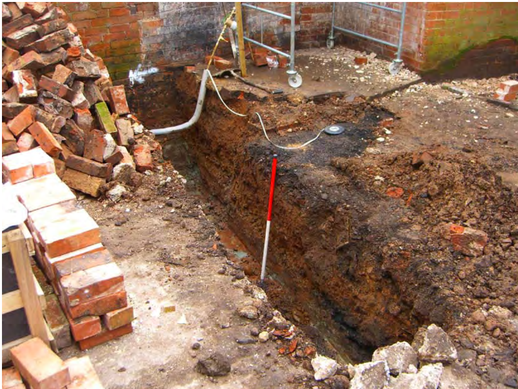
Fig. 8: Foundation trench east of Brook Cottage, view south
