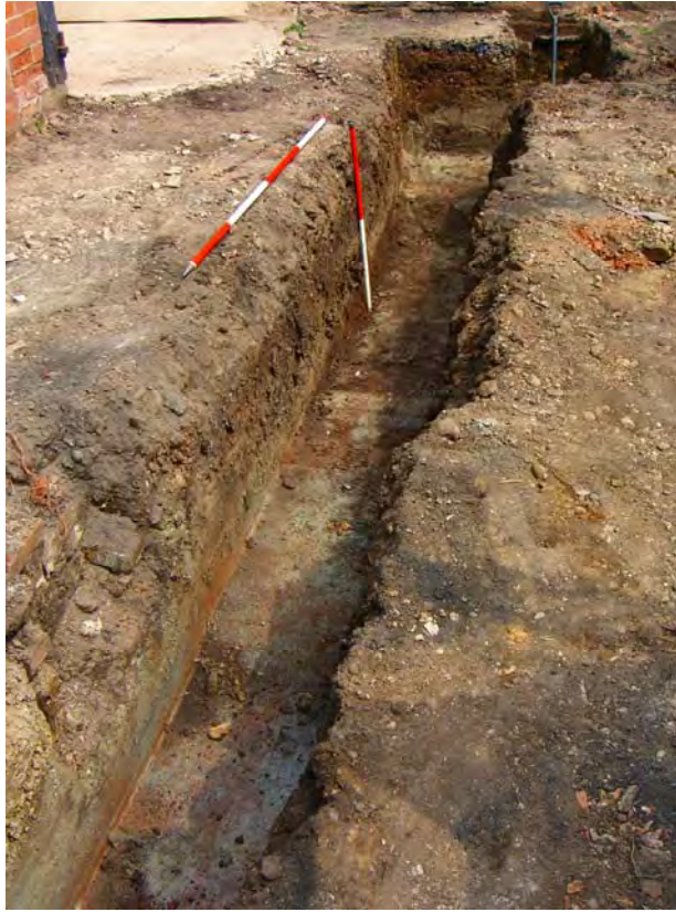
Fig. 7: Foundation trench south of barn, view north-east
