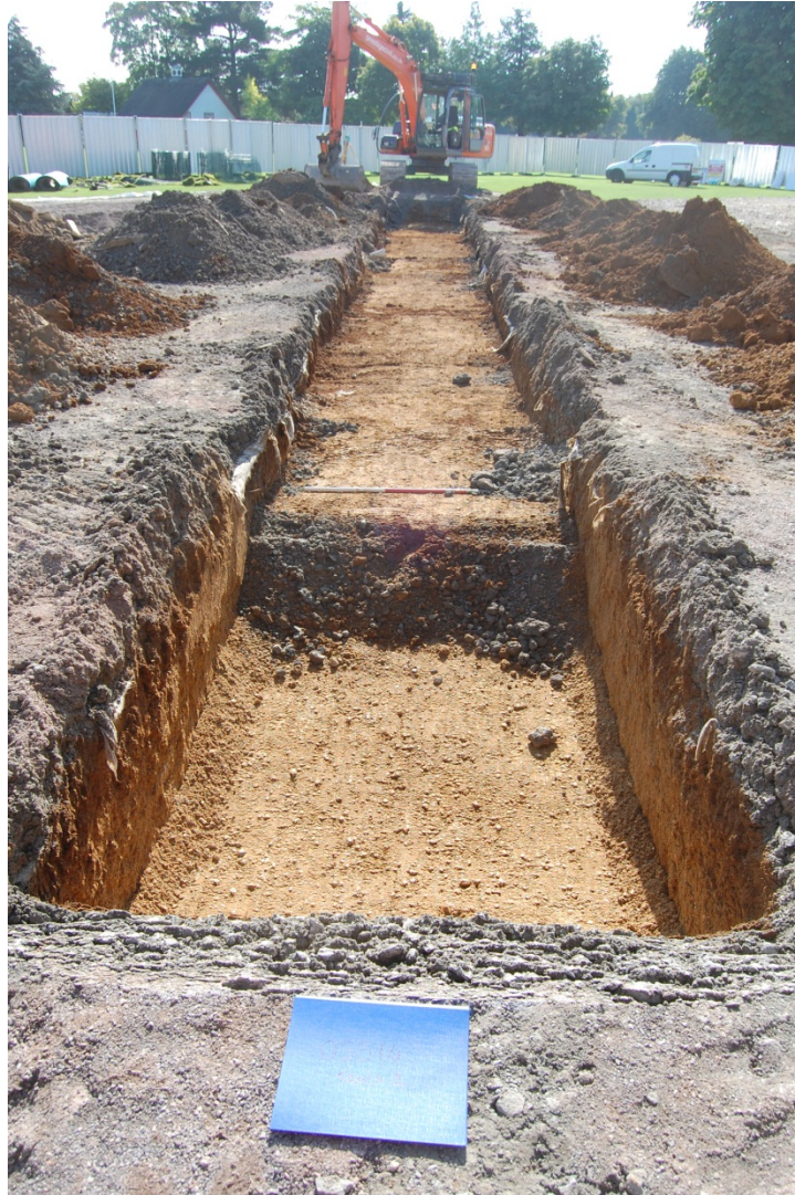
Fig 4: Evaluation trench looking south-east
