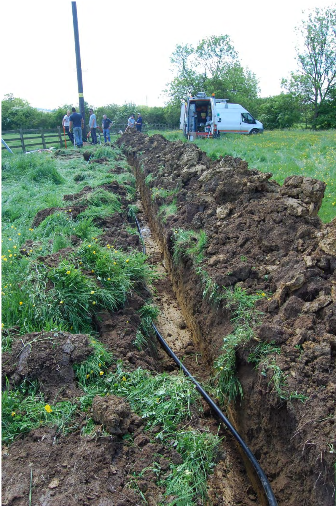
Fig 4: General view of trench excavations
