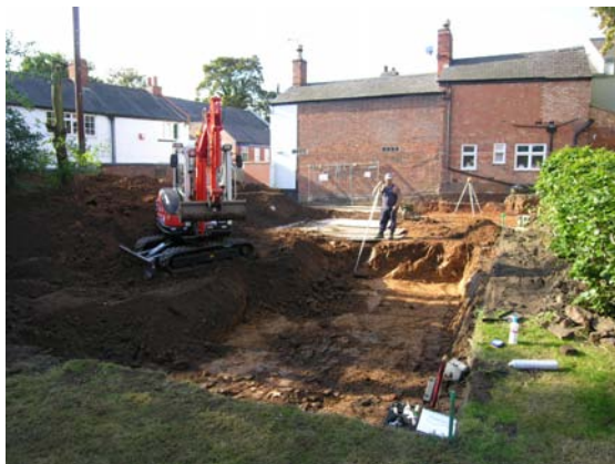
Fig. 6: Area observed, looking north-west
