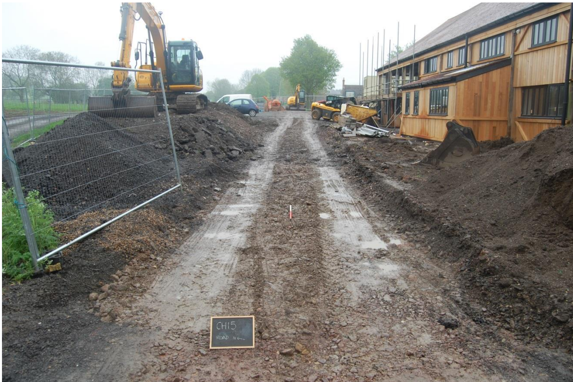
4 Grubbed out old road
