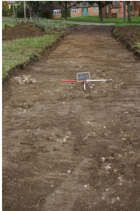
1 New road stripped
