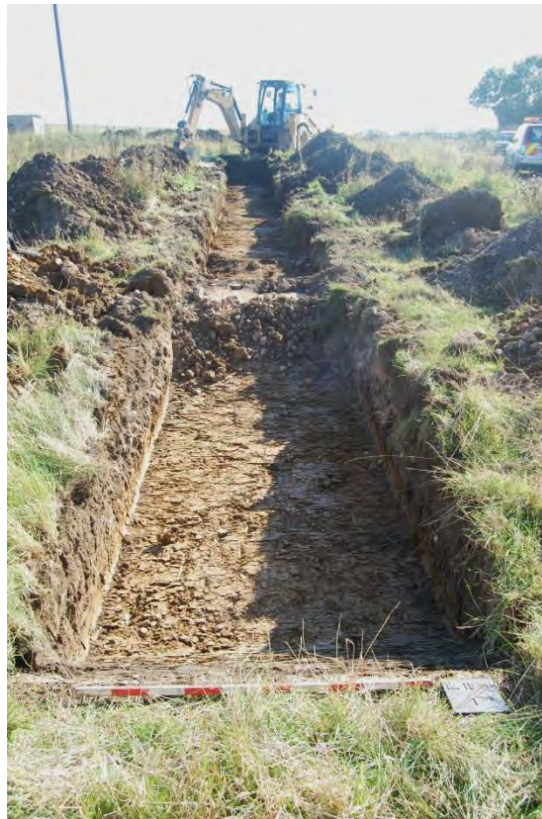
1. Trench 1 looking south
