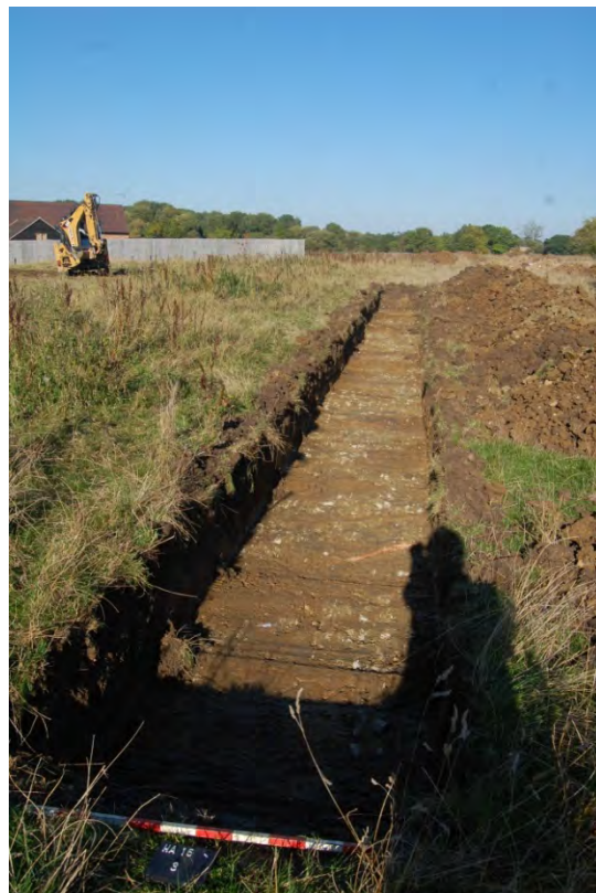
4. Trench 3 looking north-east
