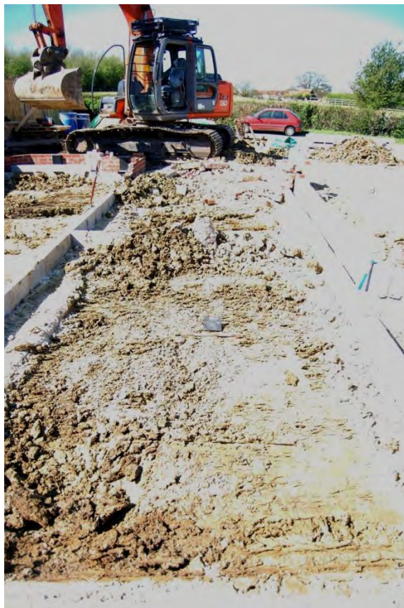
Photograph 3. Cleaning between foundations
