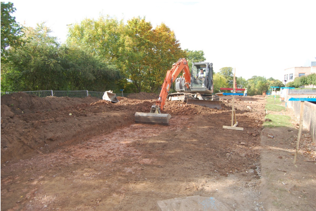
Fig 4: Ground reduction for road
