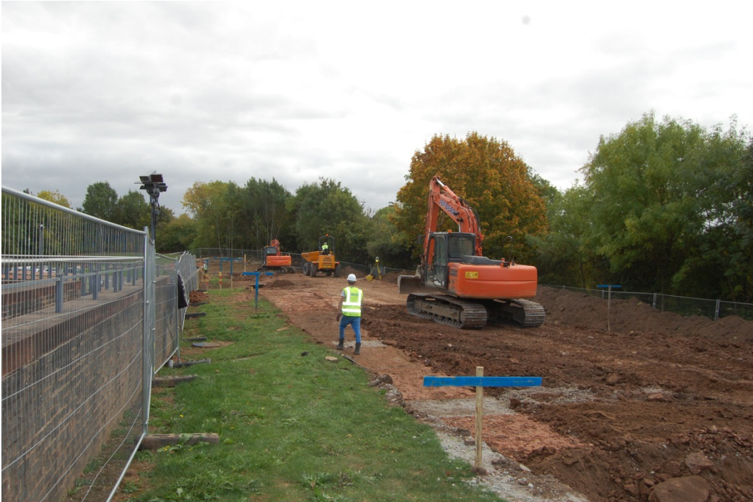
Fig 3: Ground reduction for Car Park in progress
