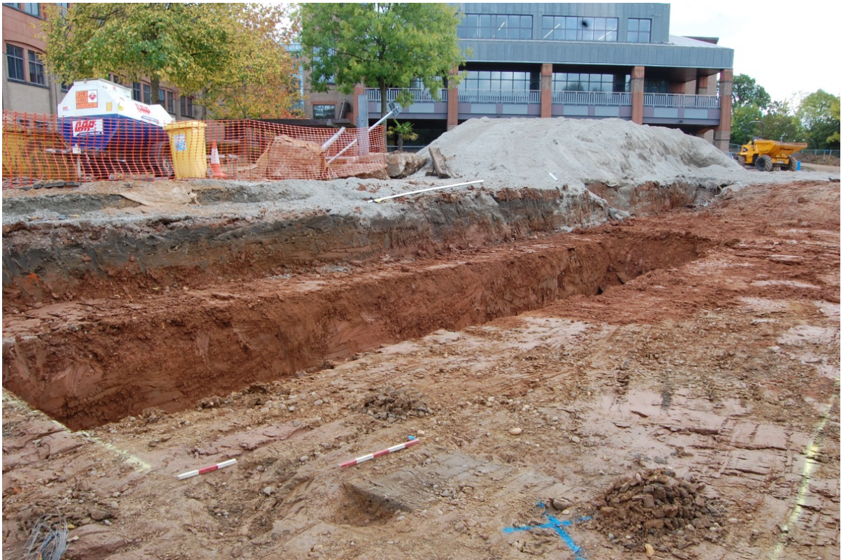
Fig 5: Tank excavations in progress
