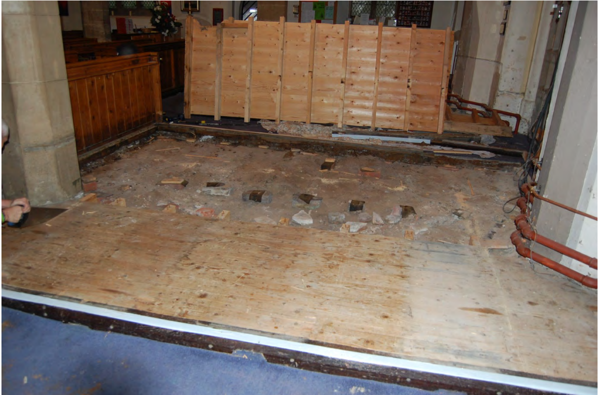
Fig 8: View of sub-floor material and joist supports
