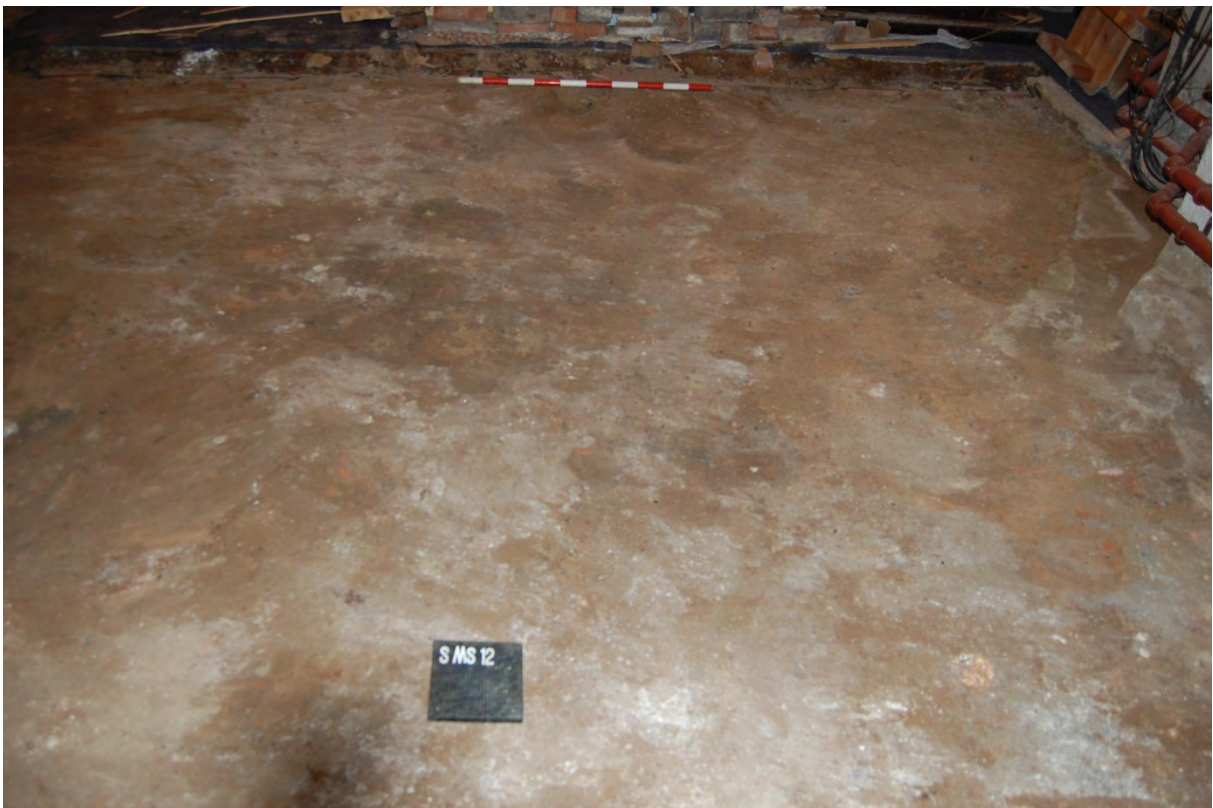
Fig 9: Sub-floor cleaned of loose material
