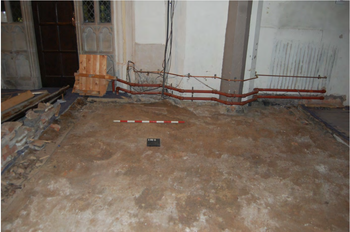
Fig 10: View of pier with stone slabs (5) below
