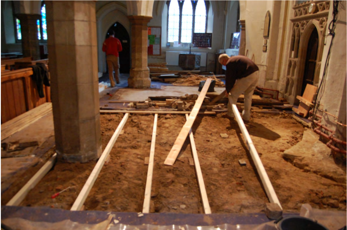
Fig 12: New joists being laid
