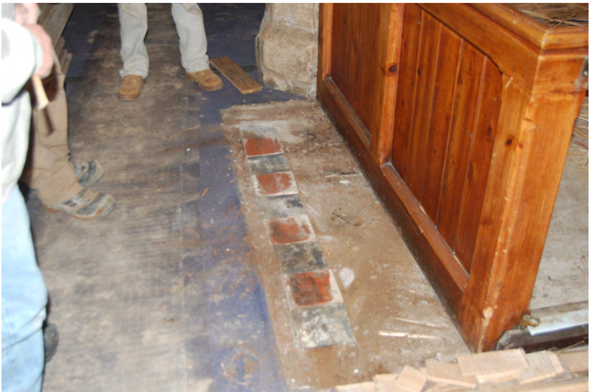
Fig 11: Victorian quarry tile floor (8)
