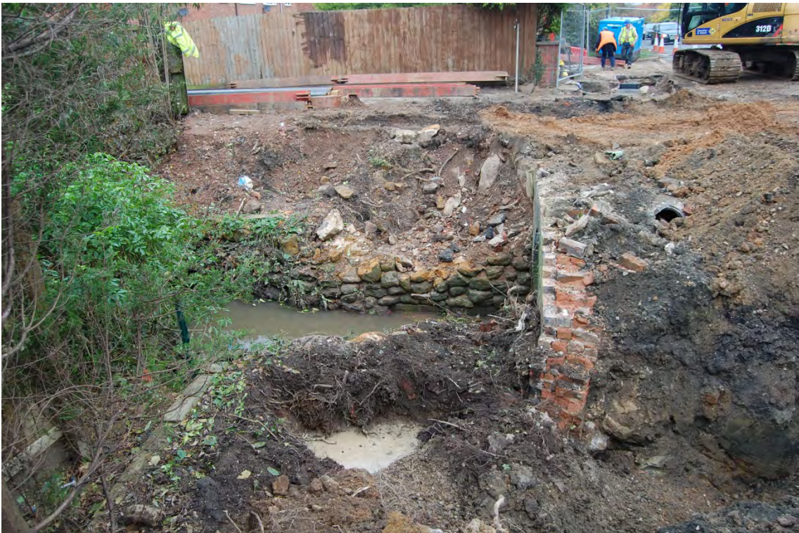
Fig 13: Western edge of bridge during excavations
