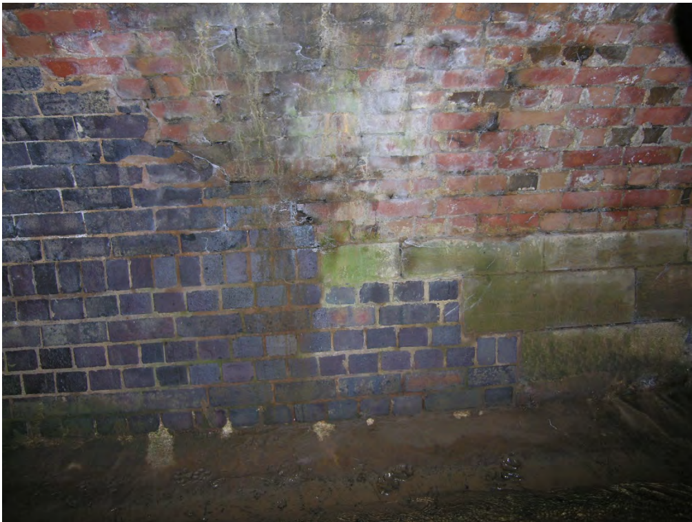
Fig 6: Red brick phase of bridge arch
