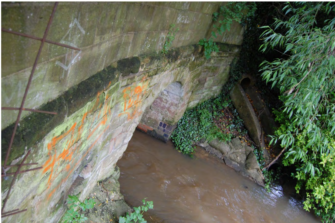
Fig 9: Eastern end of bridge prior to works
