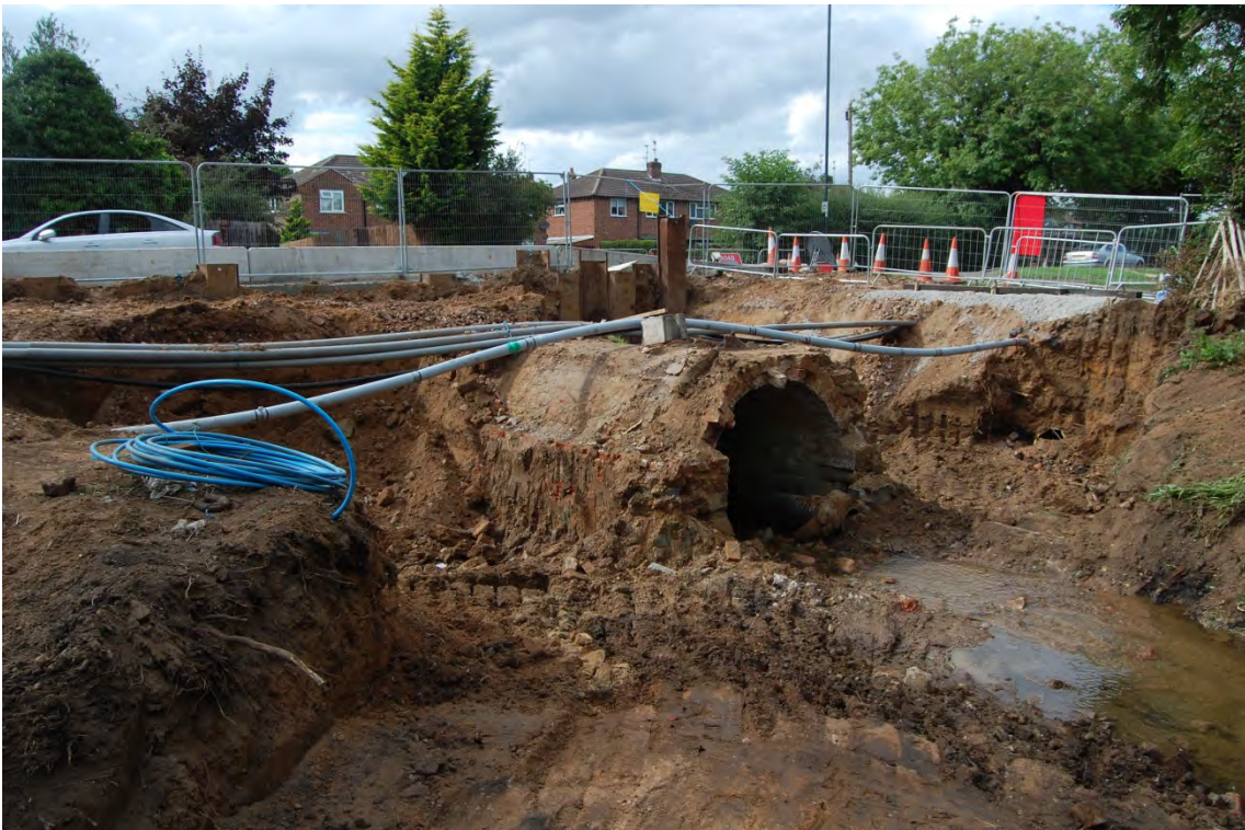
Fig 11: Ground reductions at eastern end of bridge
