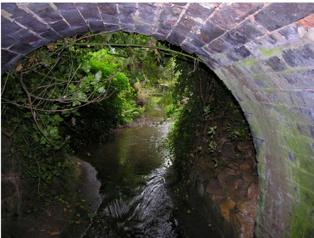
Fig 7: Western end of bridge arch; 2 nd phase of bridge extension
