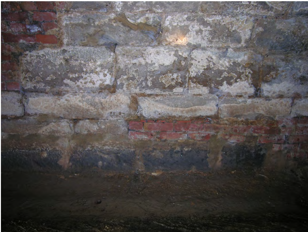
Fig 8: Tile used in repair
