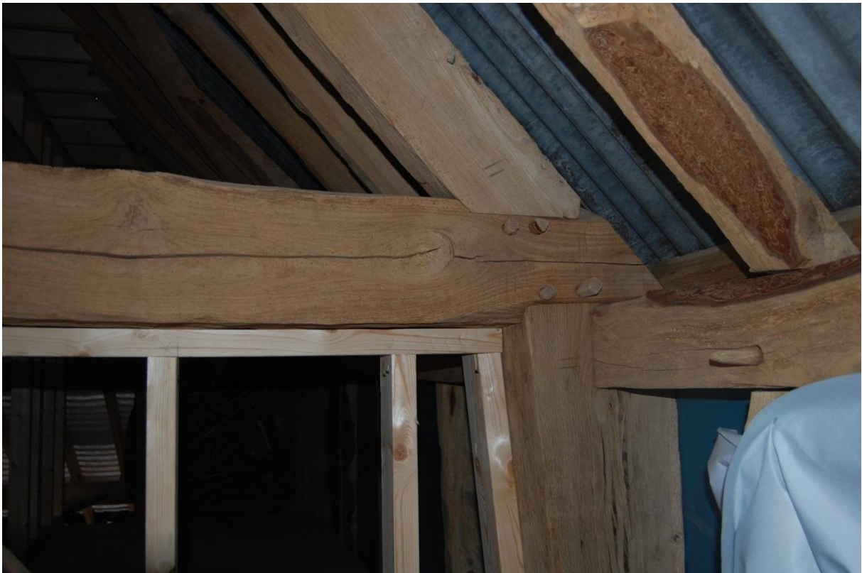
10: Carpentry marks and bark on timbers
