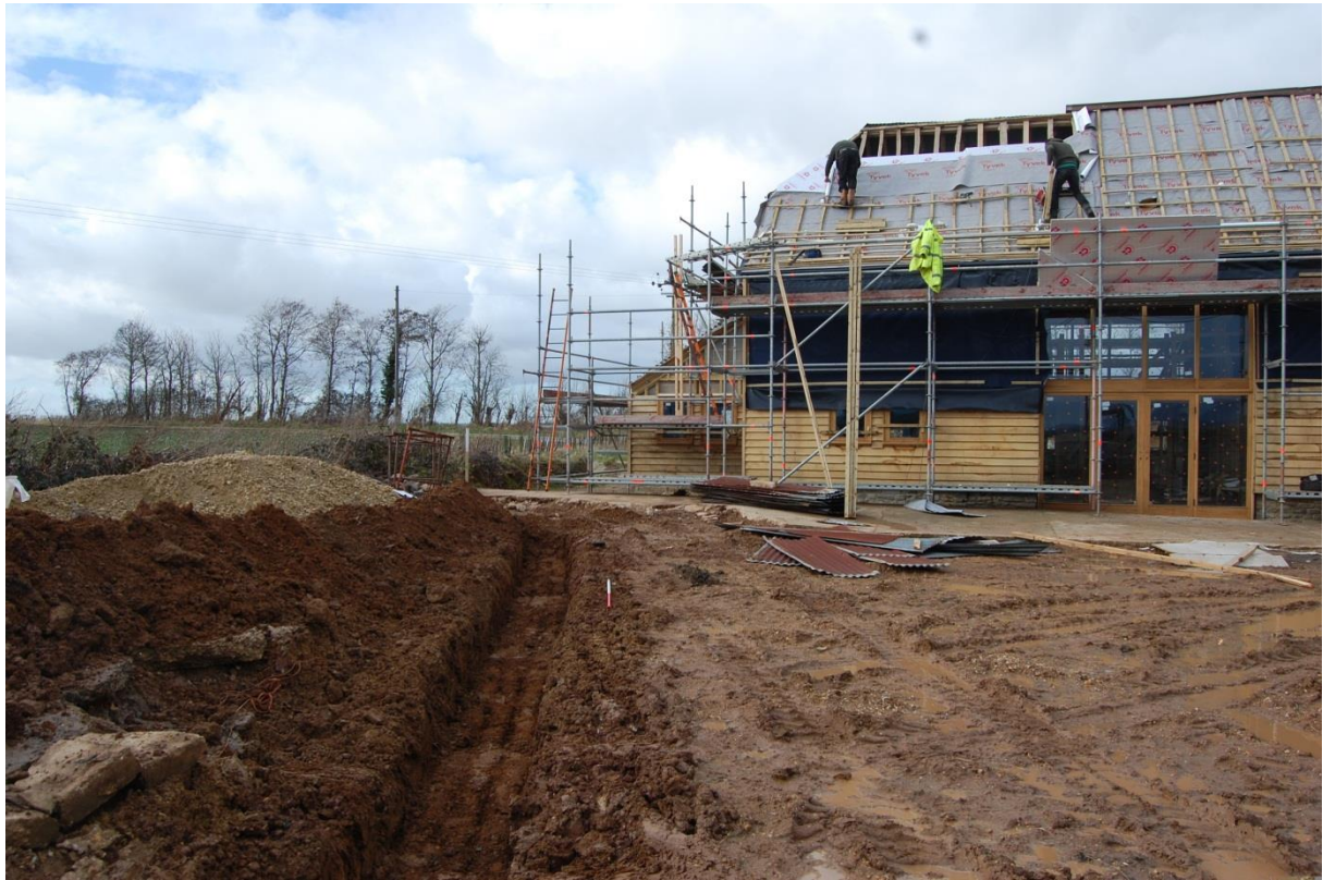
21: Service trench across courtyard
