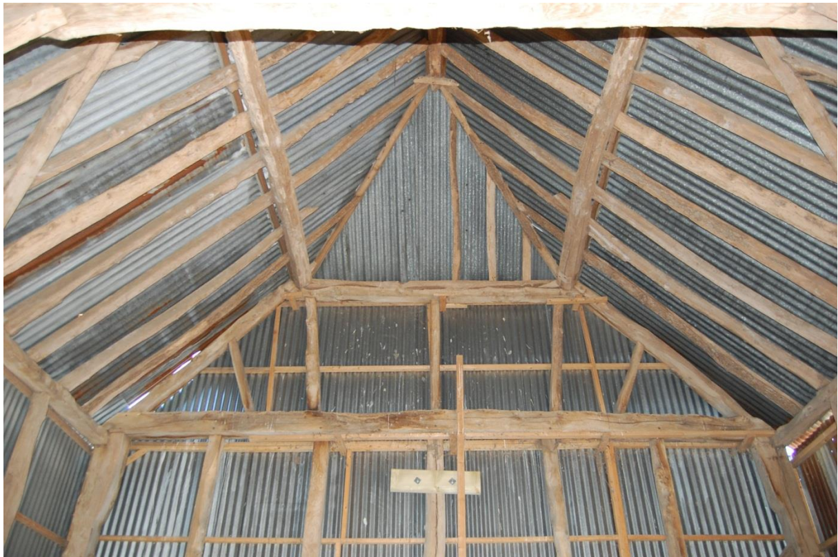
6: North-east half-hipped gable
