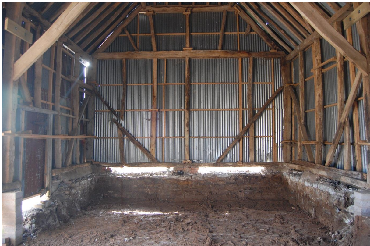
18: Ground reduction showing below-ground extent of plinth wall at south-west end of barn
