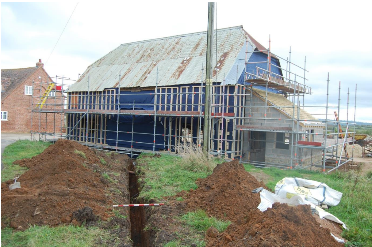
20: Service trench to the north-west of the barn
