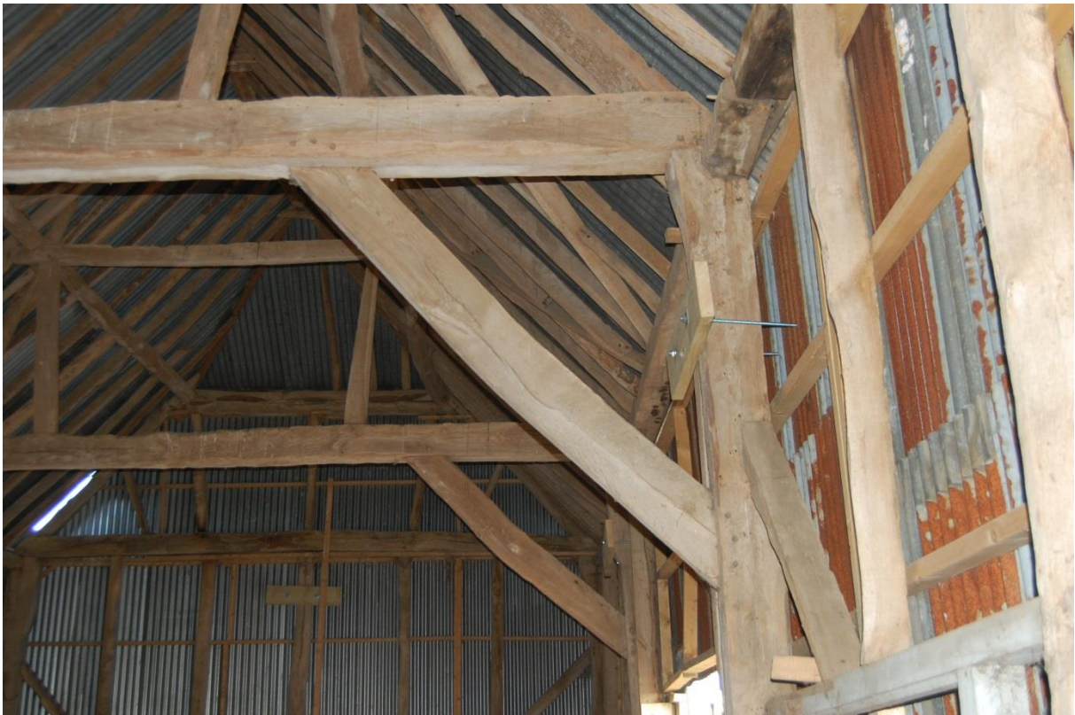
12: Diagonal bracing
