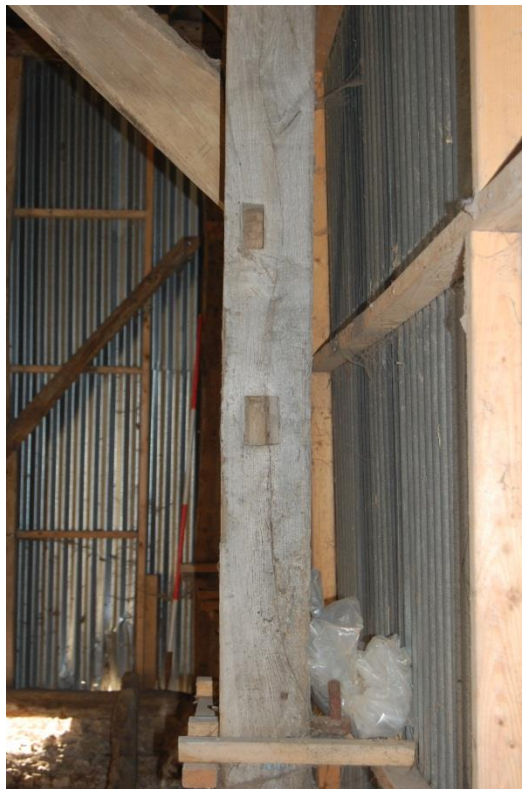
16: Slots for cross-bars on south-east door frame
