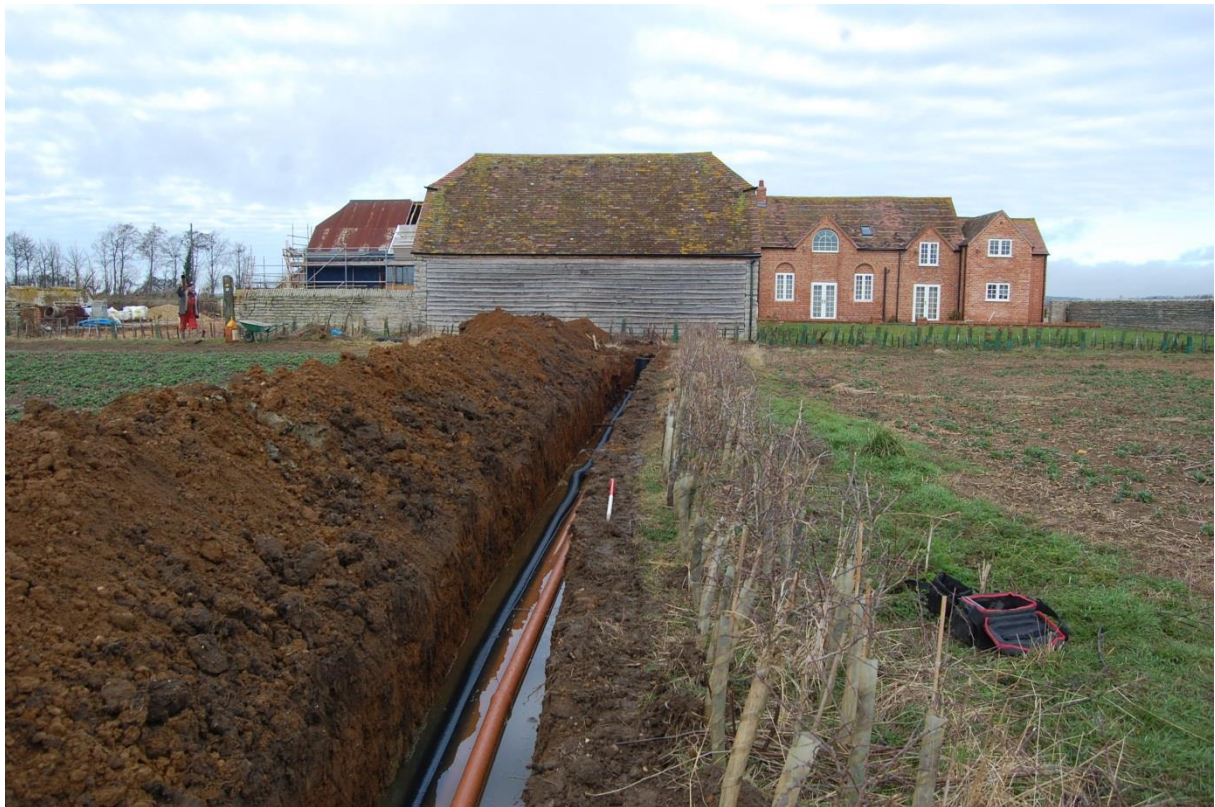
22: Service trench out into field
