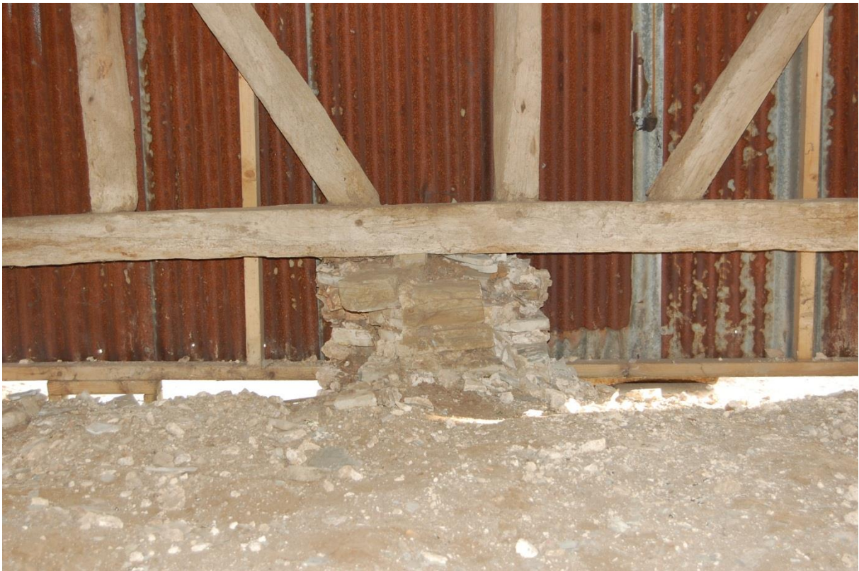
14: Remnant of wall plinth
