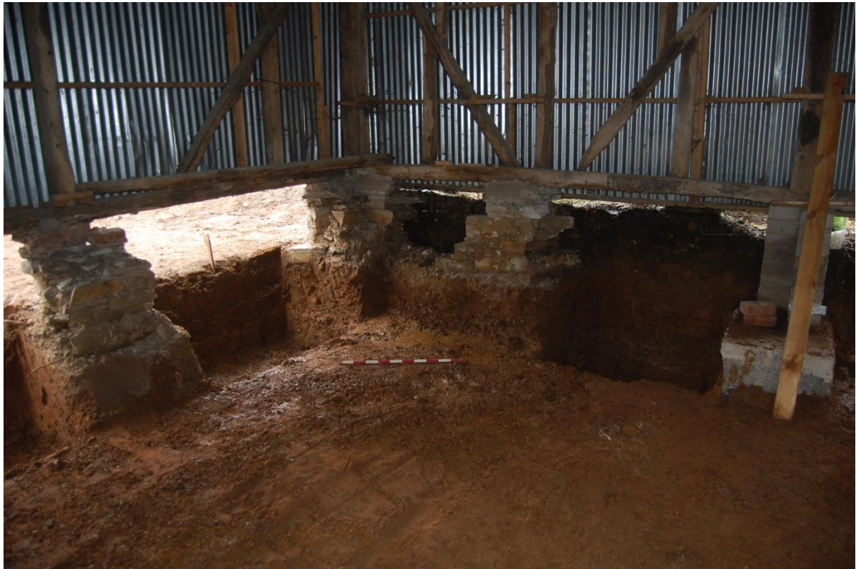
17: Ground reduction in the barn and on the line of the plinth wall
