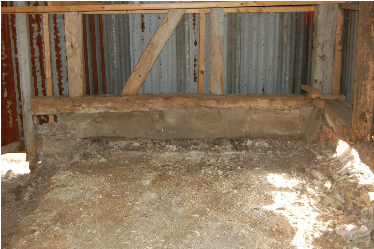
13: Remnant of wall plinth
