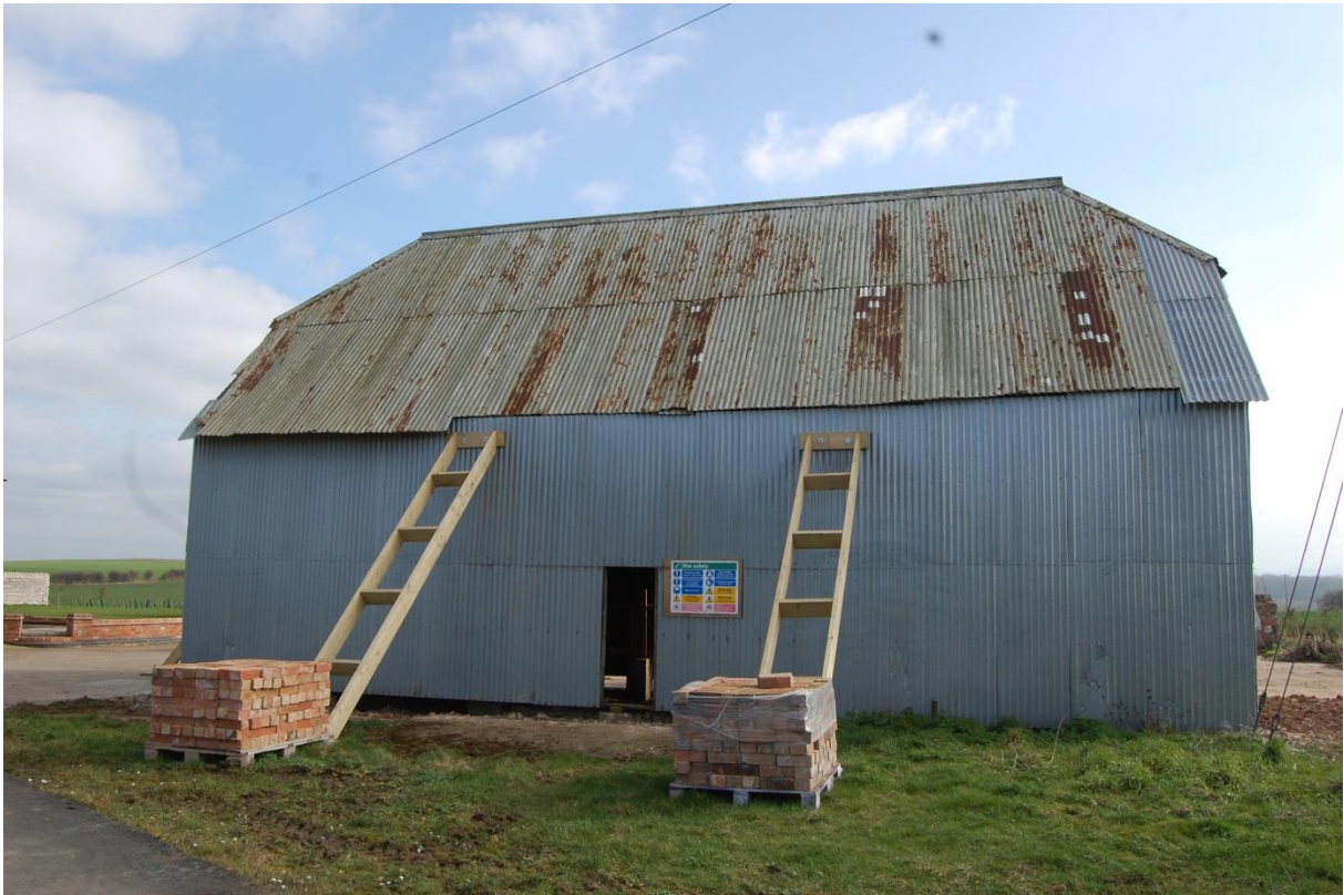
1: The barn with its corrugated iron cladding and roof cover
