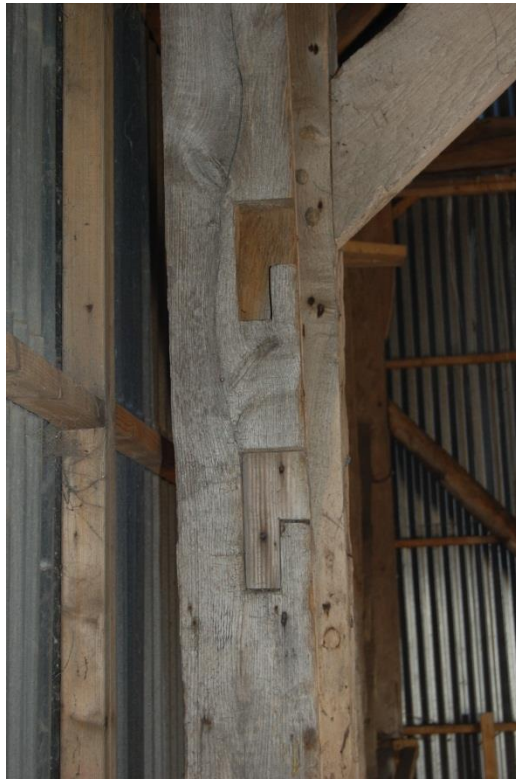
15: Slots for cross-bars on north-west door frame
