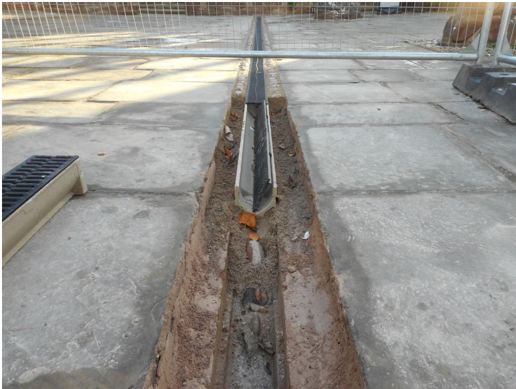
3: Detail of new drain, sitting over old drain channel
