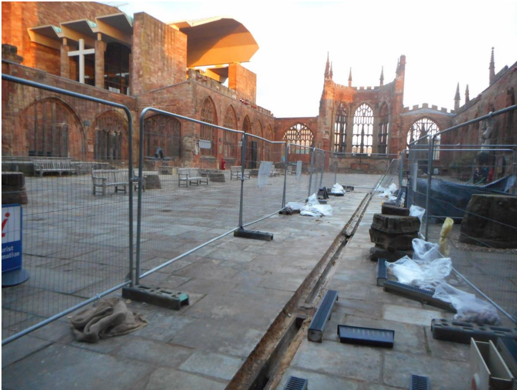
2: Old drain removed and new drain being installed
