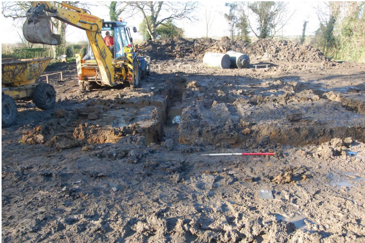
1. General shot of the site
