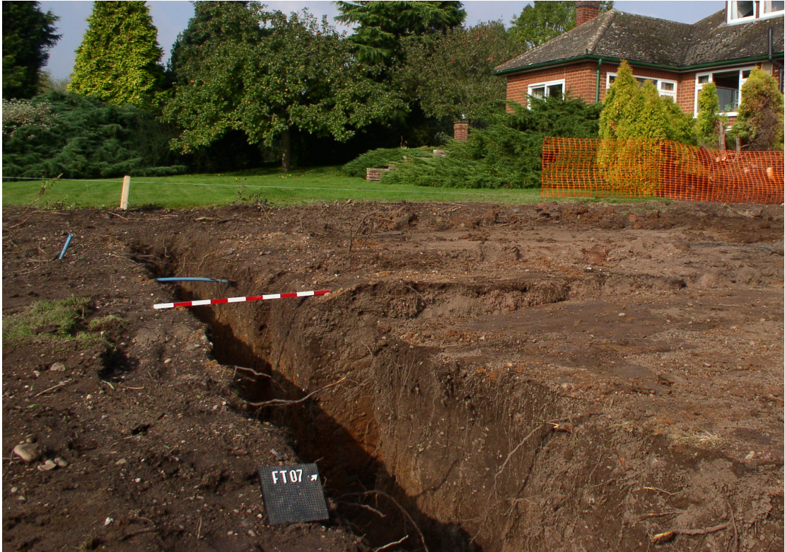
Fig. 7: Foundation trenches looking north-west
