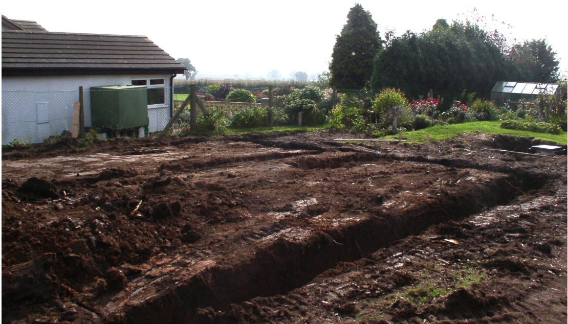
Fig. 8: Foundation trenches looking south-east
