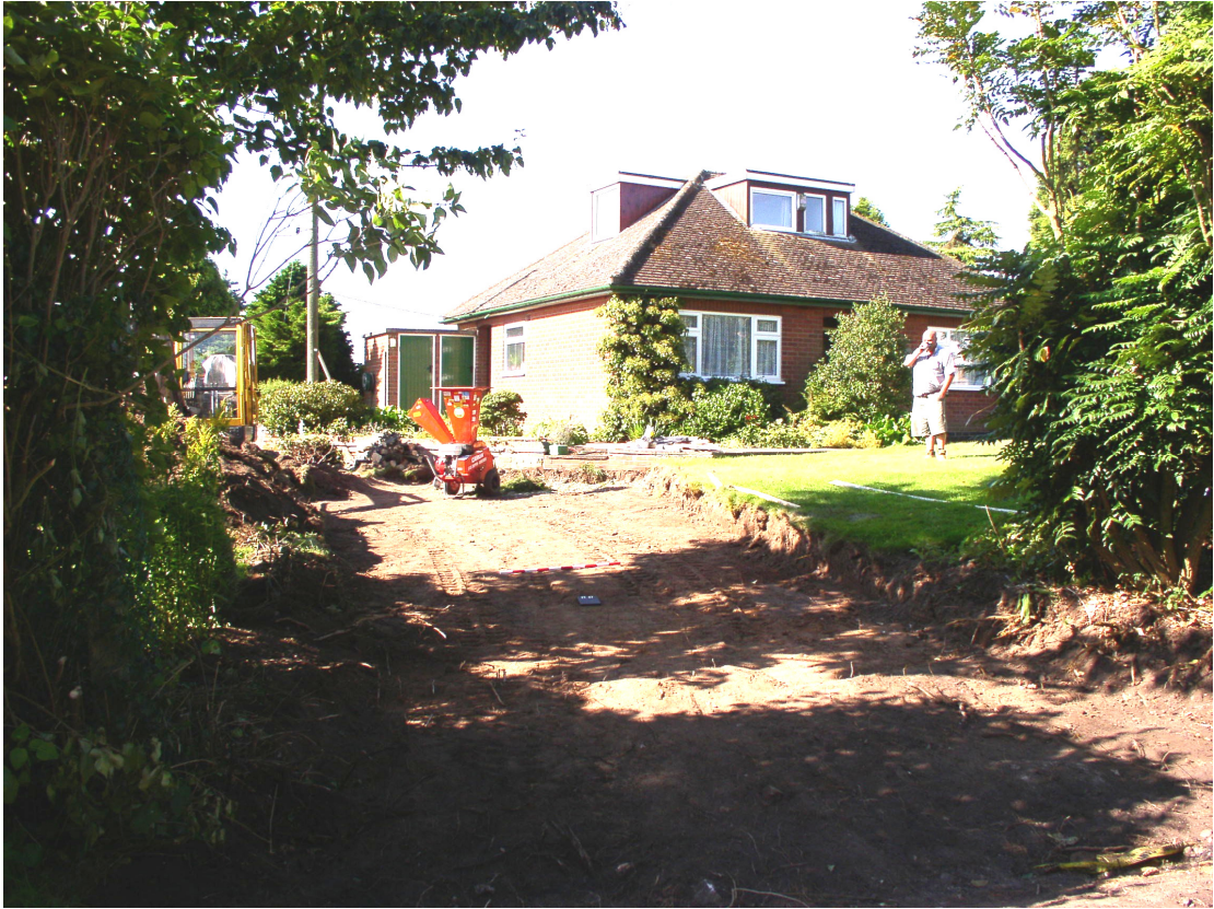
Fig. 5: Driveway looking south-west
