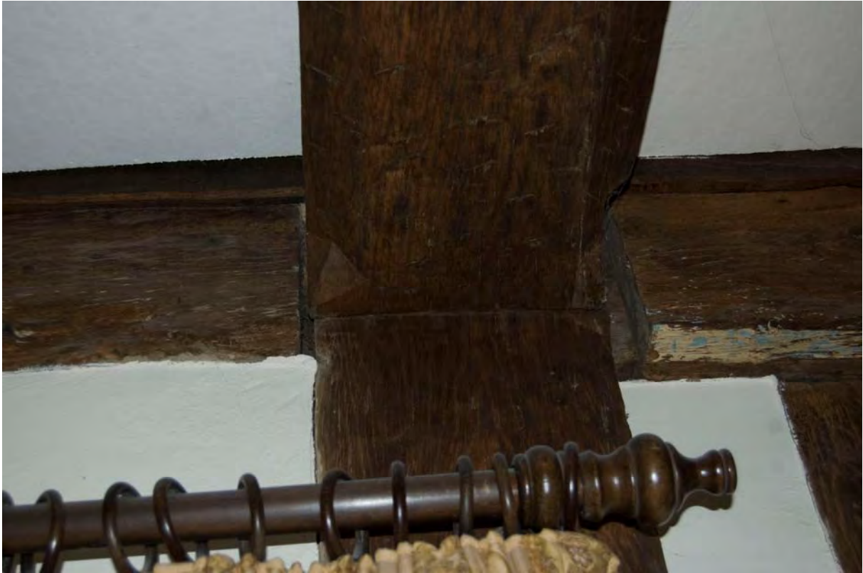
Fig 20: Beam with chamfer stops
