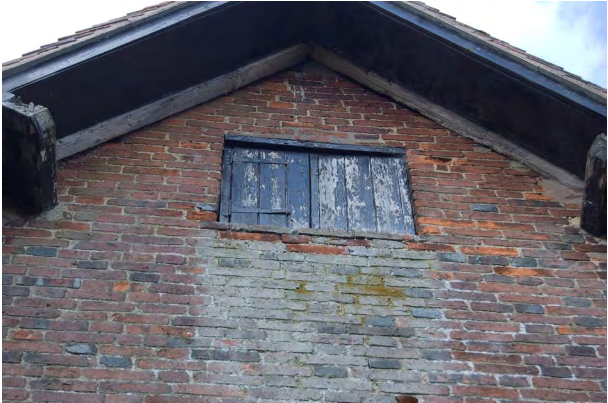
Fig 7: Shuttered window in gable end
