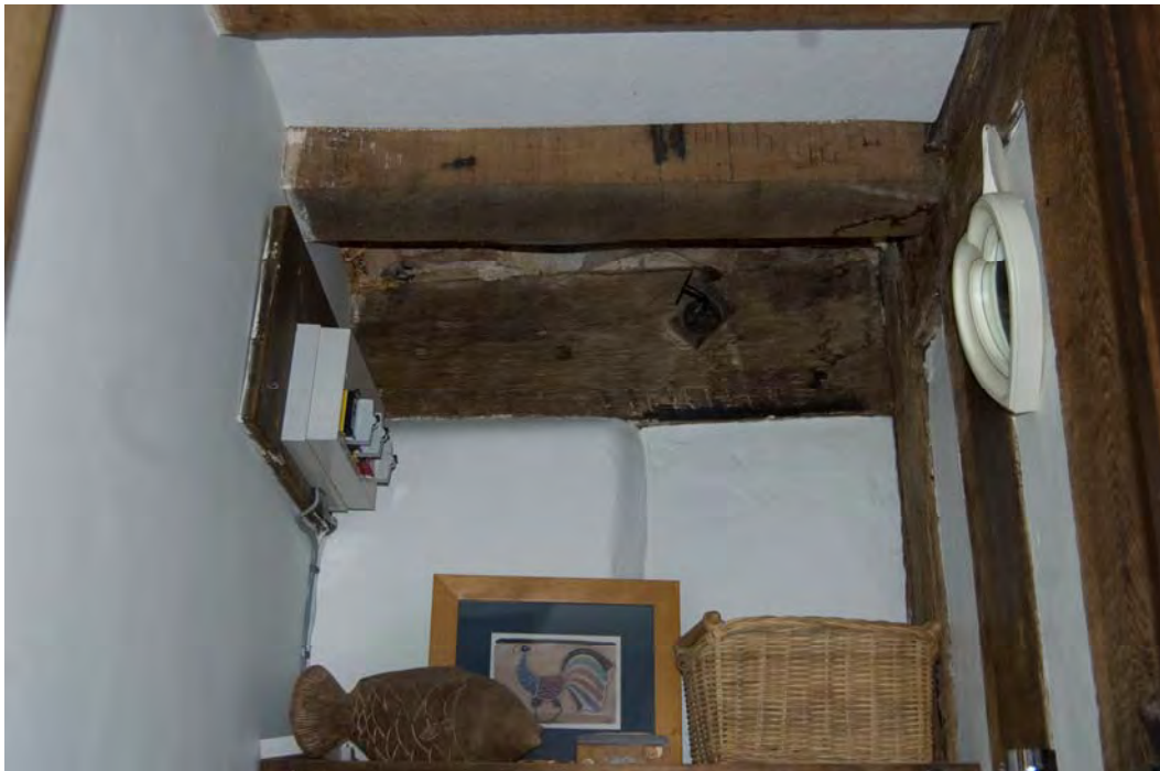
Fig 23: Blocked window and bracket for former stair rail on beam
