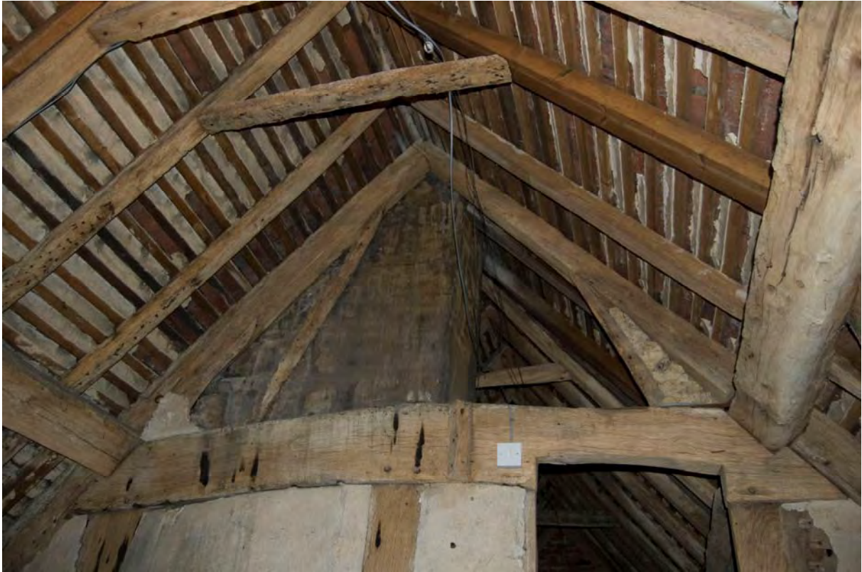
Fig 44: Attic, upper roof timbers
