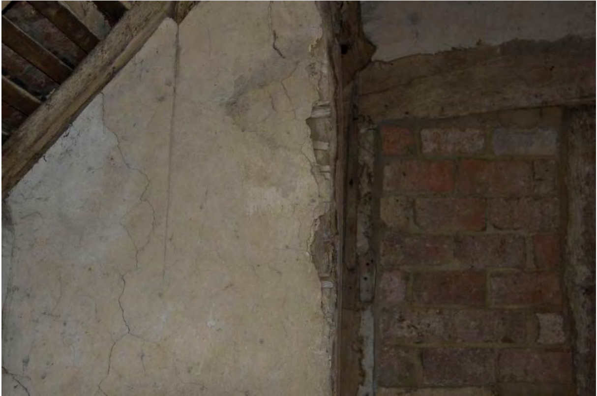
Fig 48: Lath and plaster
