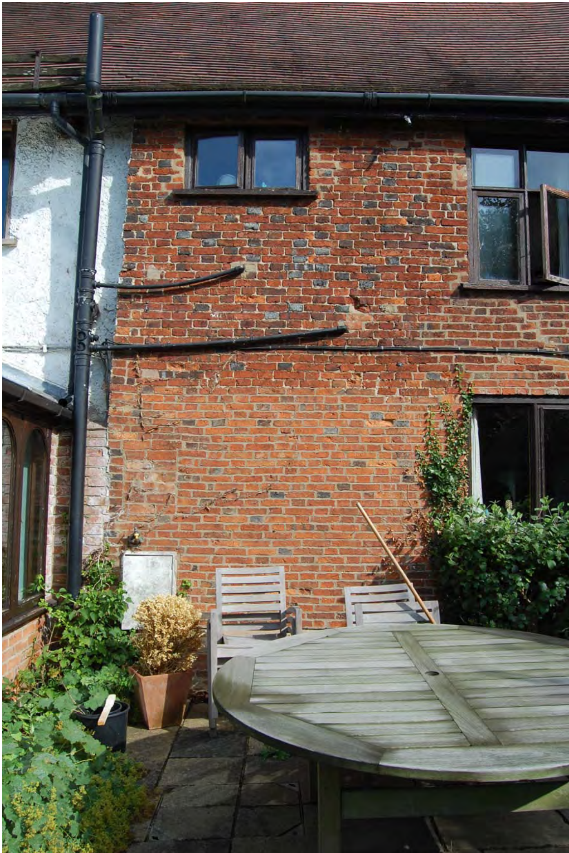
Fig 9: Rear of house showing change in brickwork between ground floor and first floor
