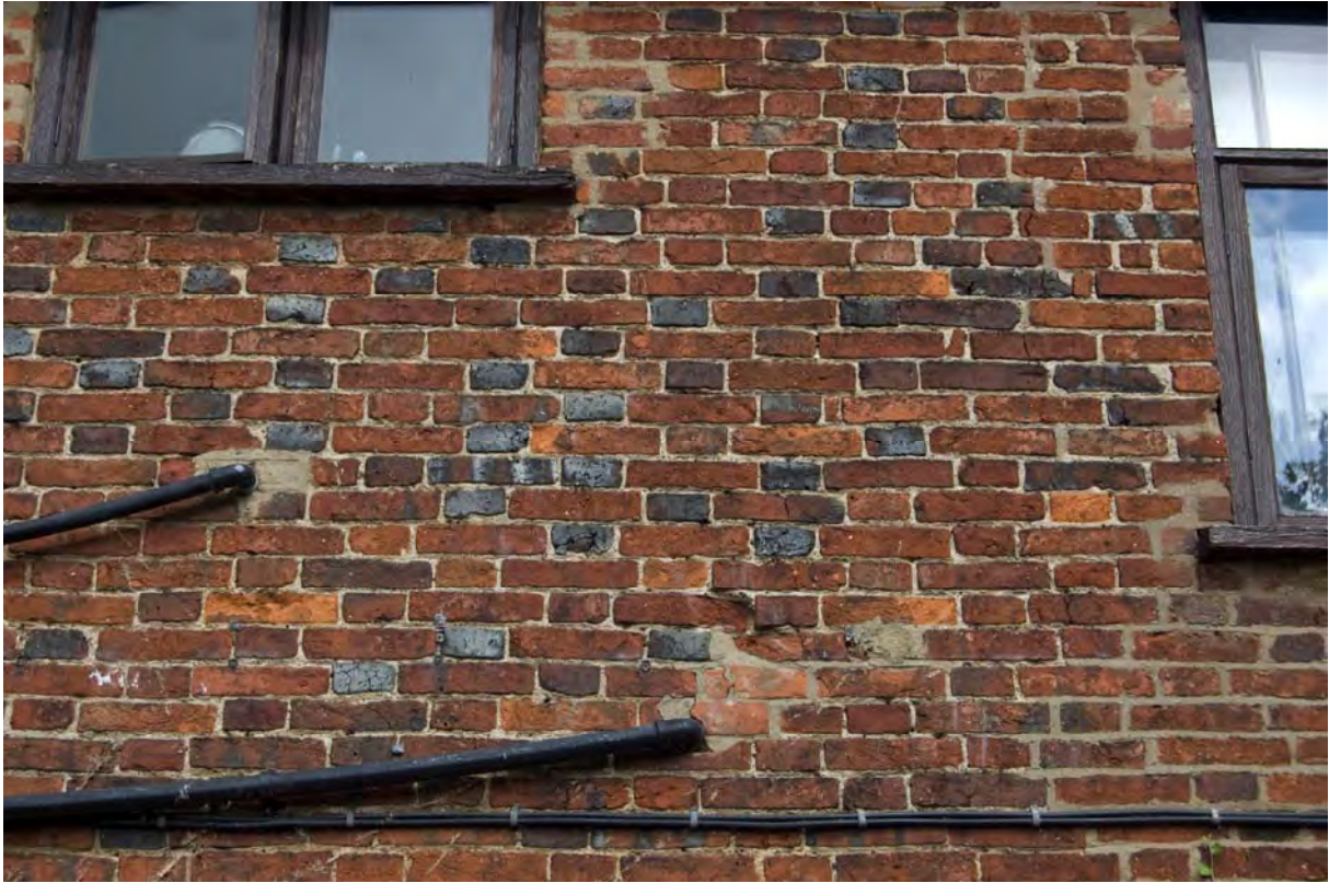
Fig 10: Flemish bond brickwork in upper part of rear wall
