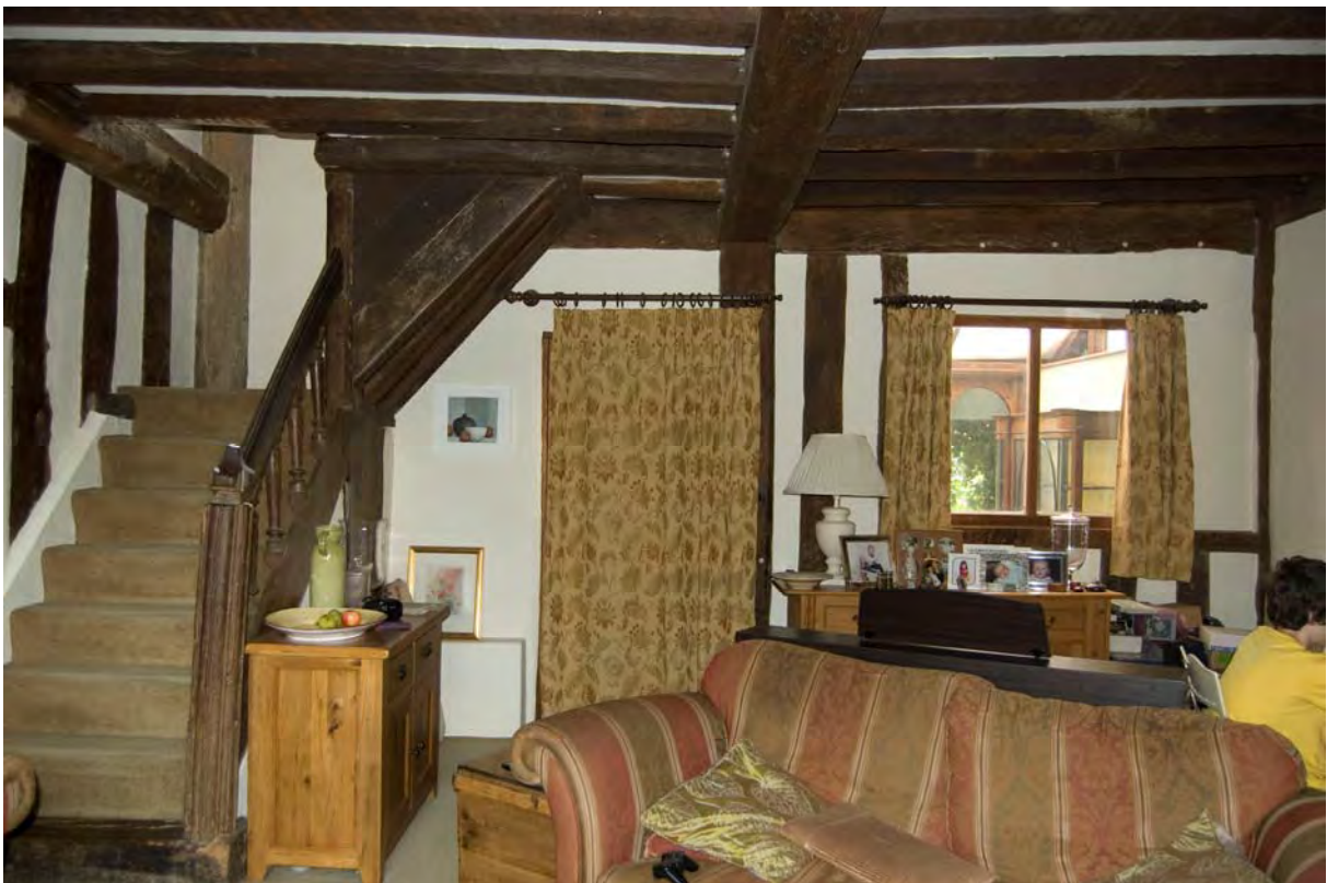
Fig 19: Close studding and inserted stair
