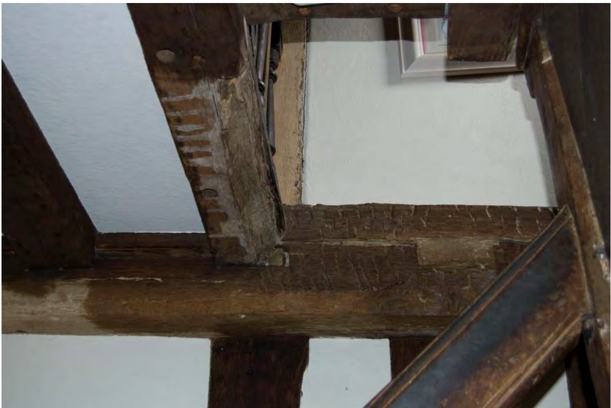
Fig 21: Chamfered side of beam
