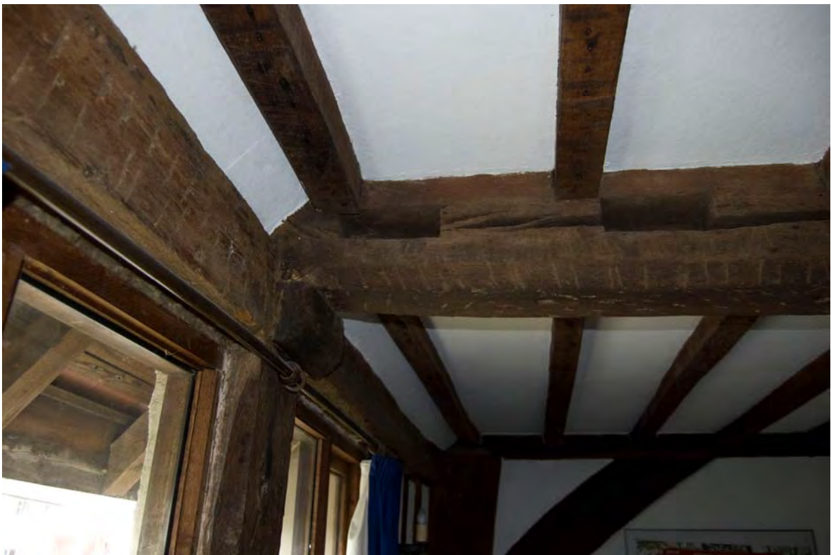
Fig 35: Detail of timberwork
