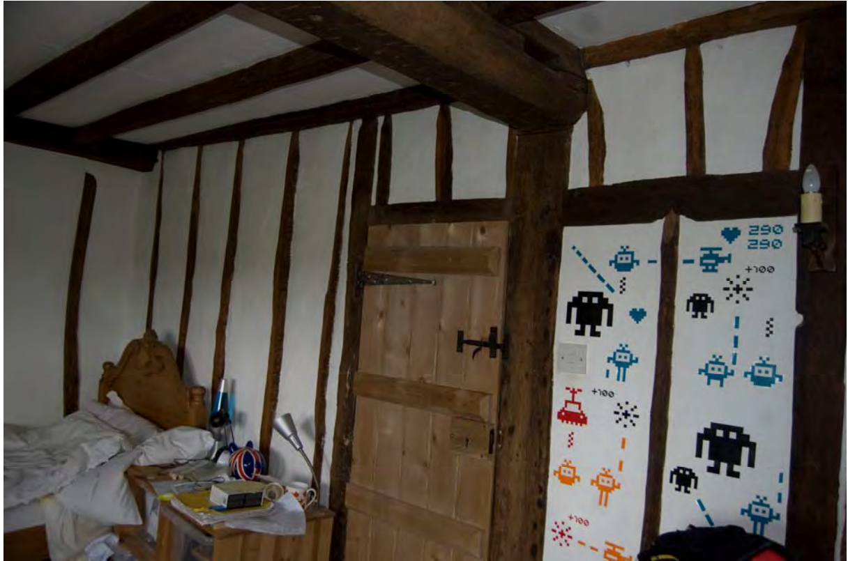
Fig 36: Staves in dividing wall
