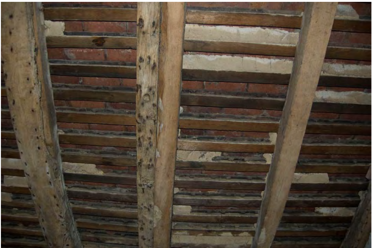
Fig 49: Old and new rafters
