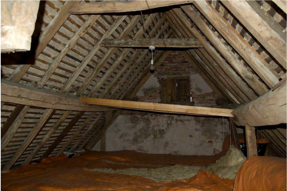
Fig 46: Eastern side of roofspace
