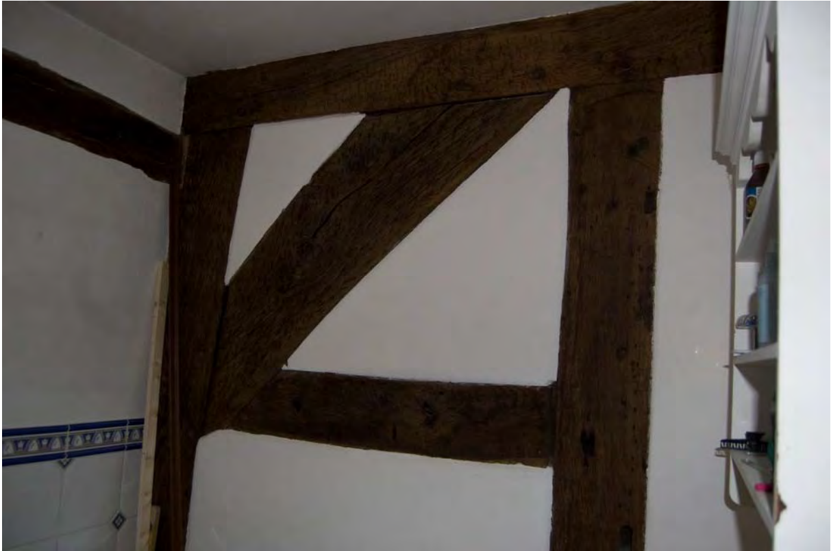
Fig 40: Timber-framing in bathroom
