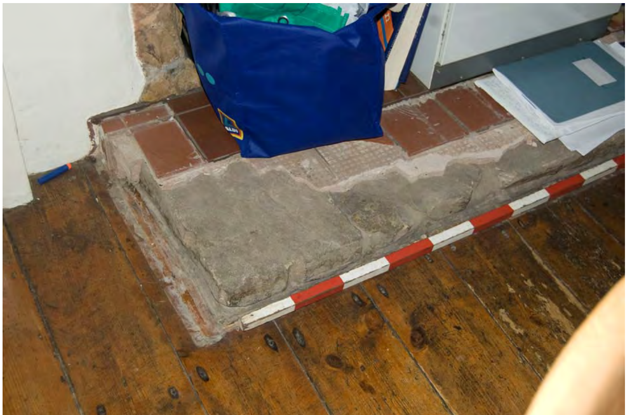
Fig 15: Stone hearth beneath quarry tiles
