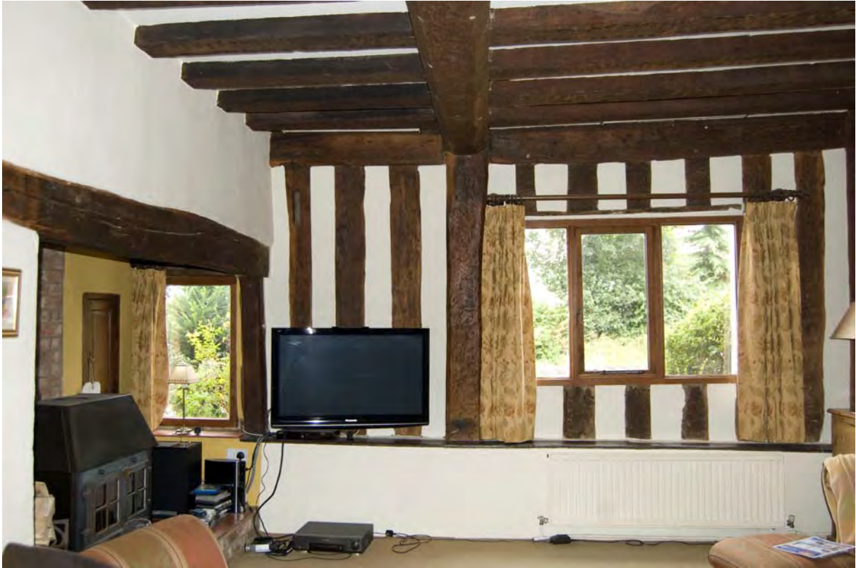
Fig 18: Close studding on interior wall
