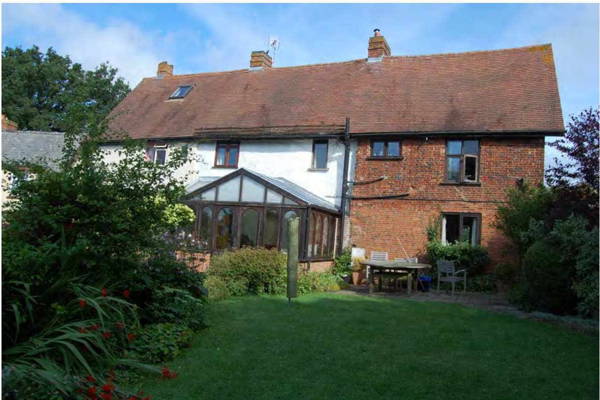
Fig 5: Rear of house
