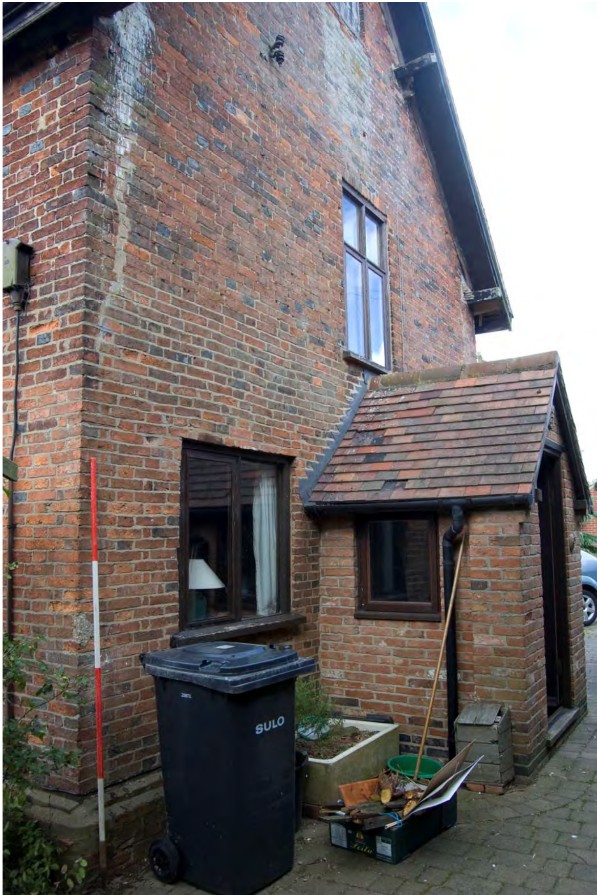
Fig 6: Gable end of house with modern porch
