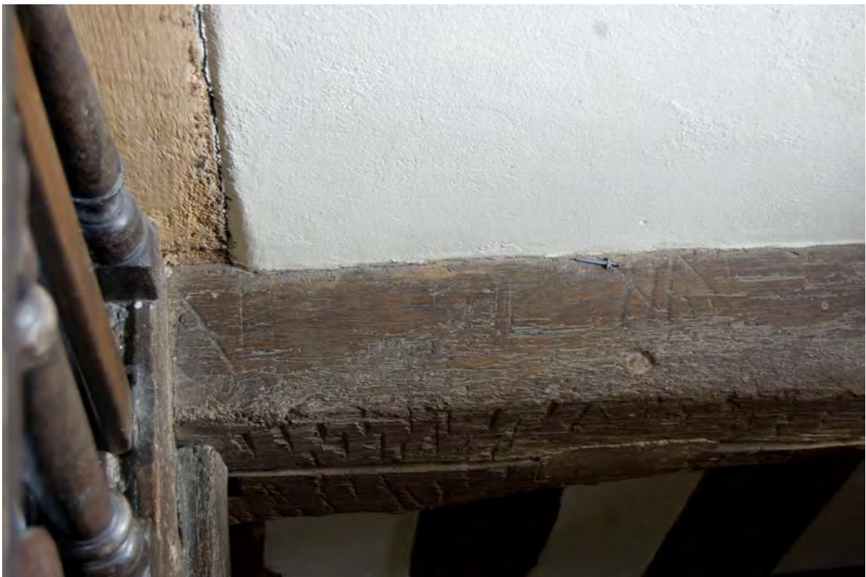
Fig 39: Carpenter's marks
