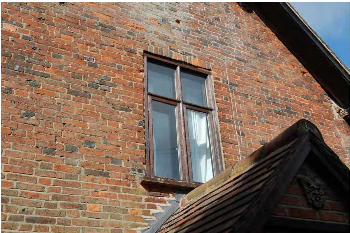
Fig 8: Window in former doorway in gable end
