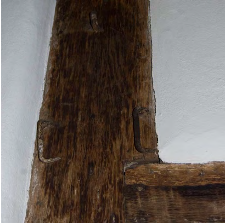
Fig 22: Hooks on beam
