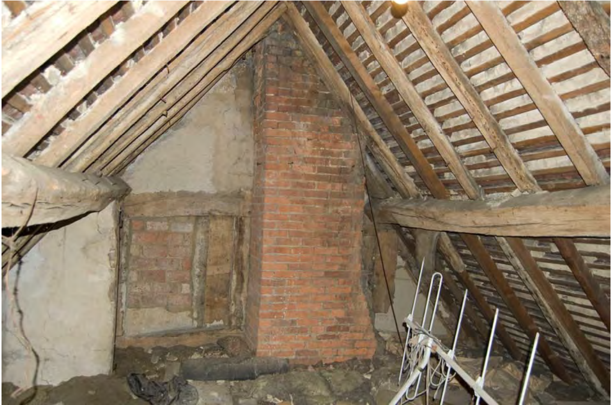
Fig 42: Attic, brick chimney
