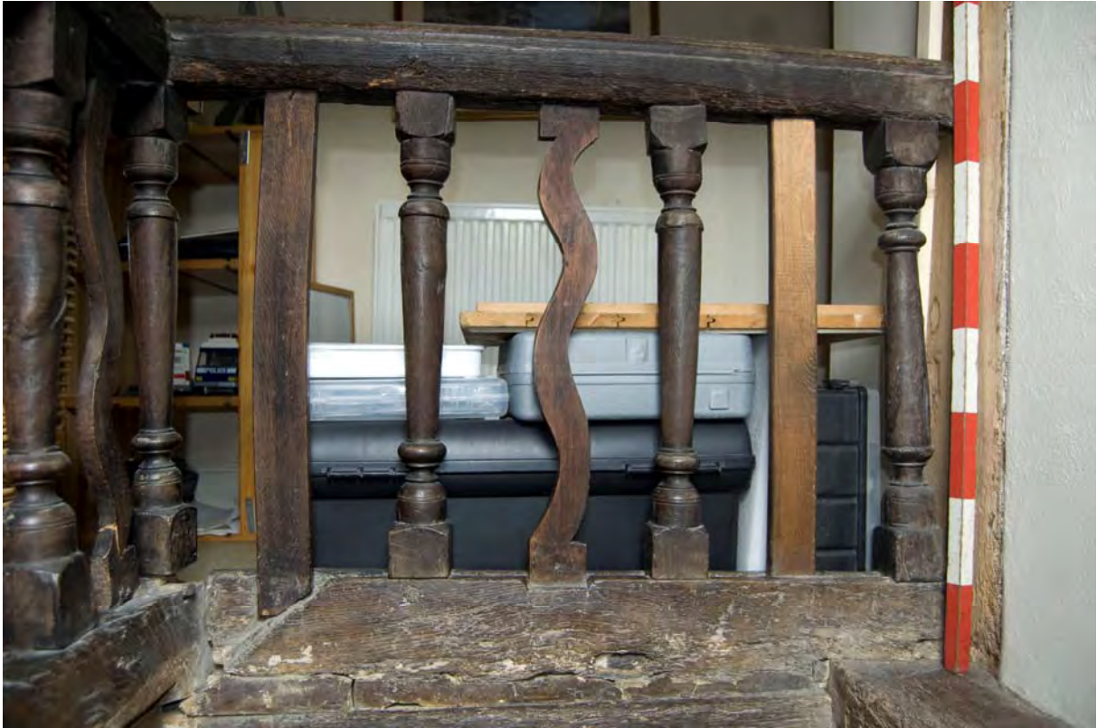
Fig 38: Staircase balusters
