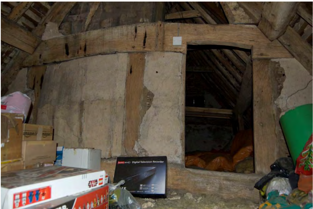
Fig 43: Attic, central partition
