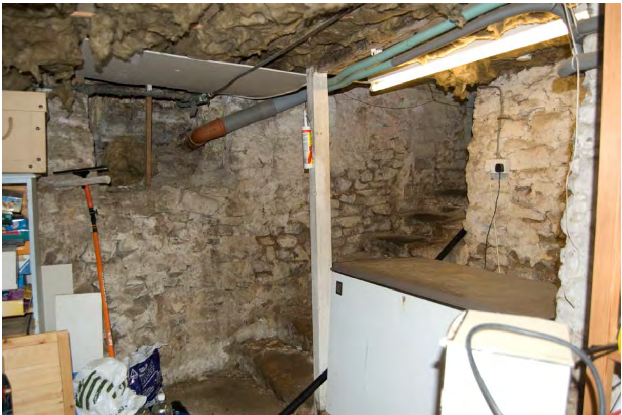
Fig 29: Cellar, looking south
