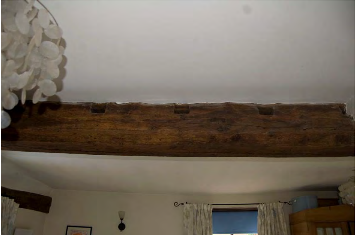
Fig 32: Timber with joist holes
