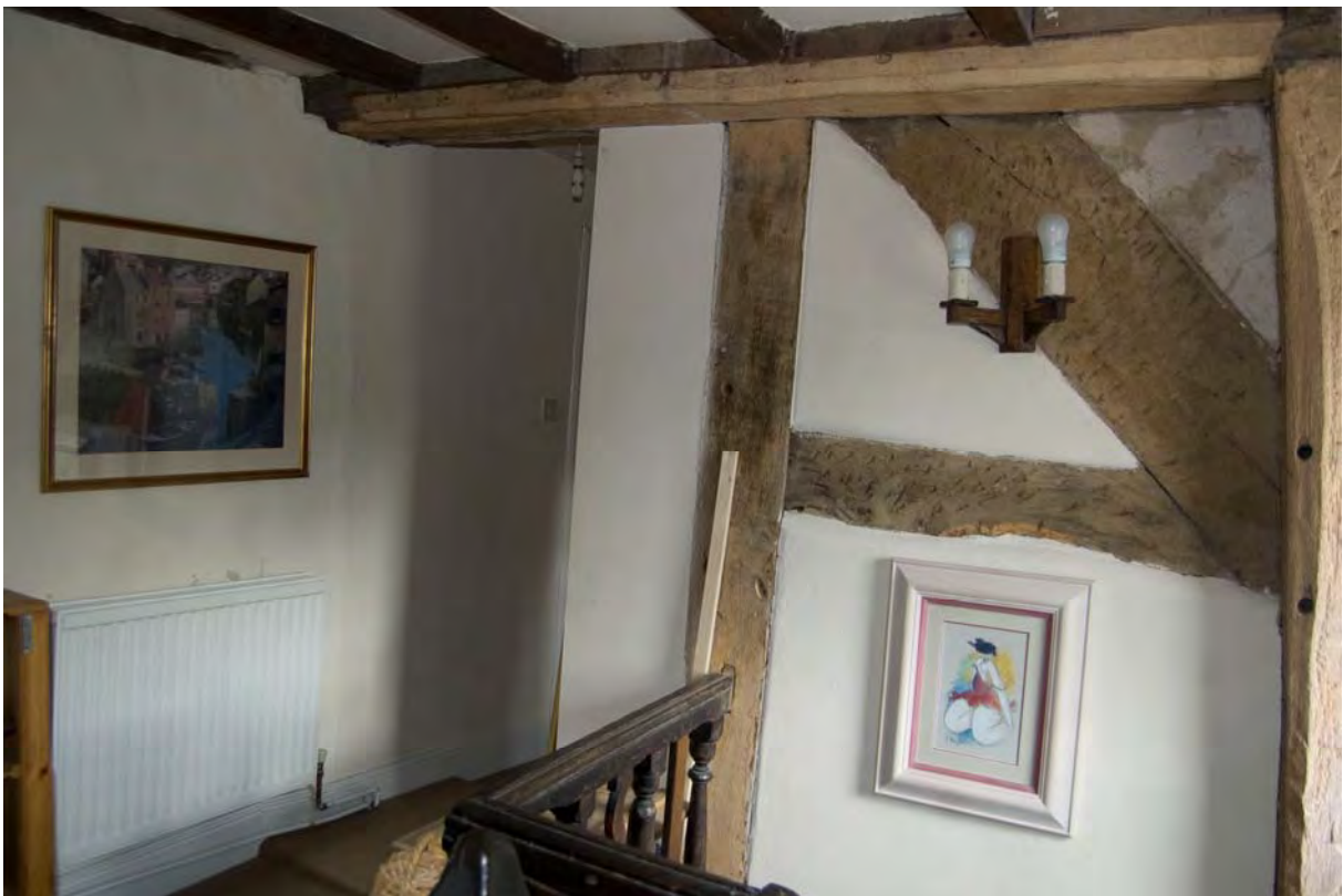
Fig 41: Timber-framing in hall
