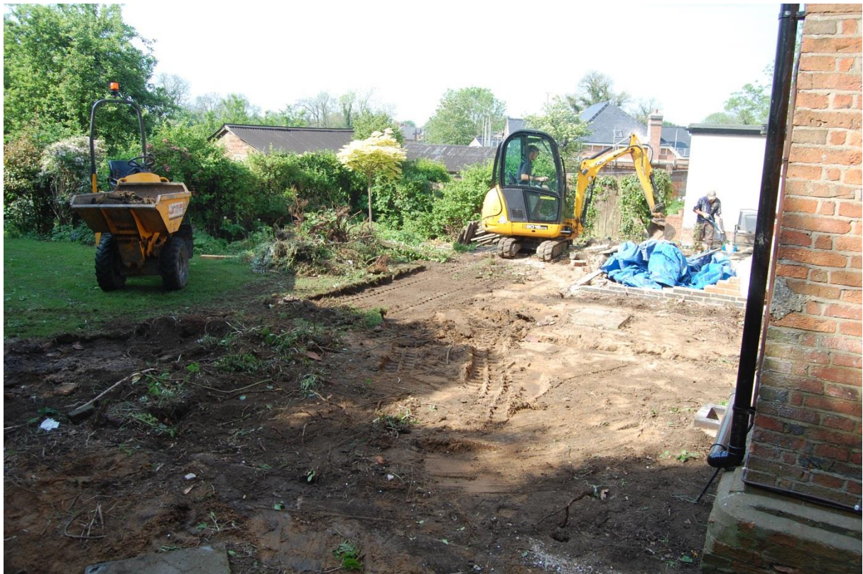
Fig 4: Rear of the house, prior to trench excavation
