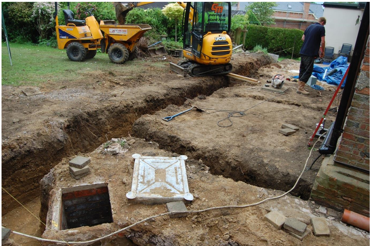
Fig 6: Trenches excavated for extension
