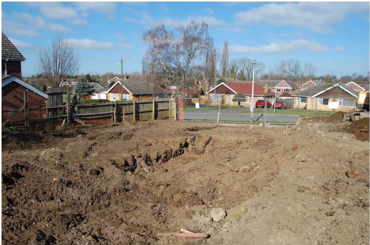
2 Site stripping, looking towards Constable Road
