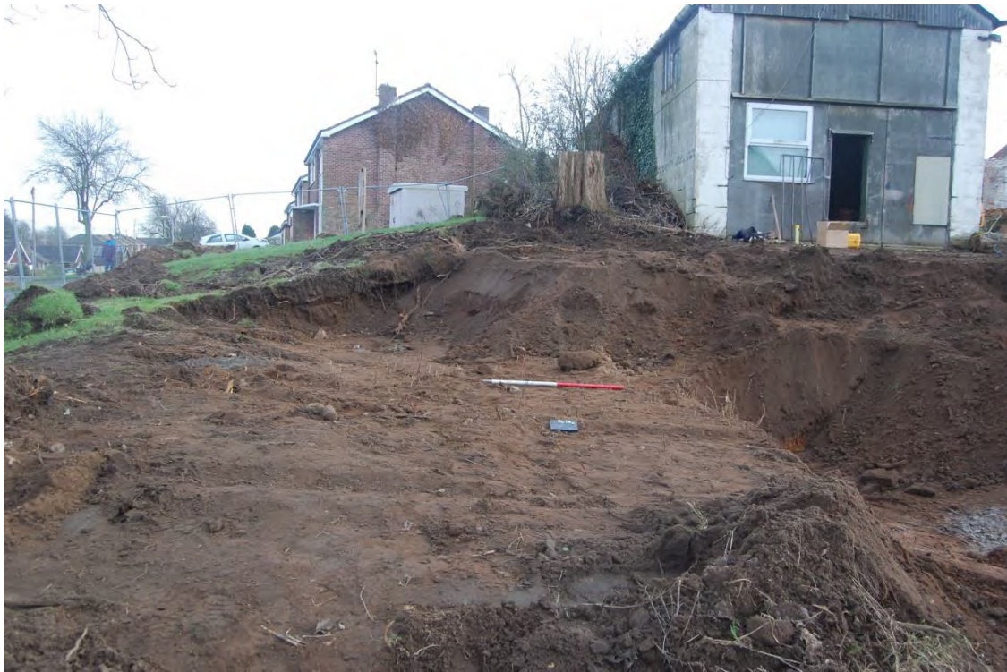
1 Site being stripped, looking east
