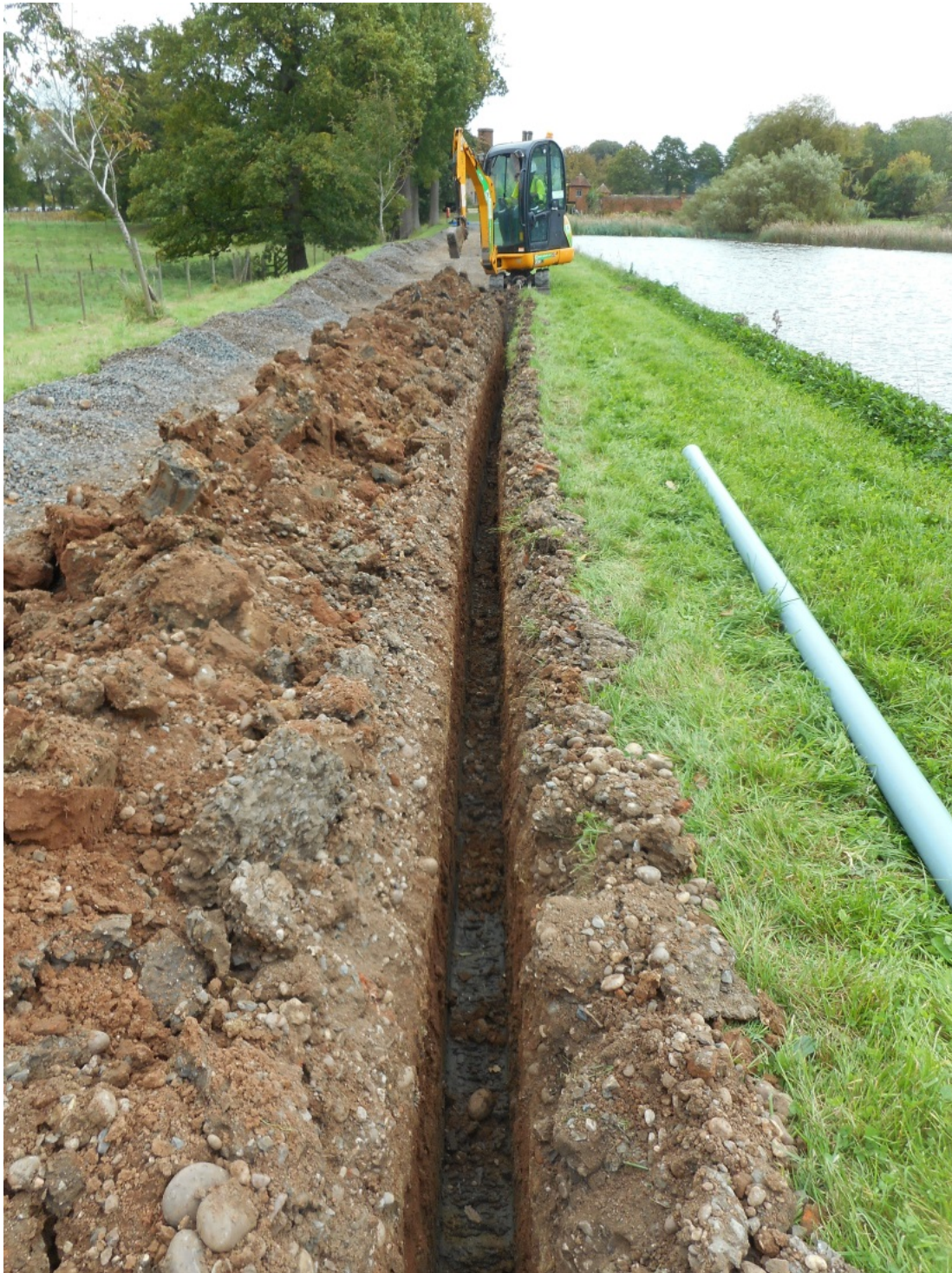
1. View of service trench alongside lake, looking north-east towards Packwood House
