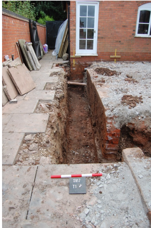
1. Foundation trench 1 facing south-east
