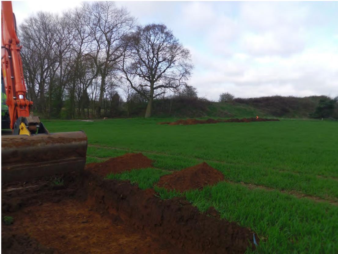
1: General view of site during excavation, looking NW
