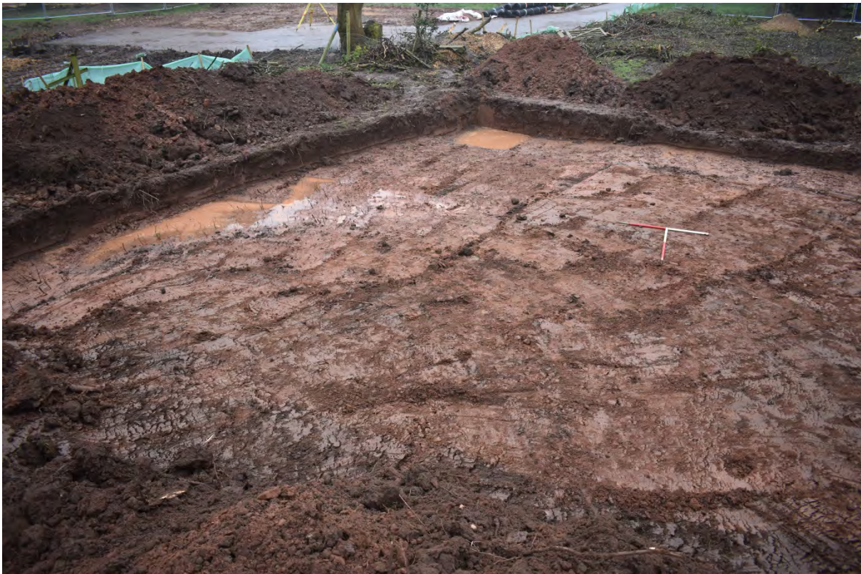
Photograph 2: SE corner of the site during stripping looking SE
