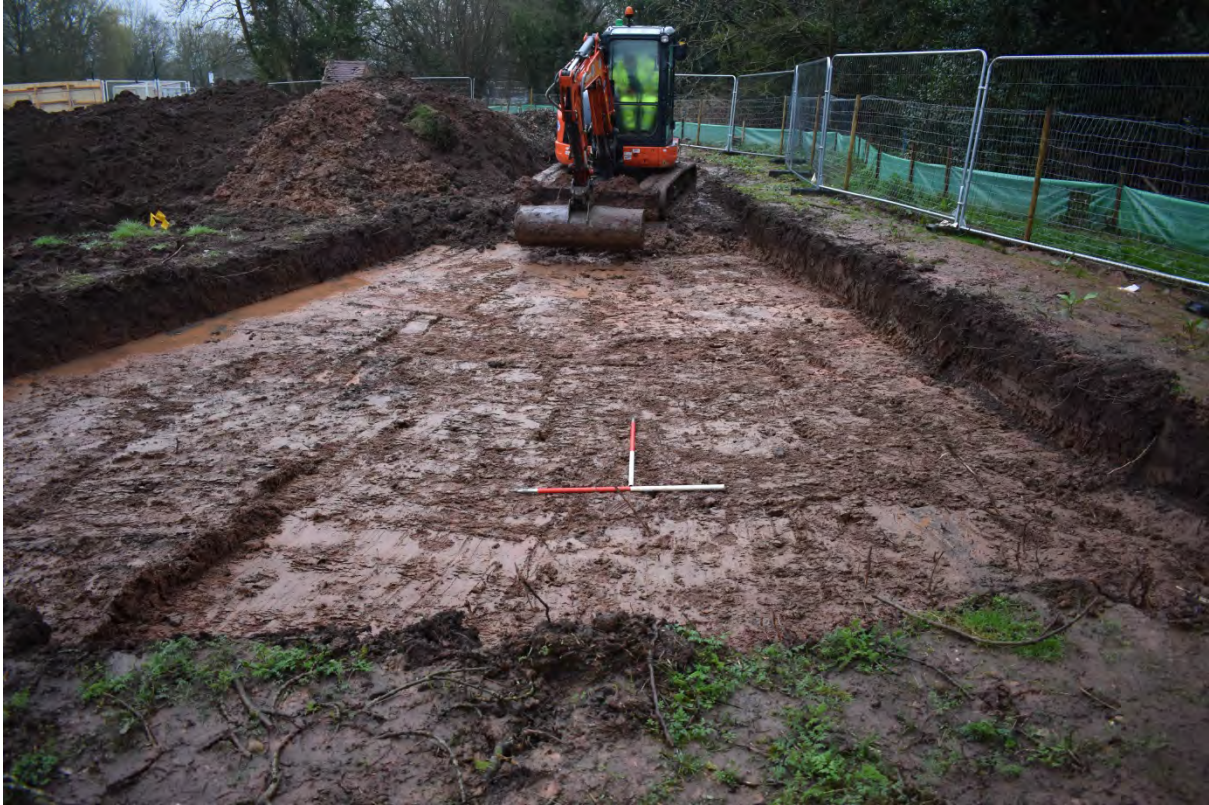
Photograph 1: NW corner of the site during stripping looking S
