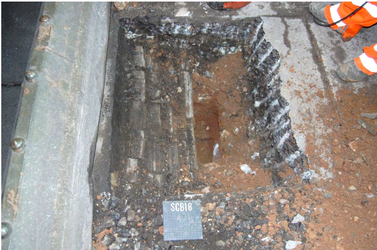
2. Original footings, tie iron and pipe
