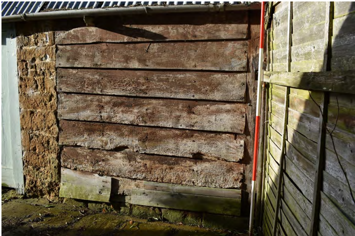
4: Detail of weather-boarding
