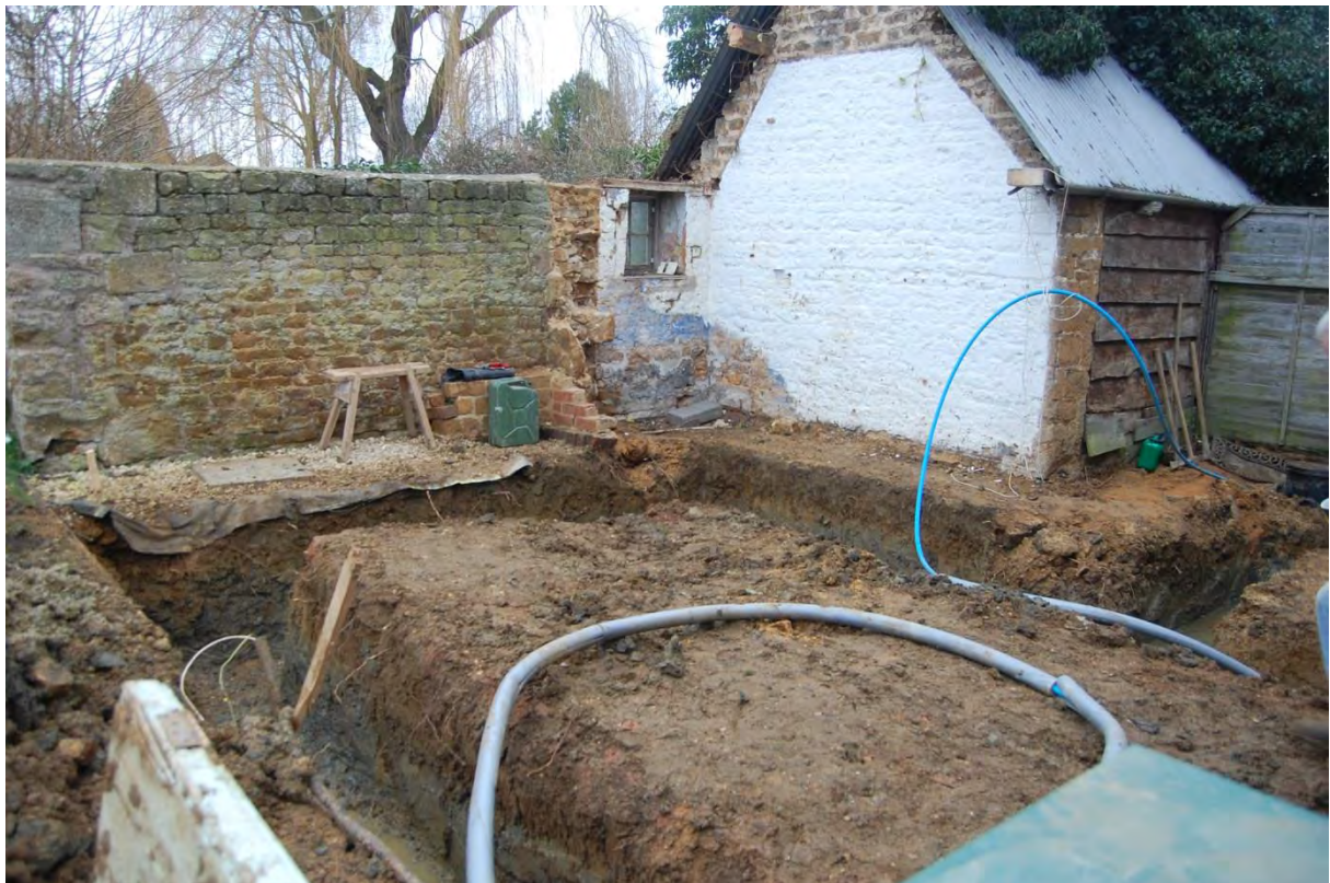
12: New foundation trenches excavated
