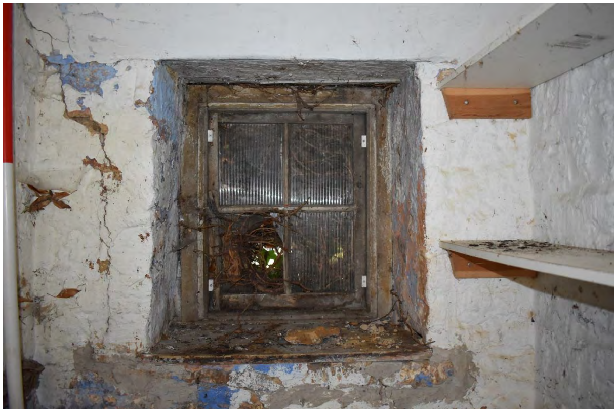
9: Window set into rear wall
