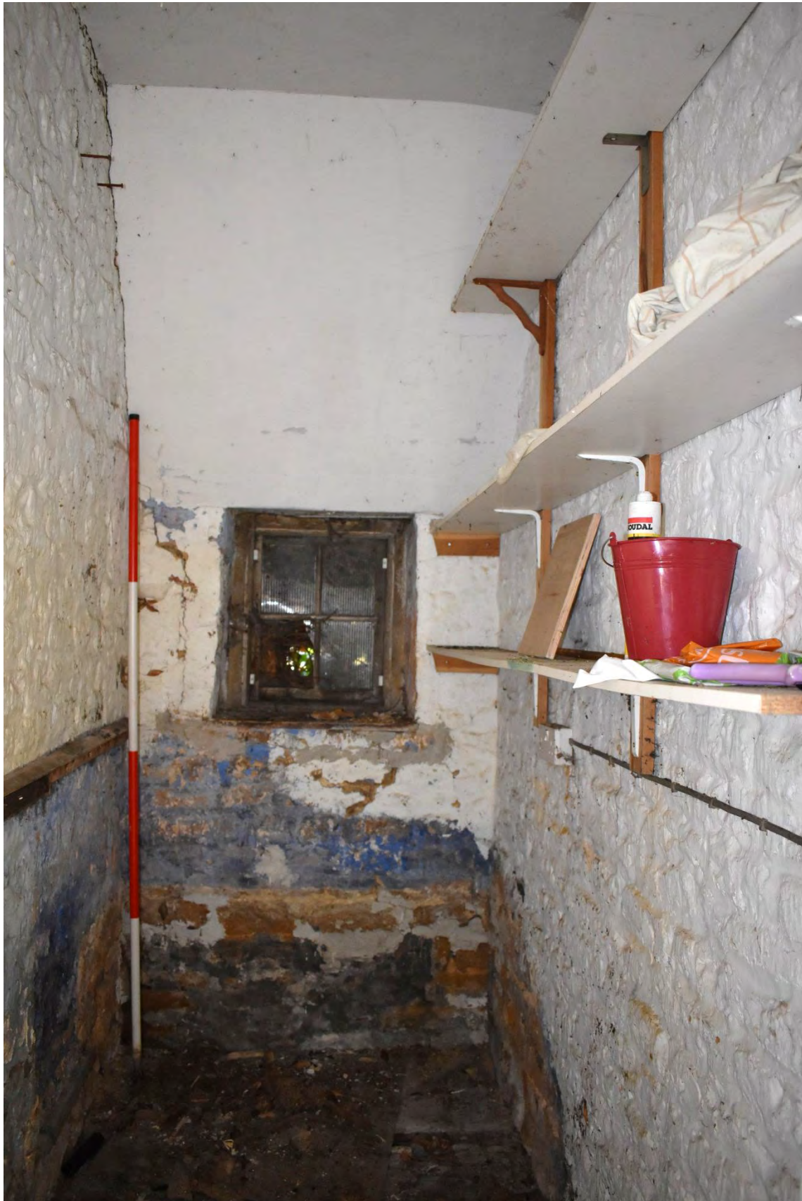
10: Interior of south-west part of outbuilding
