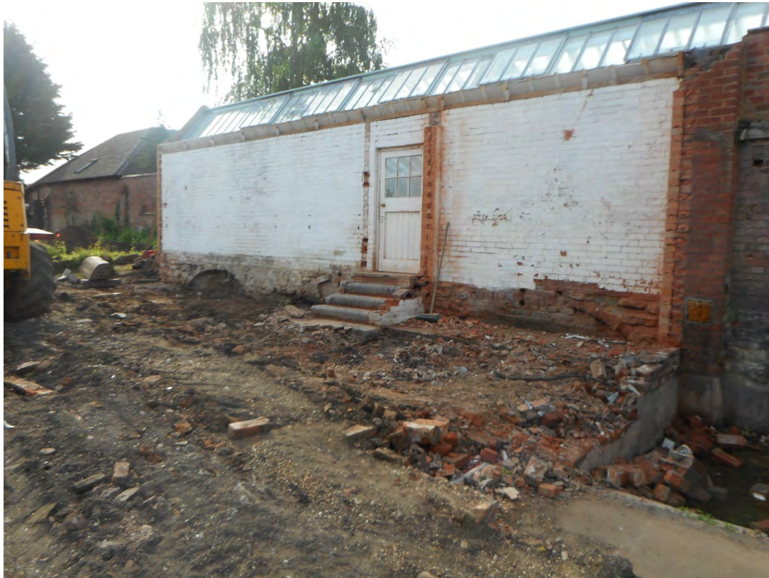
5: Arches in the foundations of glasshouse on southern boundary
