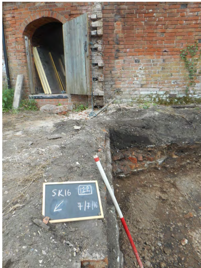
4: Demolished wall 122, looking south
