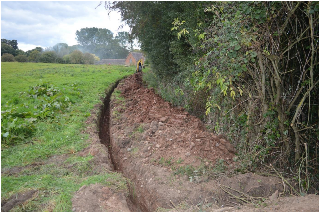
1. Excavation of trench in main field
