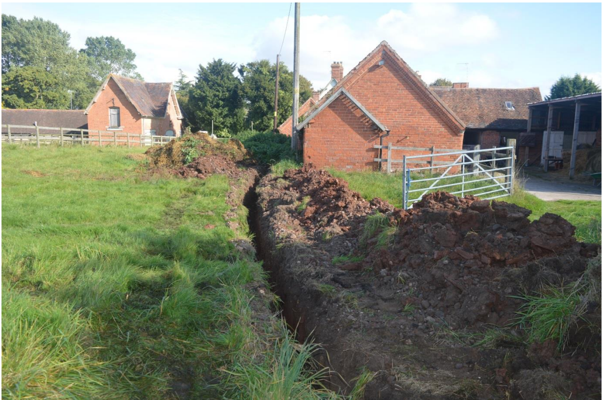
2. Trench excavated adjacent to farm buildings
