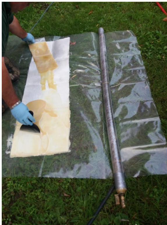
3: Preparation of patch-liner material
