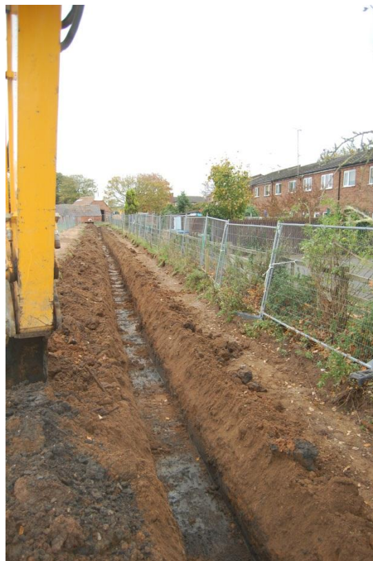
Fig 2: View along excavated trench
