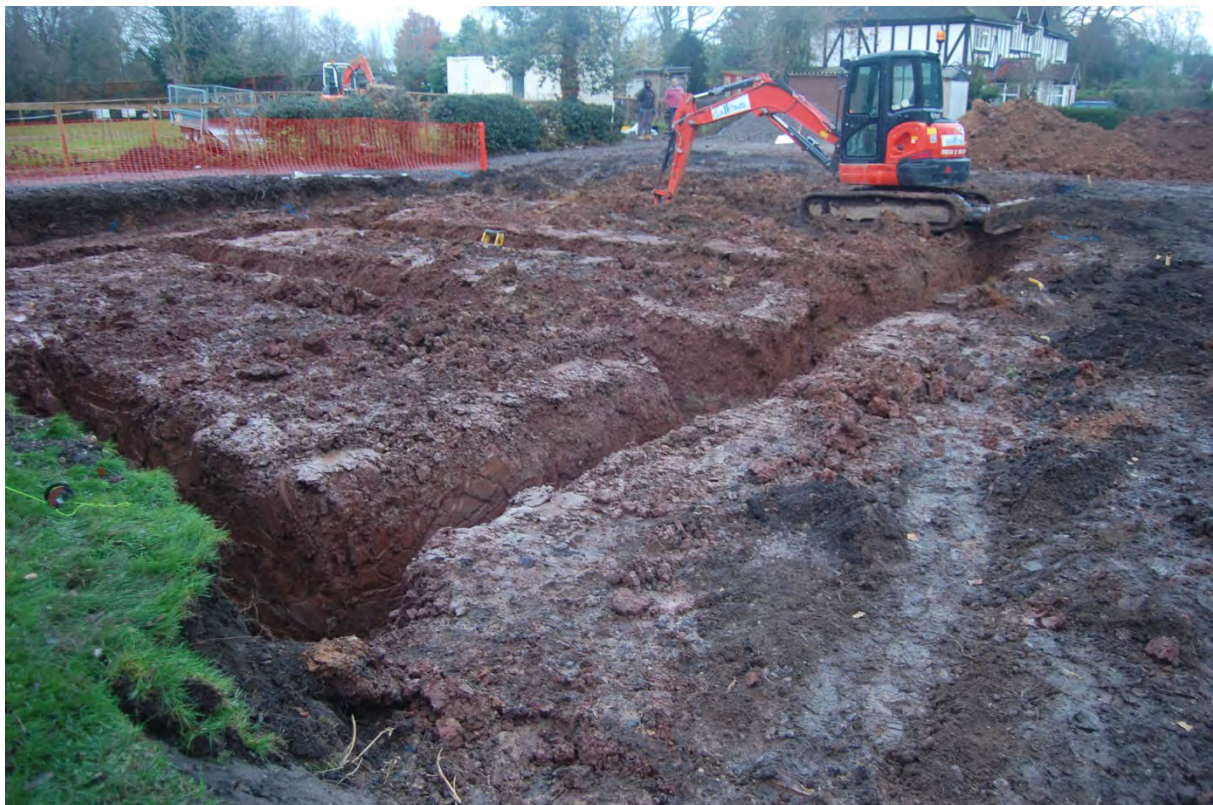
4: General site shot following excavation of observed foundation trenches, looking north-east
