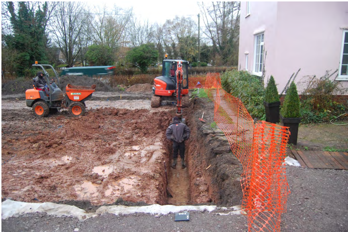
1: Foundation trenches under excavation, looking south
