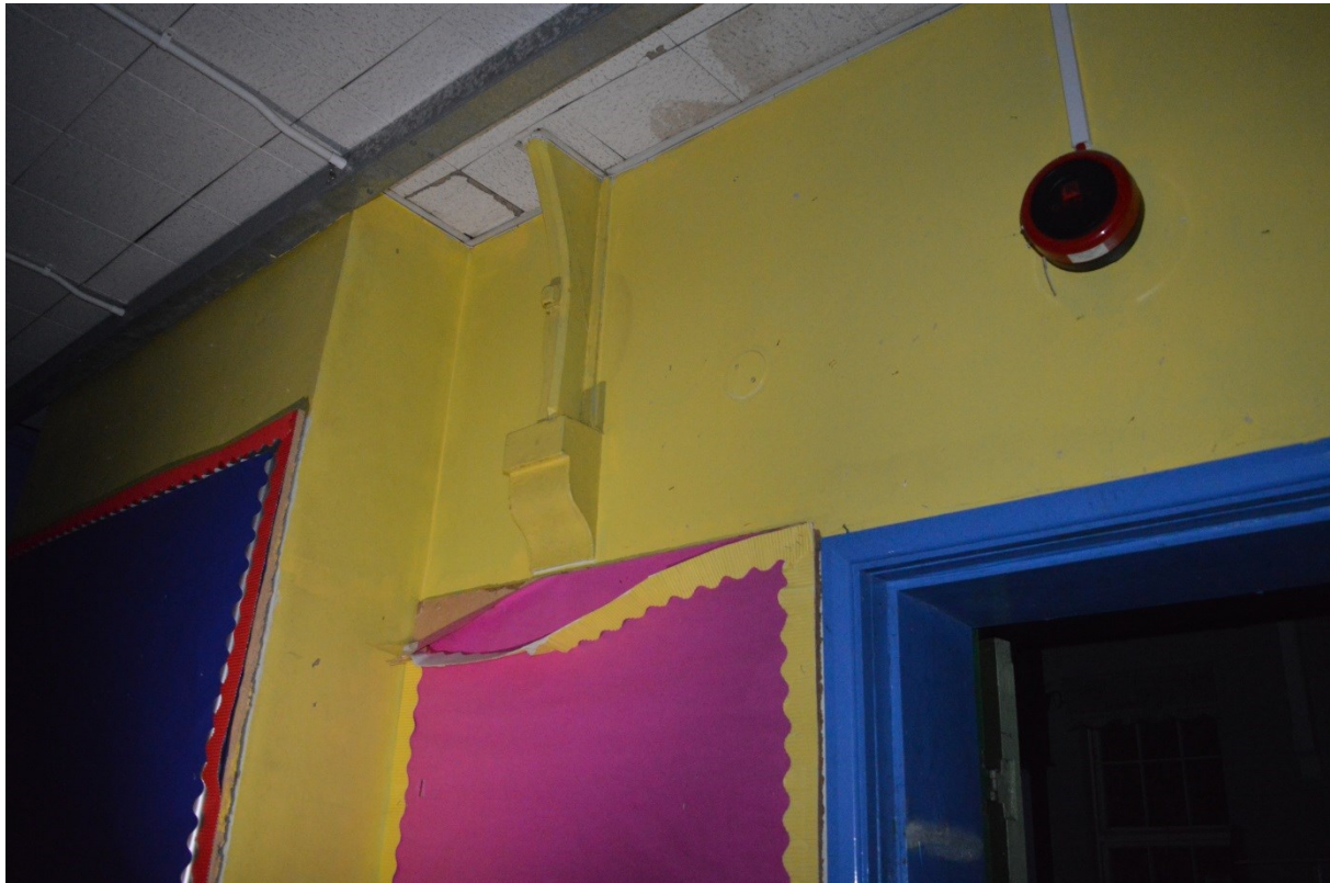
Photograph 18: Classroom A corbel detail
