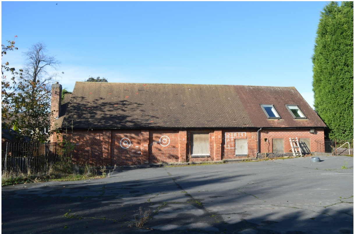
Photograph 7: Rear of school
