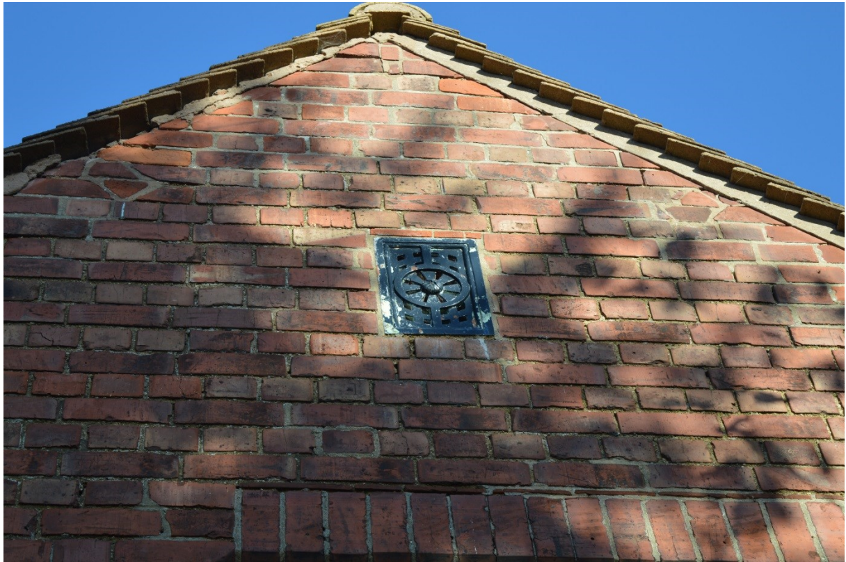
Photograph 6: SW elevation vent detail
