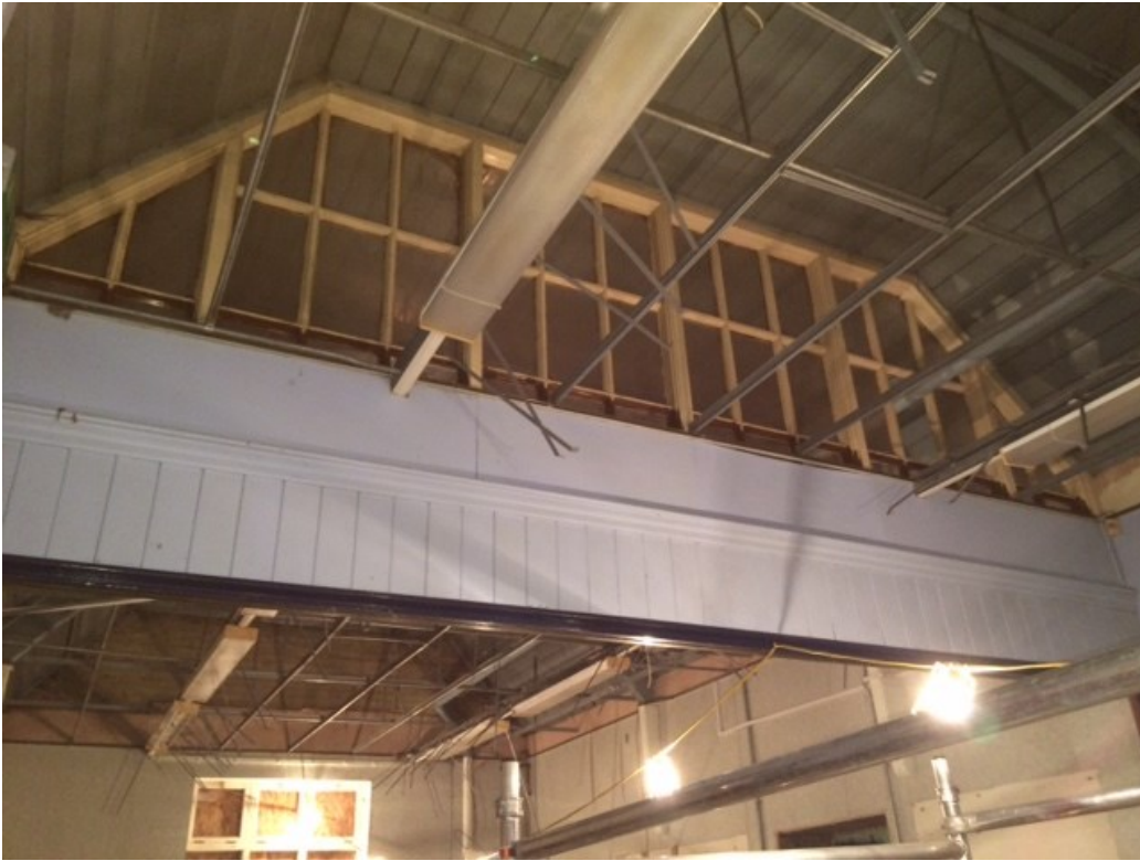
Photograph 16: Classroom B roof detail
