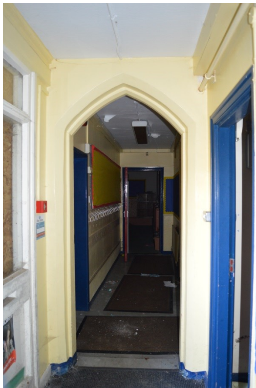
Photograph 9: Door to school, now within modern extension
