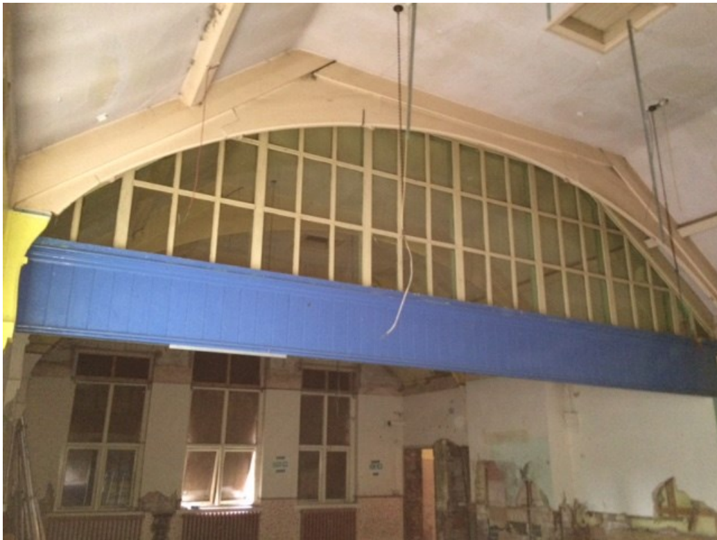
Photograph 12: Classroom A roof detail
