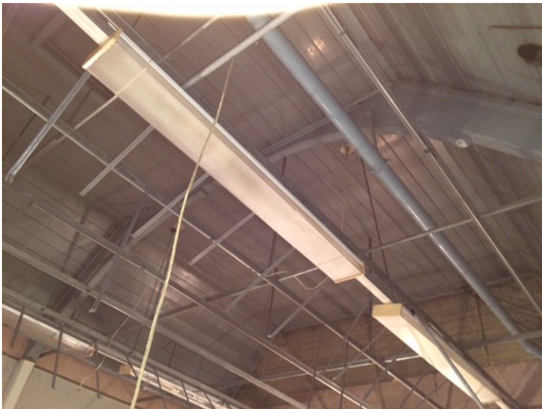
Photograph 17: Classroom B roof detail
