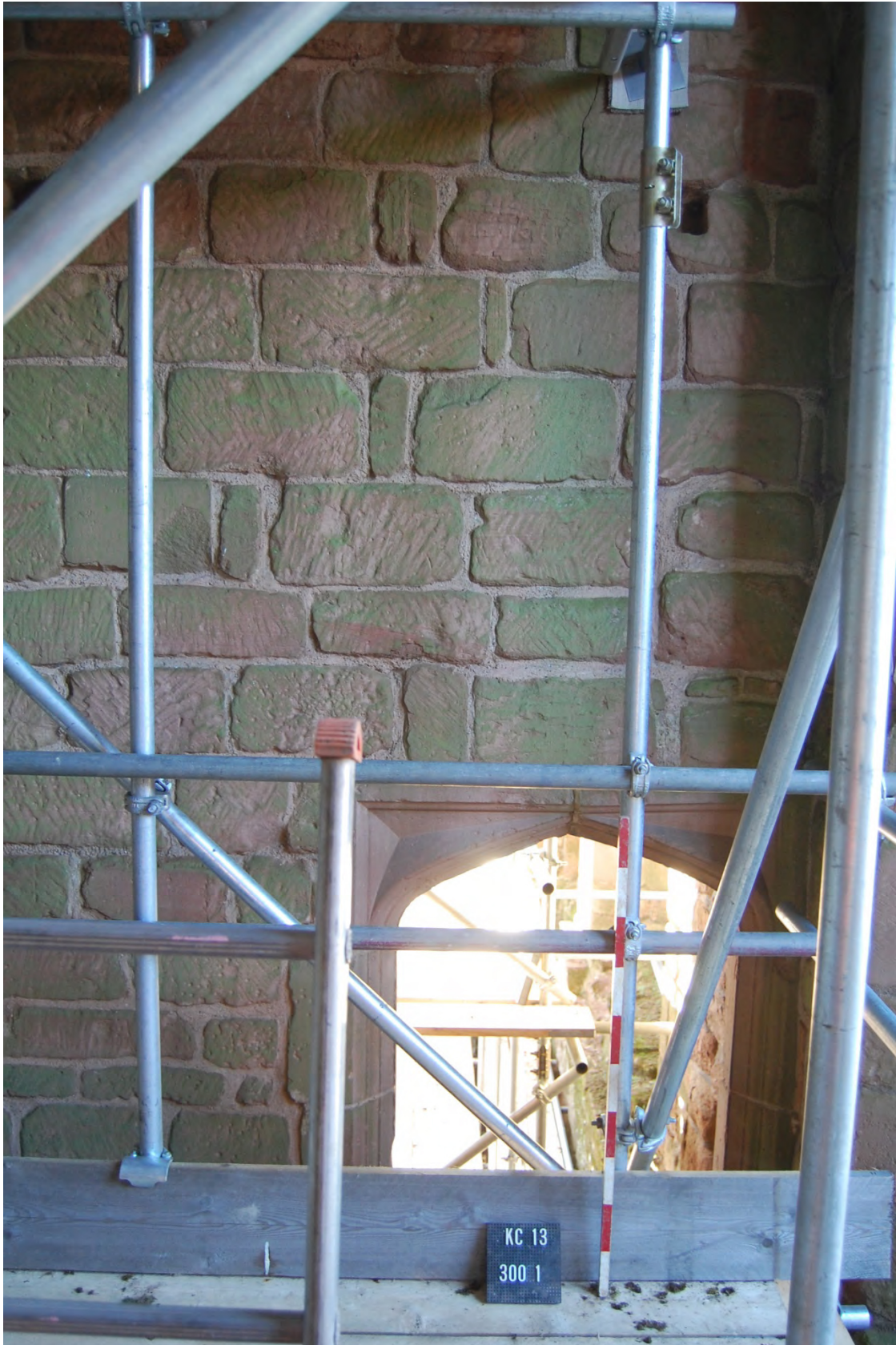
28 NW room, ground floor, masonry above doorway (Drawing 27, Sheet 8/1)
