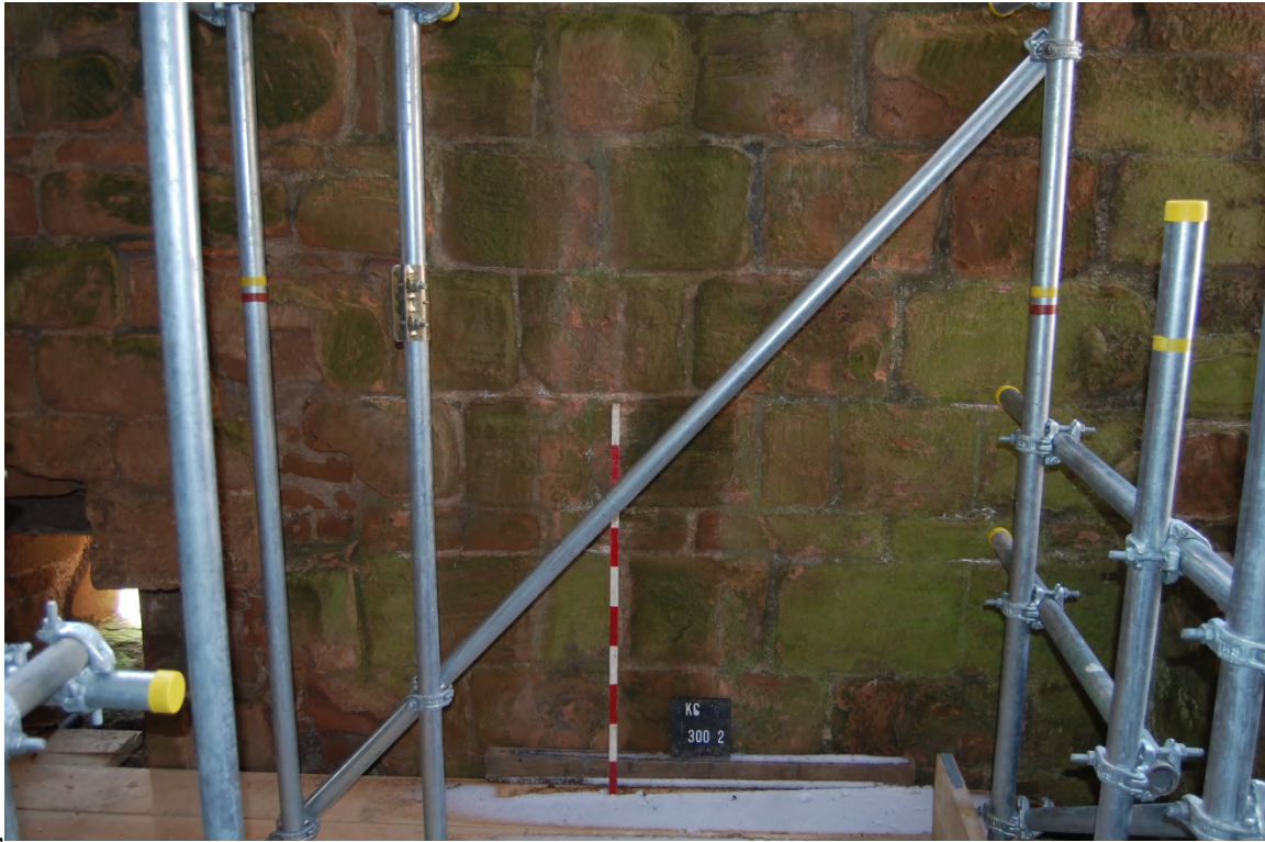
9 NW room, ground floor, masonry (Drawing 7, Sheet 1/7)
