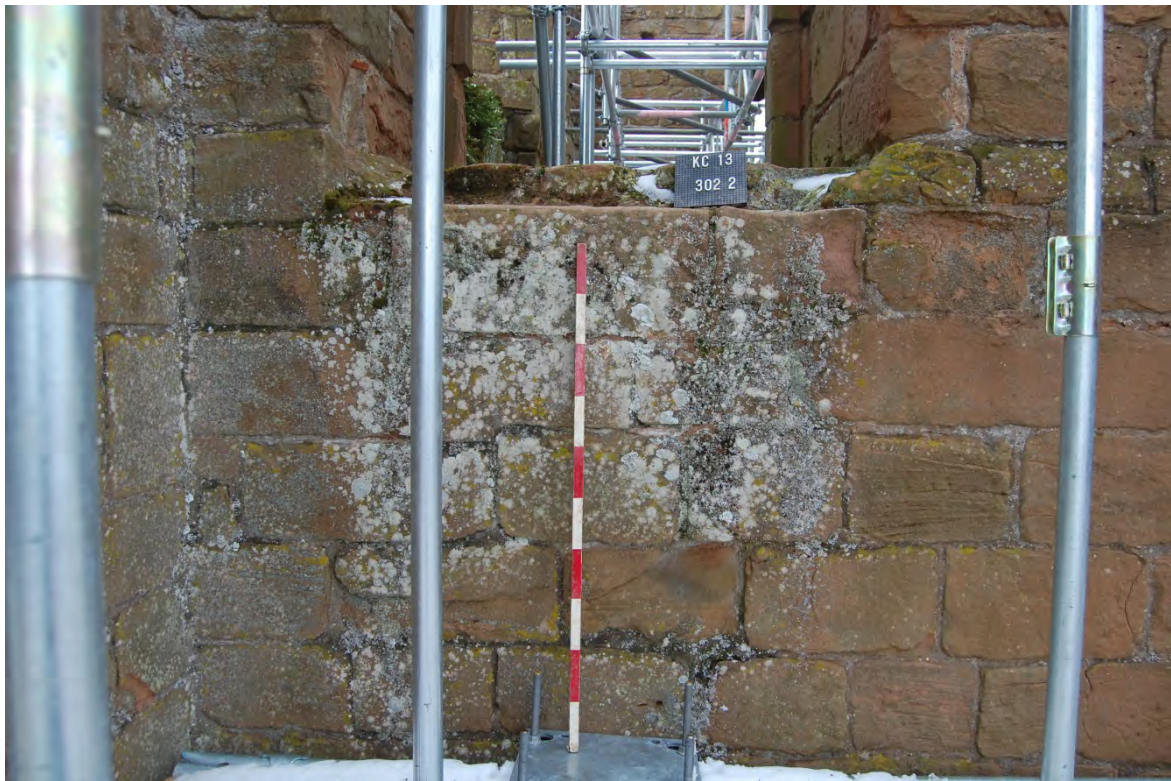
19 S room, top floor, masonry below doorway (Drawing 18, Sheet 5/3)
