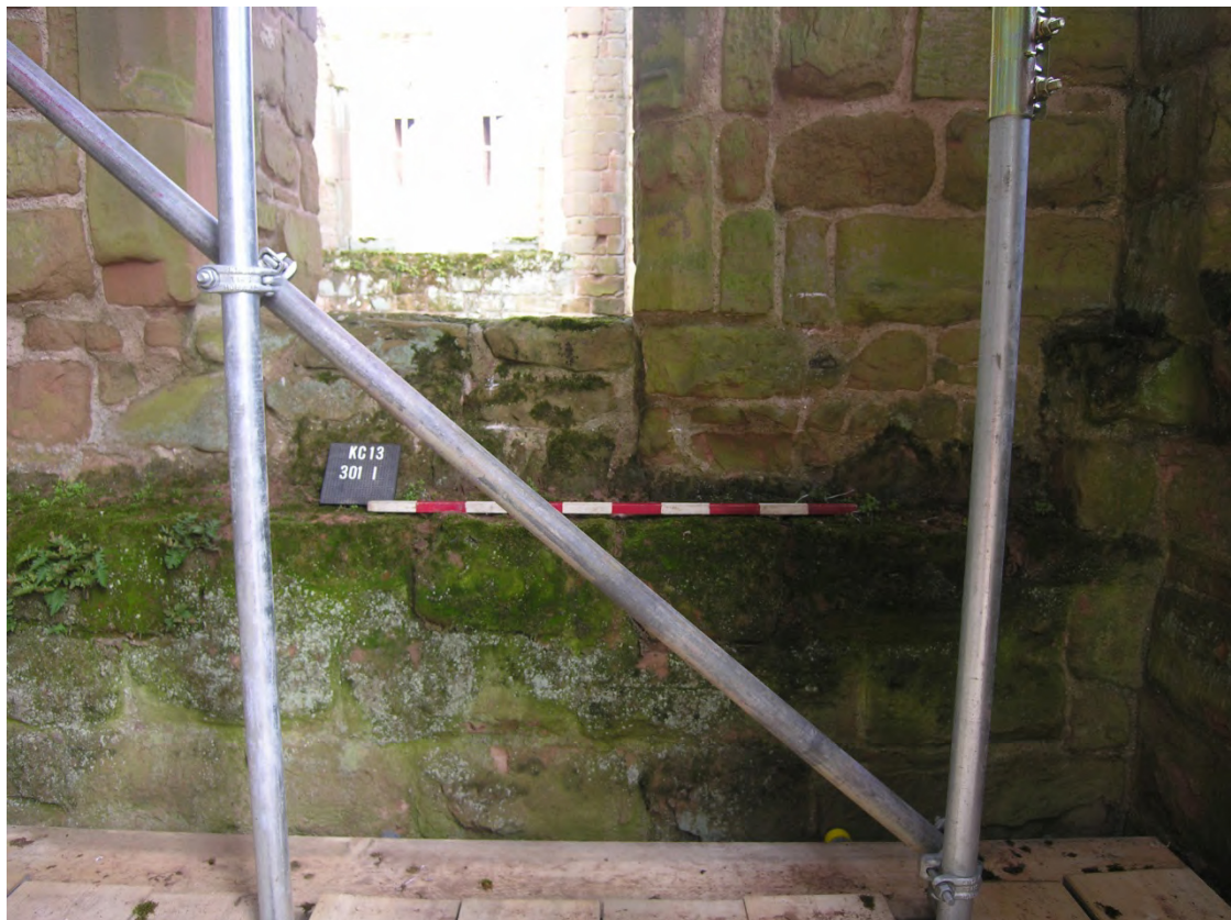
6 NE room, principal floor, masonry below doorway (Drawing 4, Sheet 1/4)
