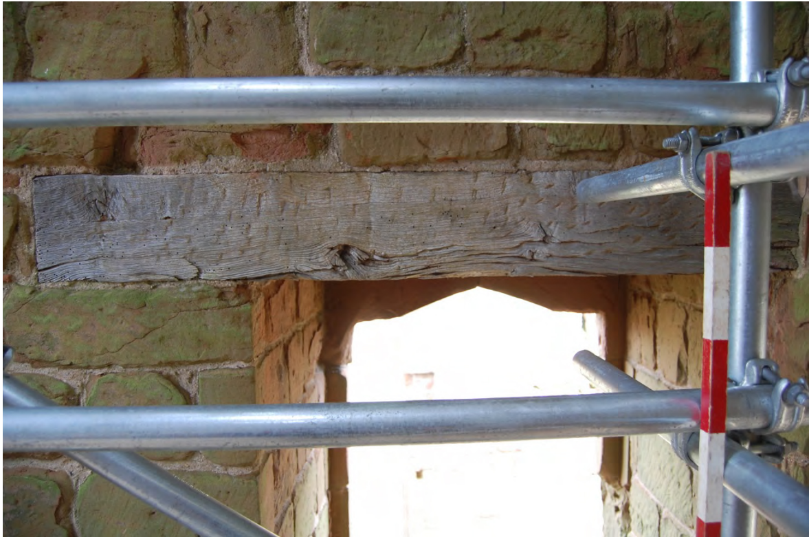
29 NW room, principal floor, lintel (Drawing 29, Sheet 8/3), HE samples 6, 21, 22
