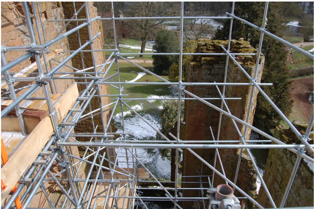
2 View of scaffolding within Leicester's Building
