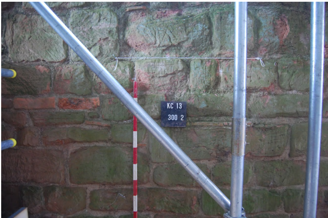
40 NW room, ground floor, masonry (Drawing 41, Sheet 12/2)
