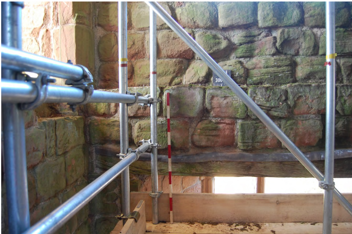
26 NW room, ground floor, lintel and masonry (Drawing 25, Sheet 7/3)
