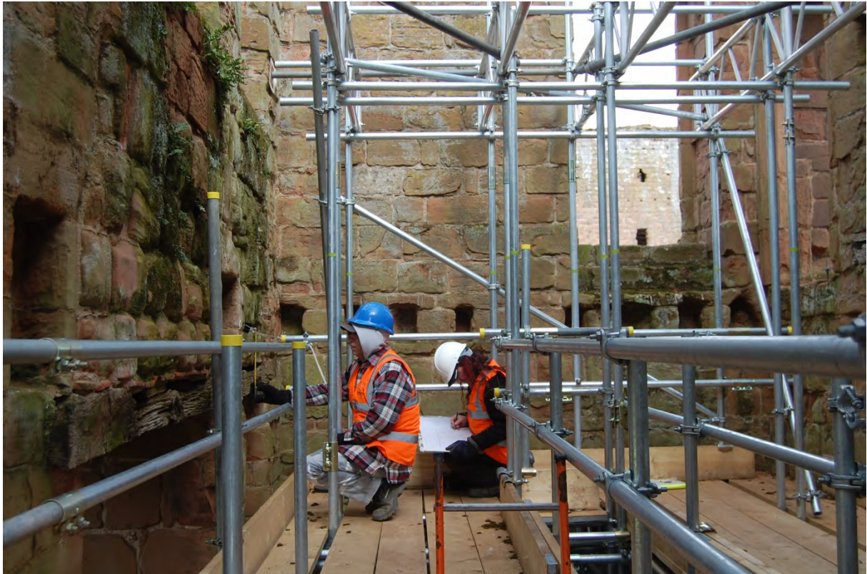
1 Carrying out recording in the NW room
