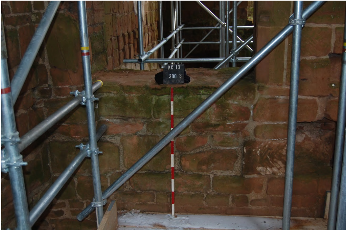
11 NW room, ground floor, masonry below doorway (Drawing 9, Sheet 2/1)
