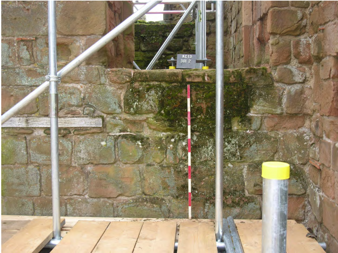
7 NE room, top floor, masonry below doorway (Drawing 5, Sheet 1/5)
