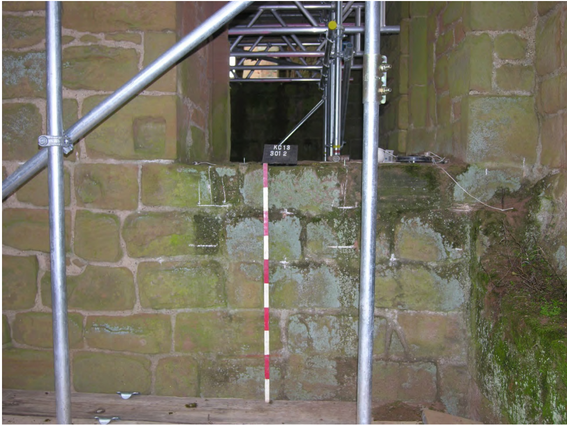
5 NE room, principal floor, masonry below doorway (Drawing 3, Sheet 1/3)
