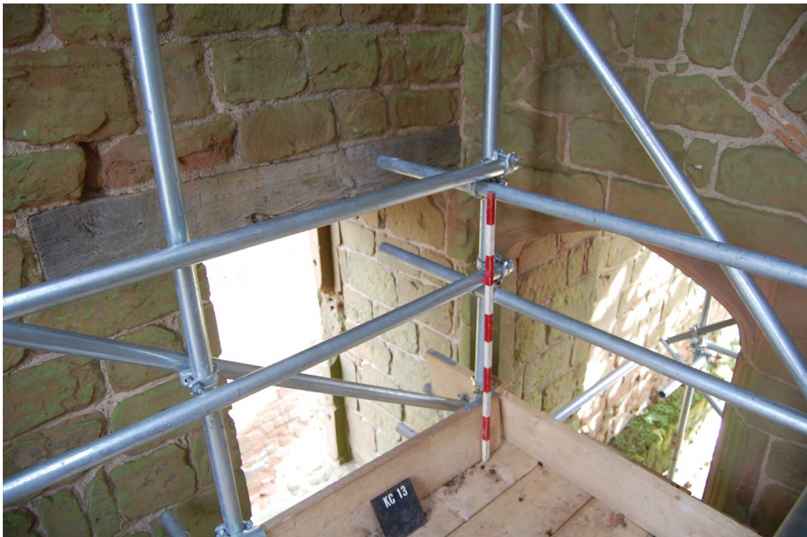
30 NW room, relieving arch over doorway (Drawings 29 and 30, Sheets 8/3 and 8/4)
