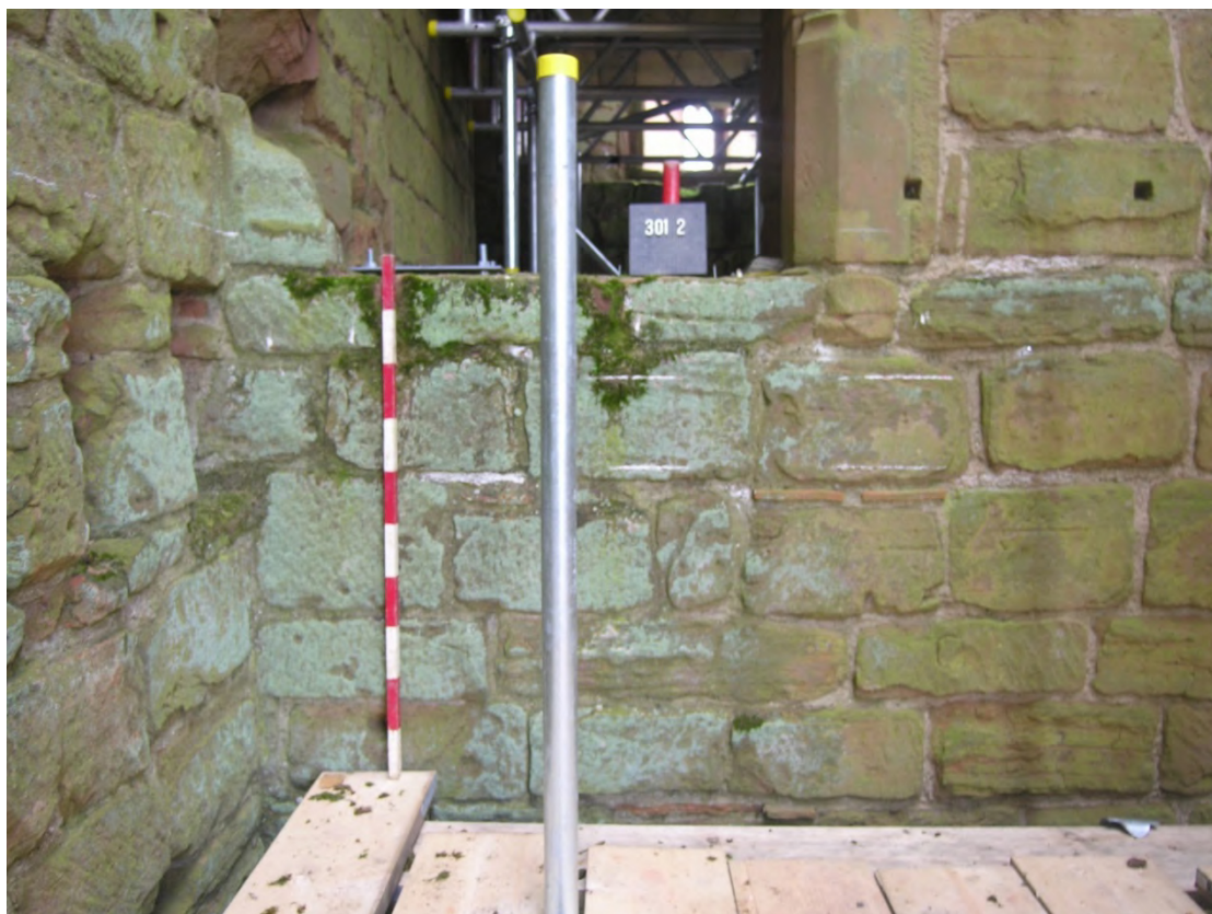
4 NE room, principal floor, masonry below doorway (Drawing 2, Sheet 1/2)
