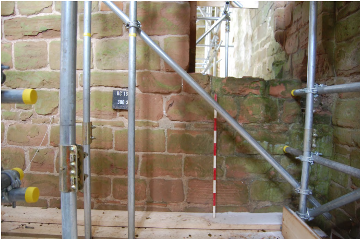
12 NW room, ground floor, masonry below doorway (Drawing 10, Sheet 2/2)
