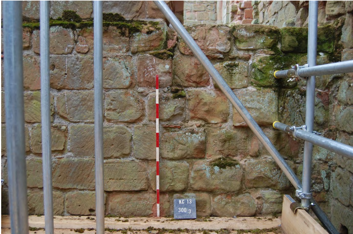
31 NW room, top floor, masonry below doorway (Drawing 31, Sheet 9/1)
