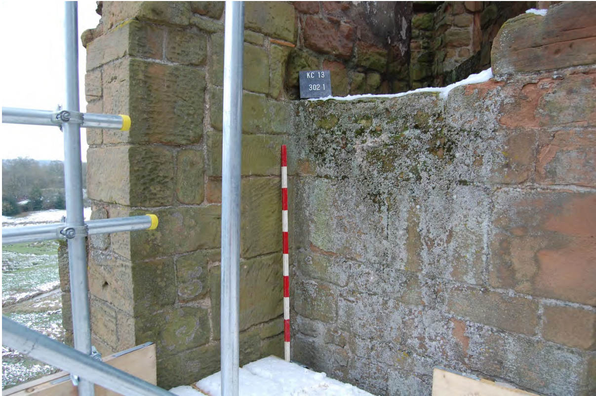
18 S room, top floor, masonry (Drawings 16 (L) and 17(R). Sheets 5/1 and 5/2)
