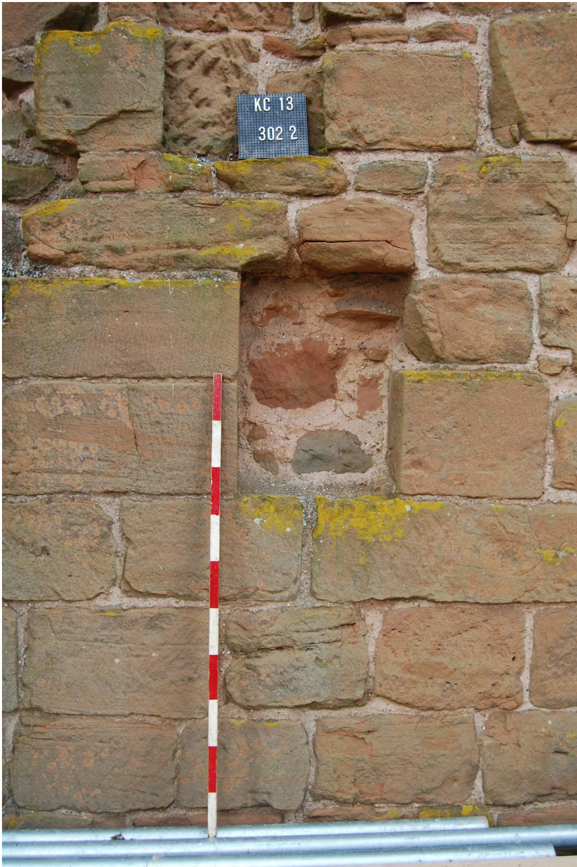
22 S room, principal floor, masonry by fireplace (Drawing 21, Sheet 6/3)
