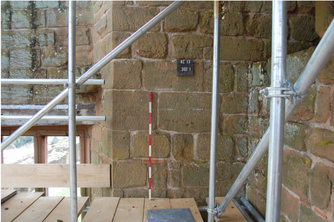
20 S room, principal floor, masonry by window (Drawing 19, Sheet 6/1)
