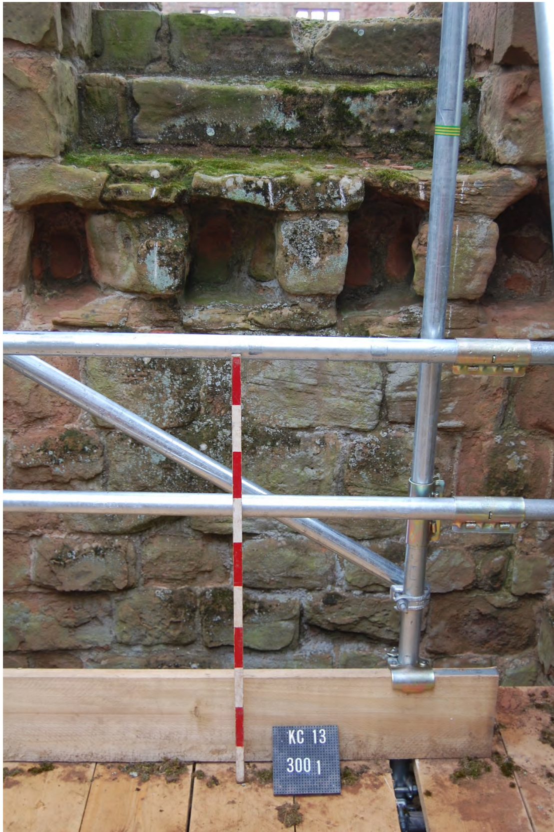
33 NW room, top floor, joist holes (Drawing 33, Sheet 9/3)
