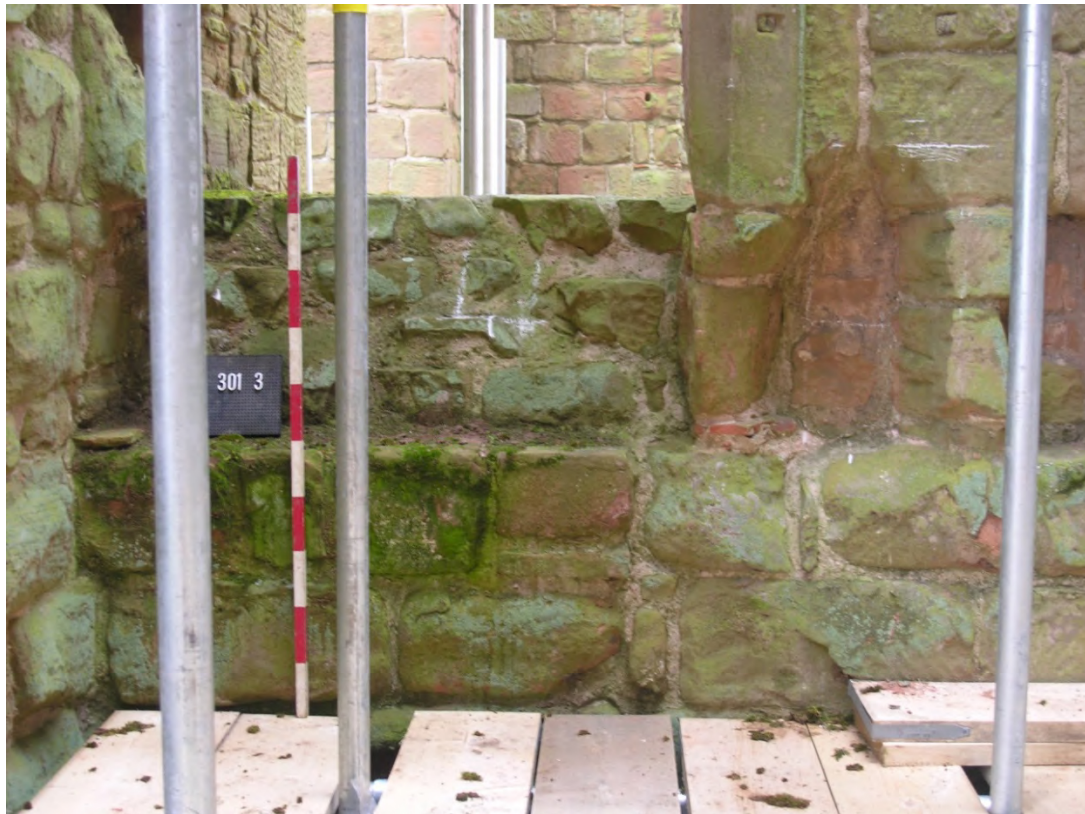
3 NE room, top floor, masonry below doorway (Drawing 1, Sheet 1/1)
