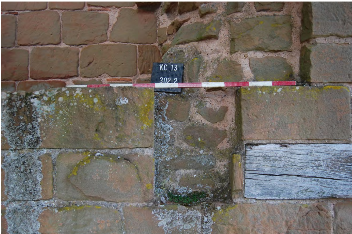
21 S room, principal floor, masonry and joist hole (Drawing 20, Sheet 6/2)
