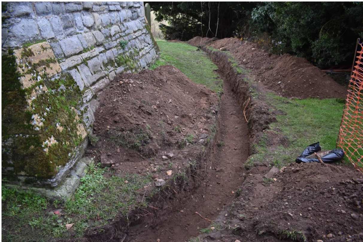
2: Service trench for water main around the church tower
