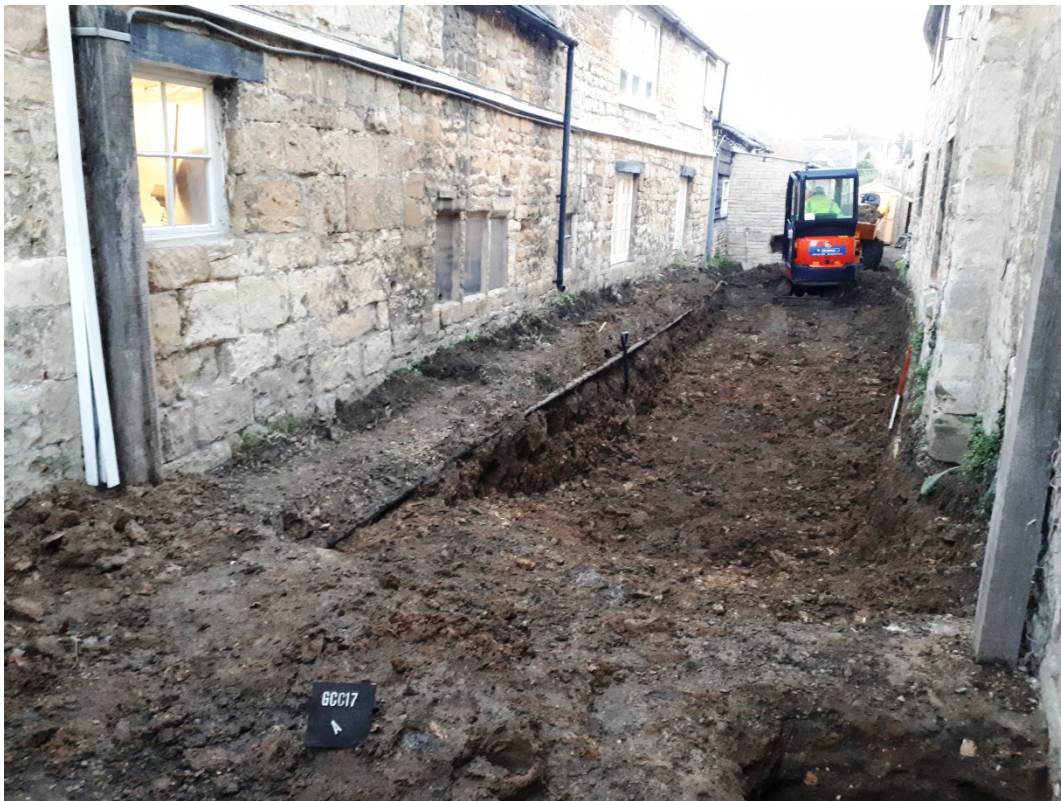
1: Excavation of the new access ramp between the buildings
