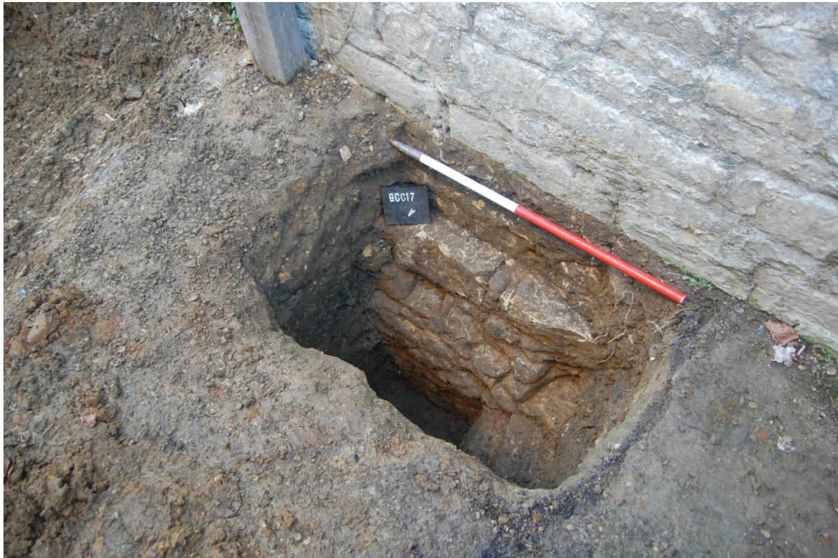
3: Remains of offset stone walling (3 and 4) below neighbouring building
