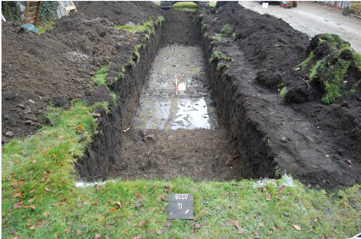
1: Trench 1 looking south showing the level of the groundwater
