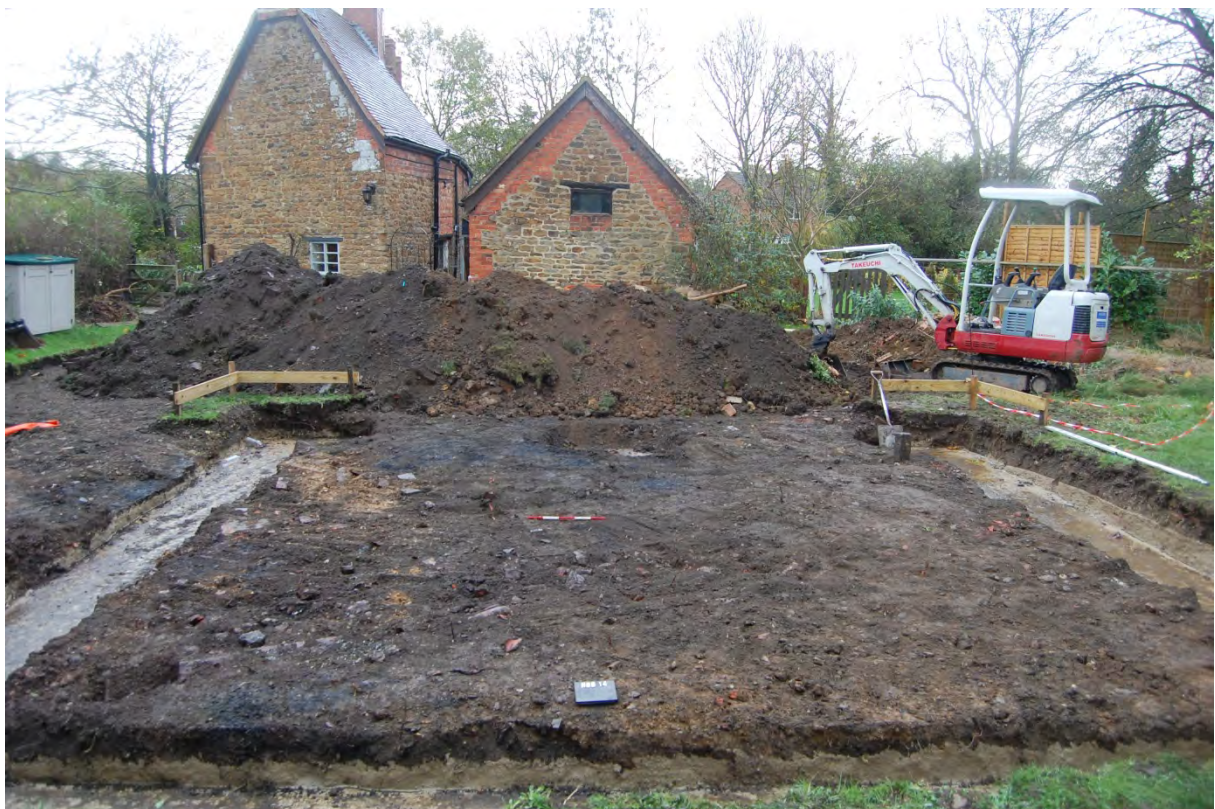
Fig 6:. Ground reductions (internal)
