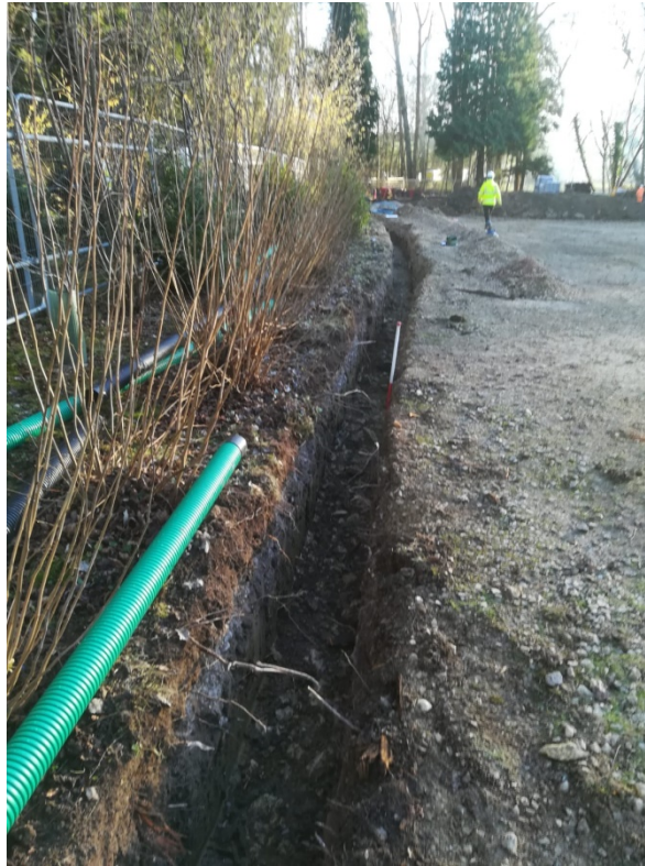
3: View south along Trench 3 at eastern edge of site
