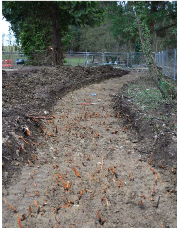
1: Initial topsoil stripping in Trench 1 looking west showing (3) in foreground
