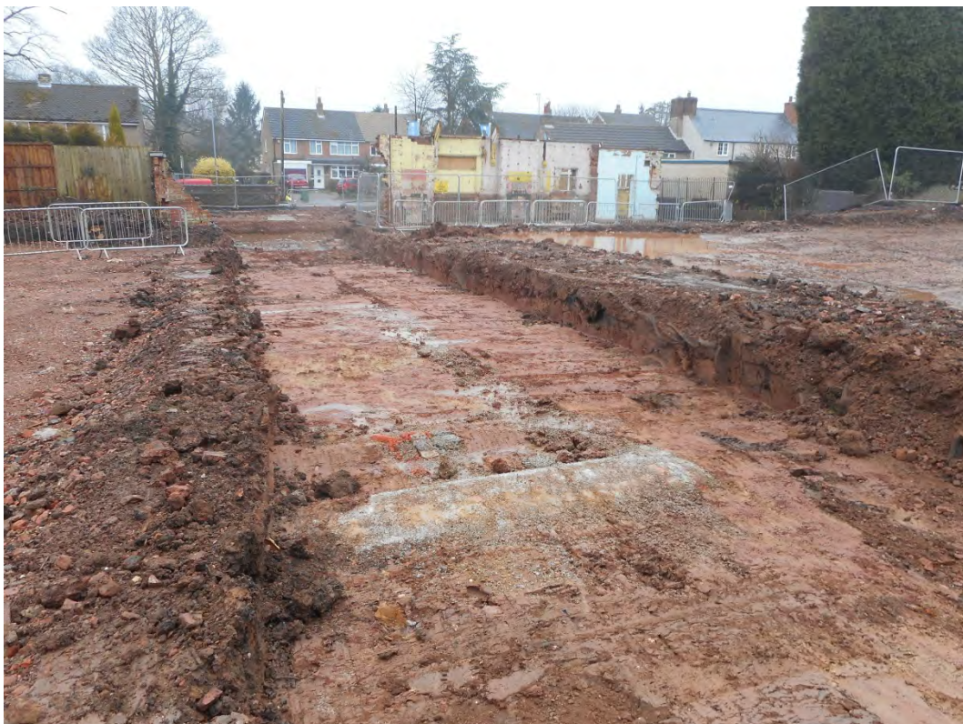
2: Access Road, looking north
