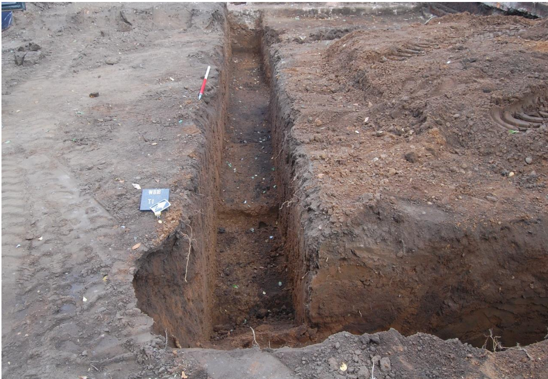
2: Foundation trench 1, looking north-west
