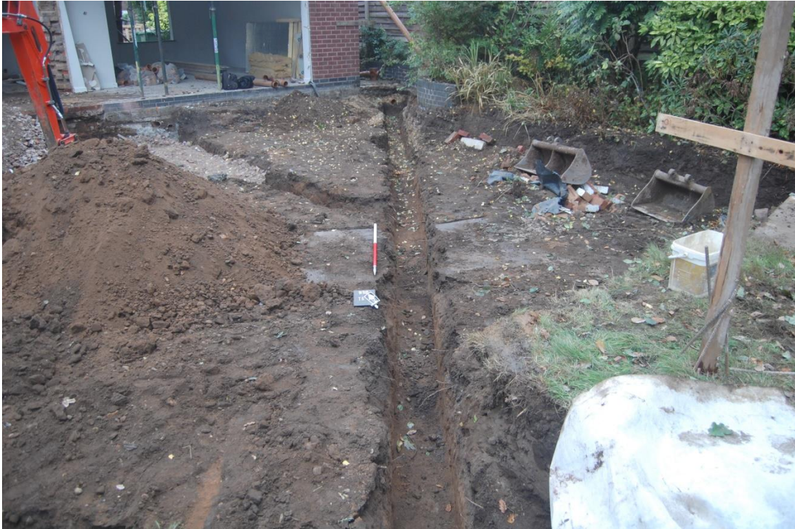
3: Drainage trench 5, looking north-east
