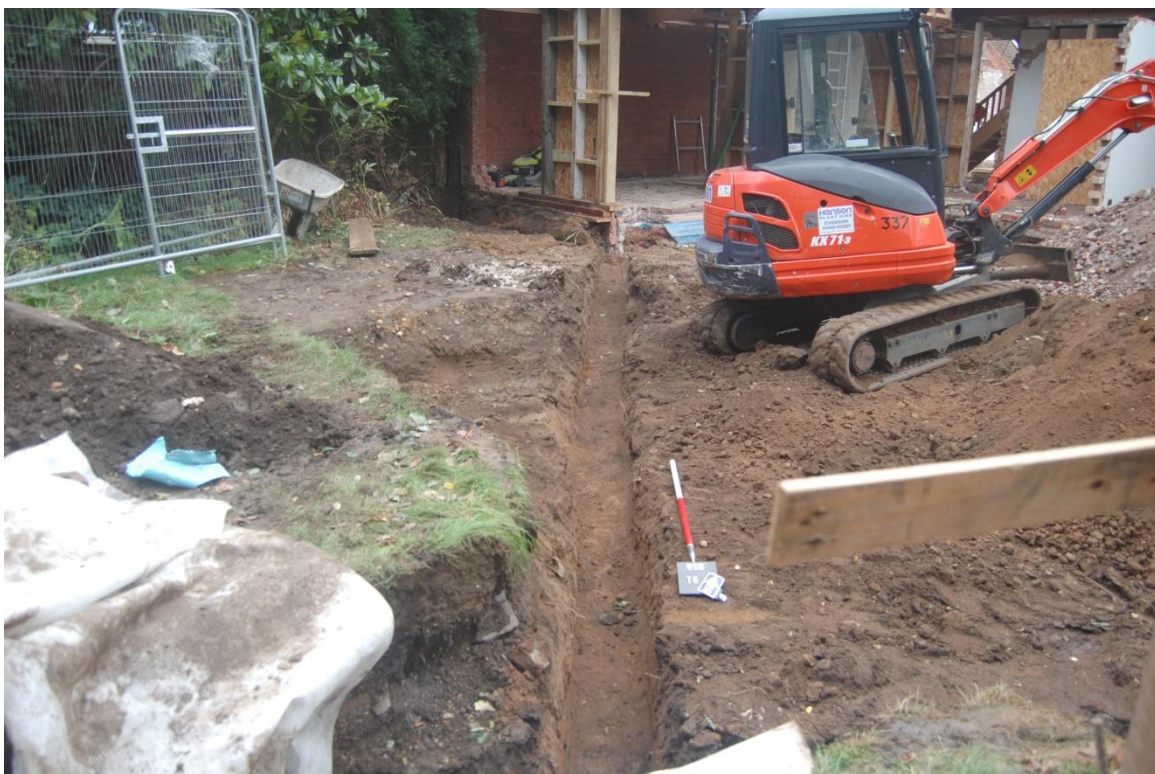
4. Draining trench 6, looking north-west
