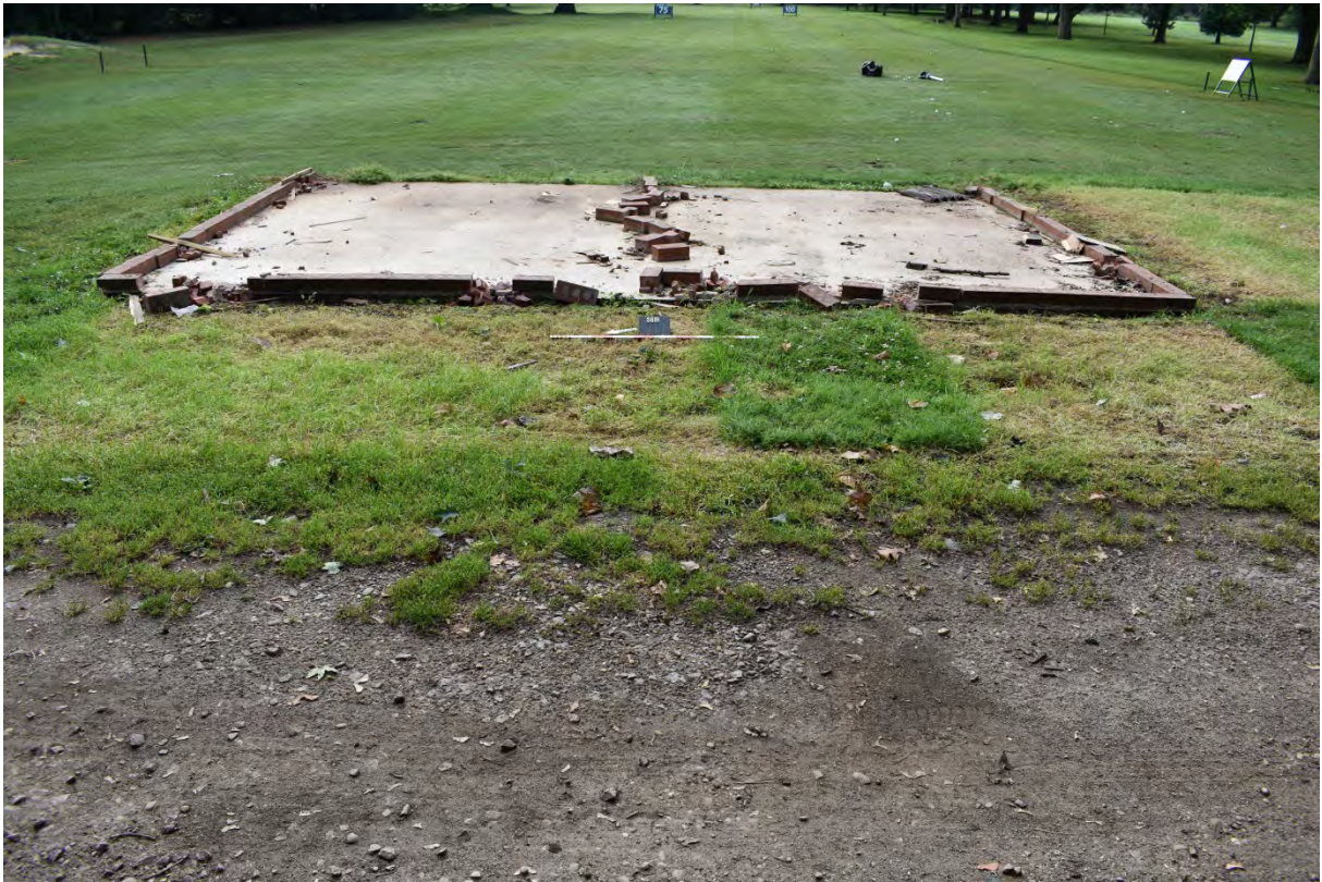
1. Pre excavation with existing building foundations (3)
