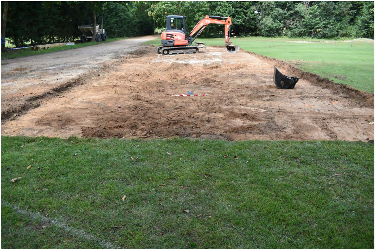
2. Area Stripped, looking NE
