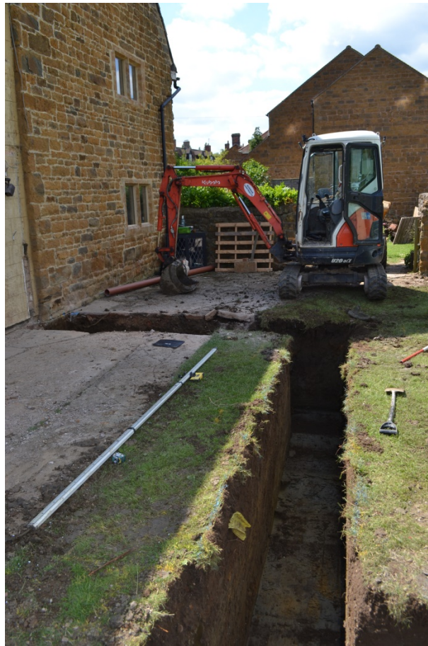
1: Observed trenches and gable end of the house
