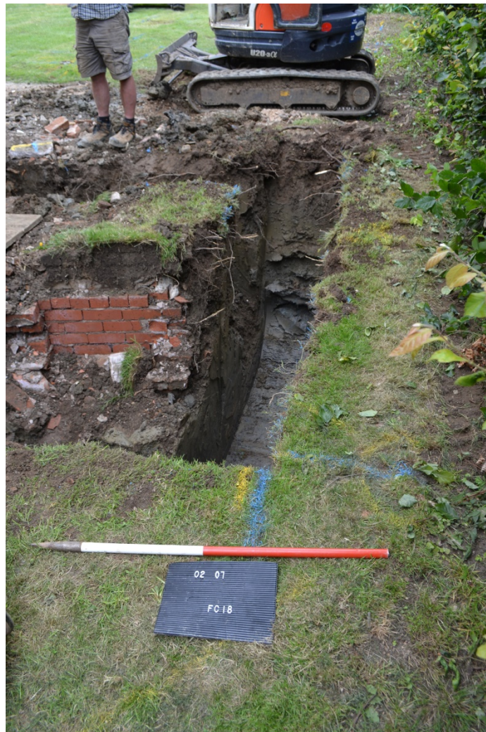
3: Observed trenches to north of the house showing pre-existing services
