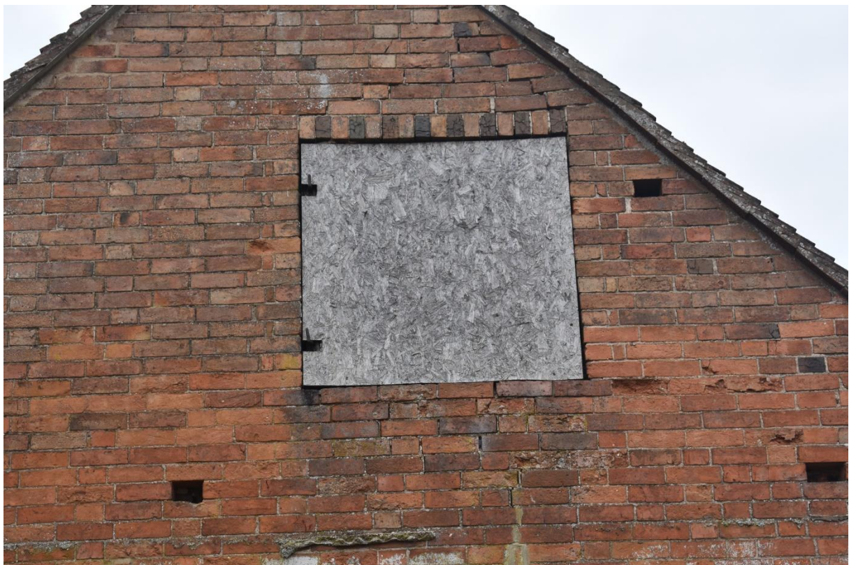
8: Detail of pitching window opening on upper part of gable
