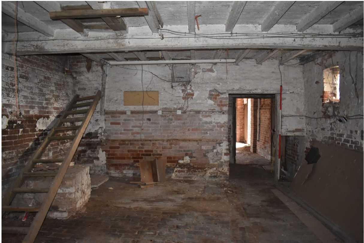
19: Room 3, looking east
