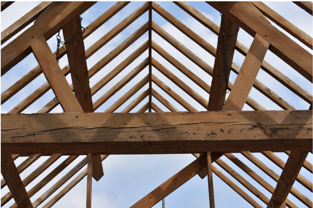
62: Raking struts and tie beam of roof truss
