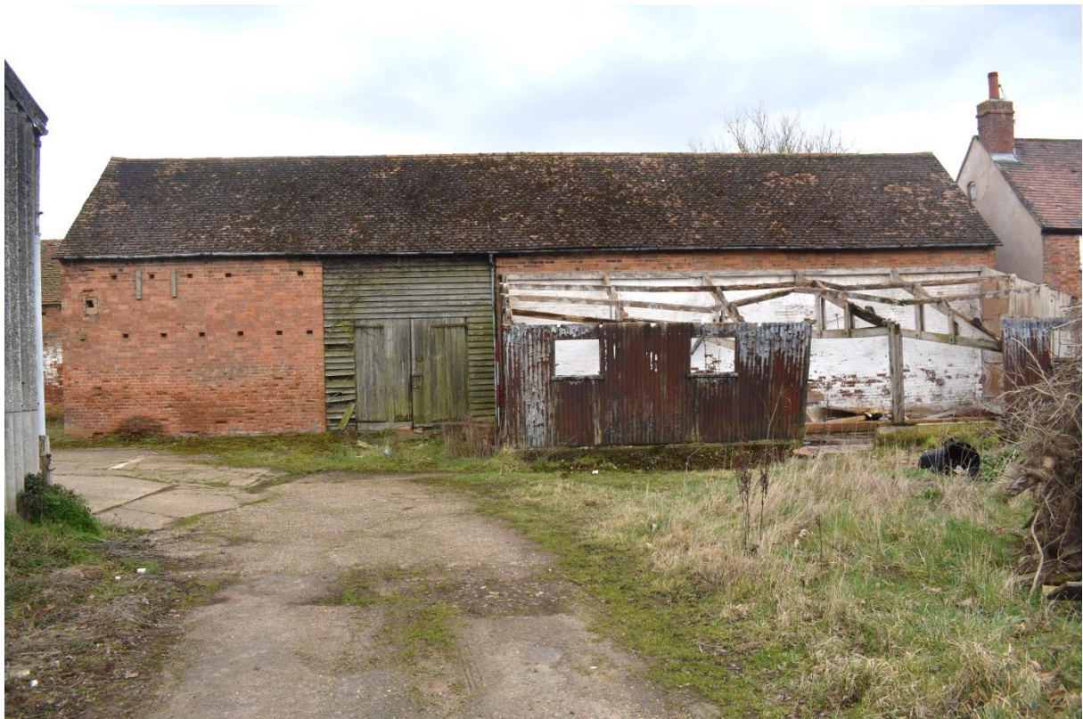
2: North side of barn and dilapidated corrugated structure
