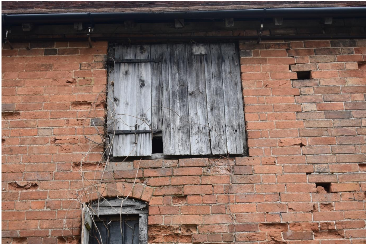
17: Pitching window and change in brickwork to the right
