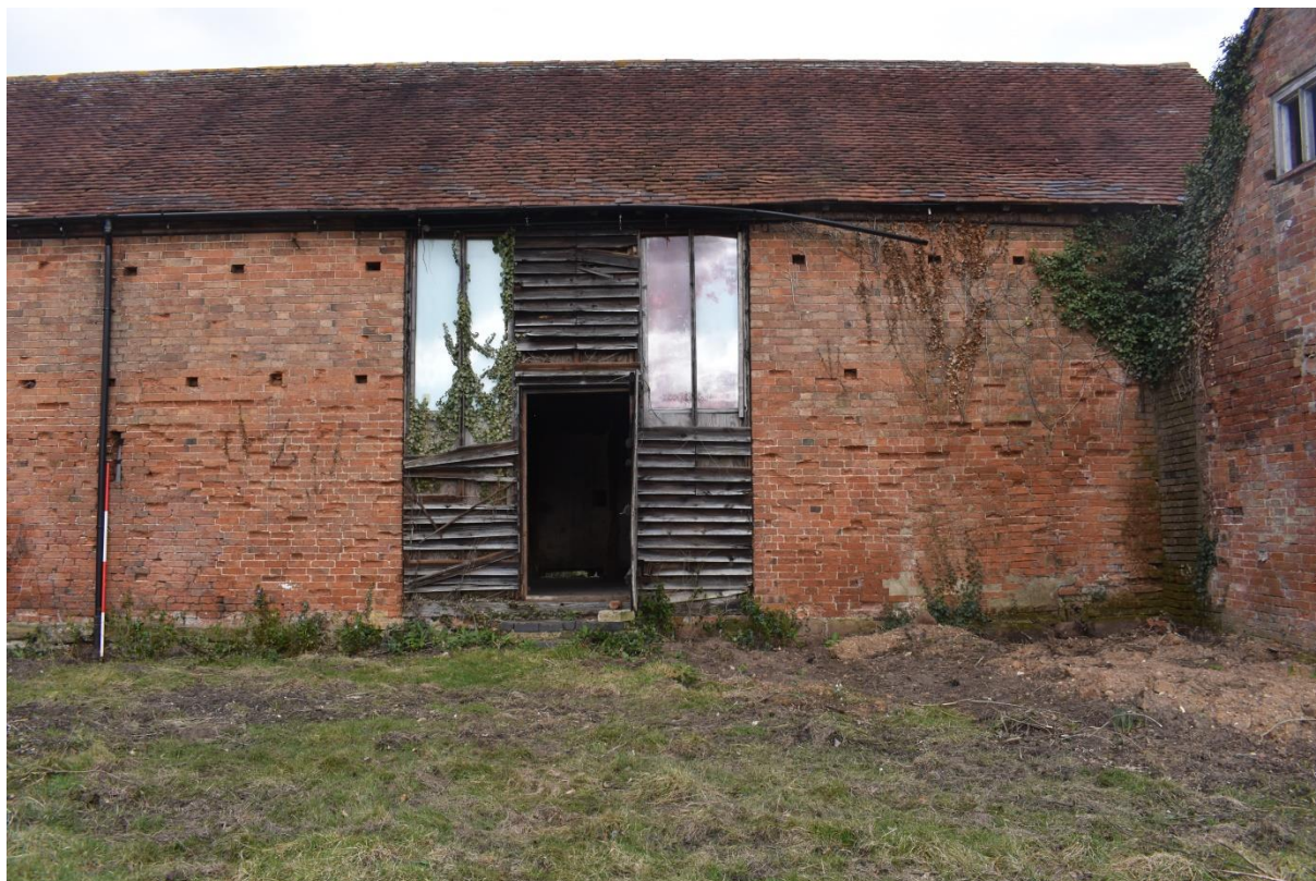
6: South side of barn
