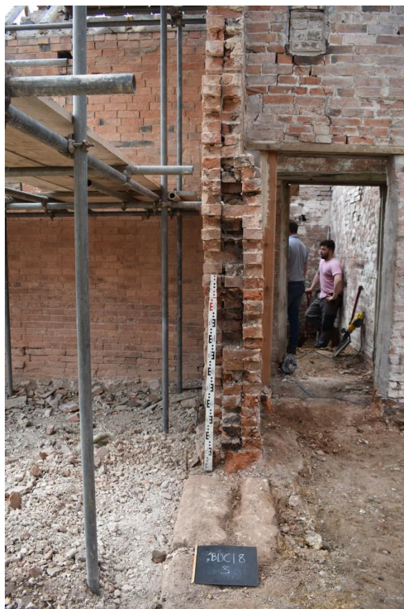
44: Stone footing 3 below brick gable wall
