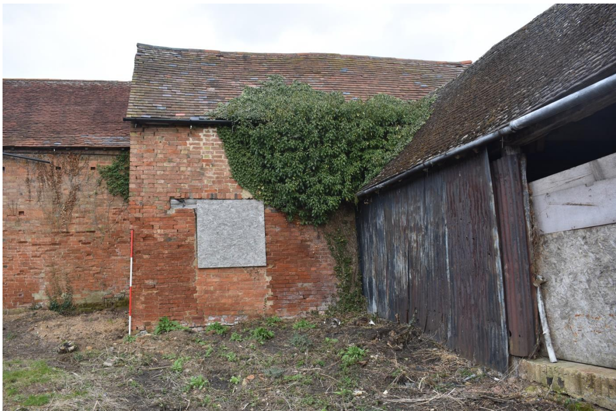
24: Building B, south wall with partly-blocked doorway
