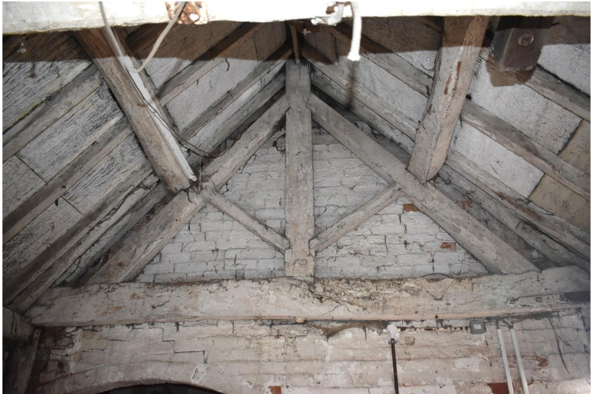
37: King-post roof truss at north end of Room 6
