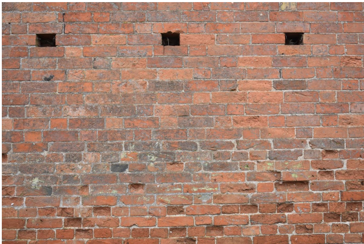
5: Detail of brick bond and ventilation holes
