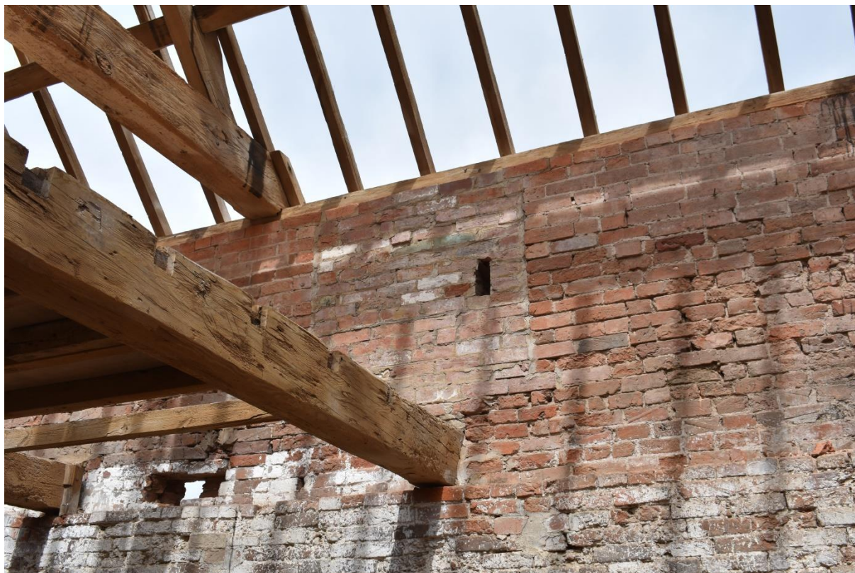
66: Chamfered edge of beam with blocked window above
