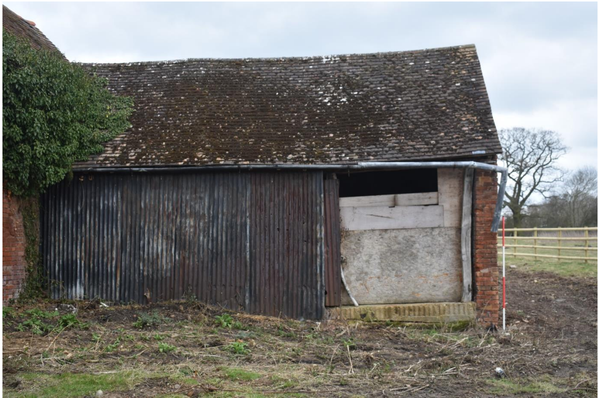
27: Building B, shelter shed, west side
