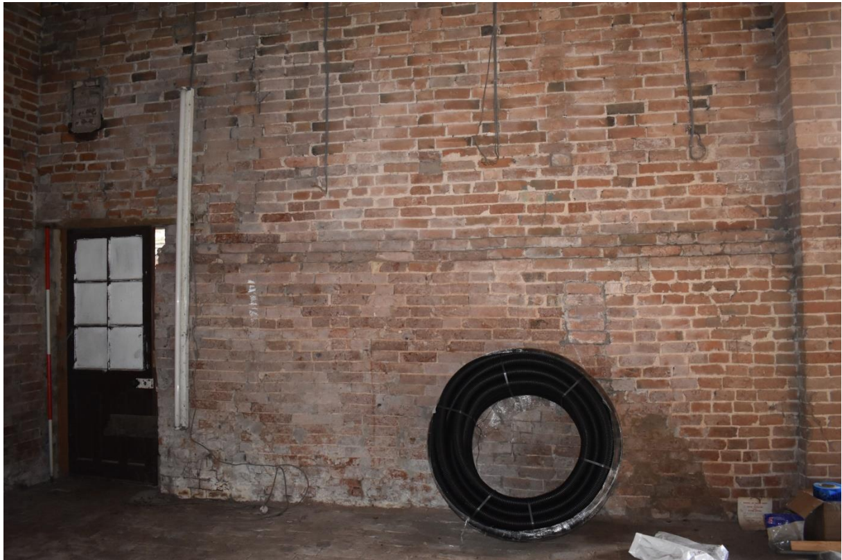
13: South wall of barn showing stepped-in brickwork and inserted door
