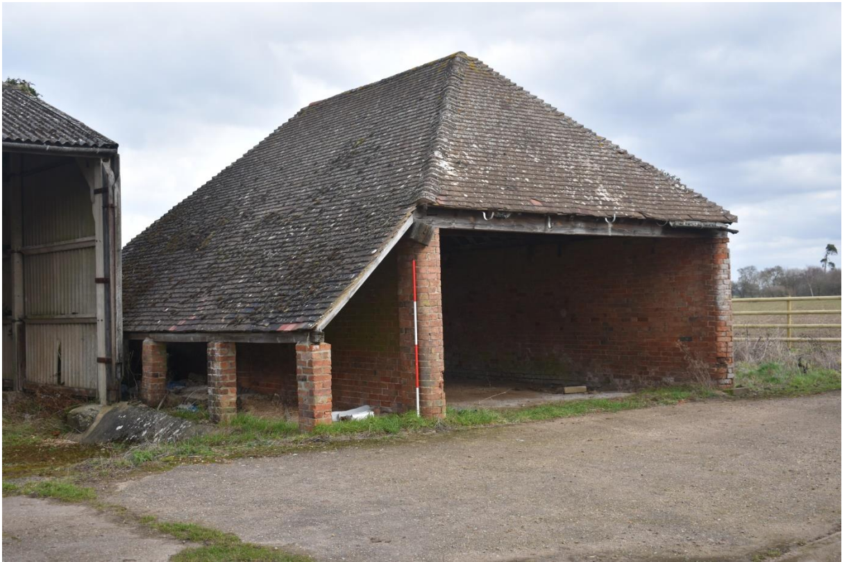
39: Building C with additional lean-to on west side
