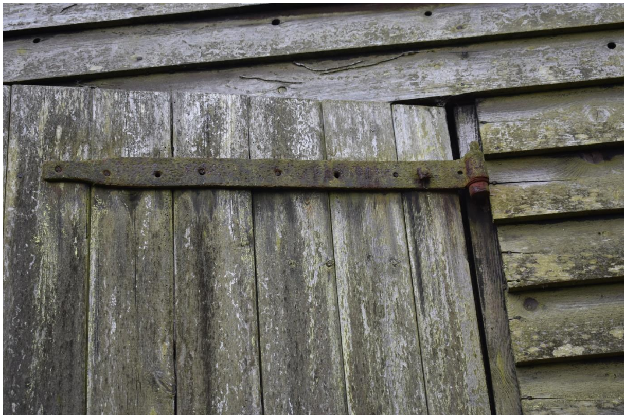
4: Detail of strap hinge on iron pintle
