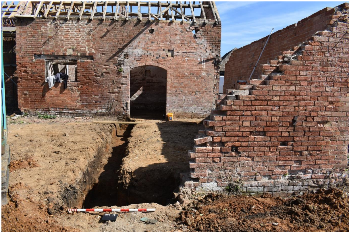
59: Trench for new footings on former edge of Room 6
