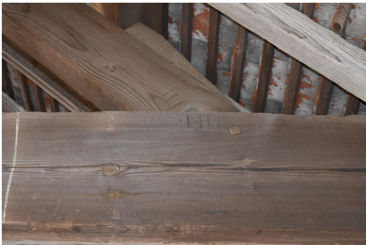
42: Carpentry marks (III) in Building C
