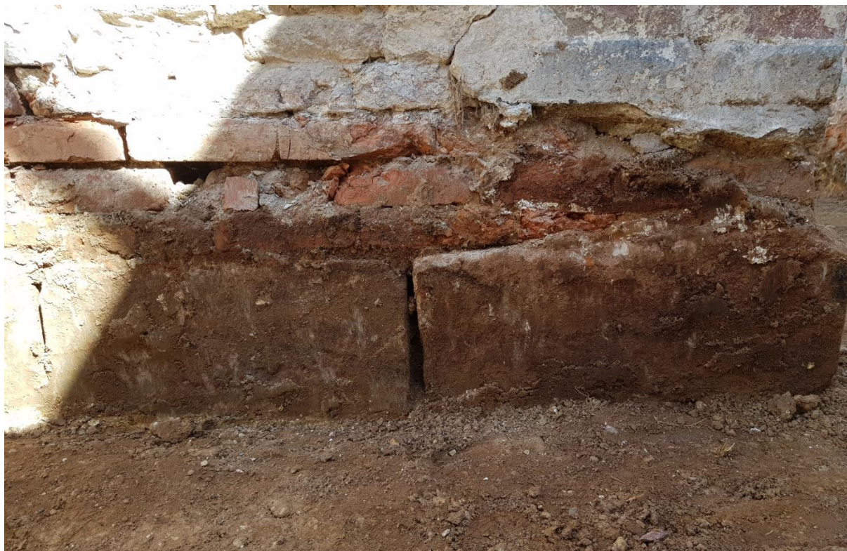
49: Footings 11 exposed after full ground reduction below N-S wall
