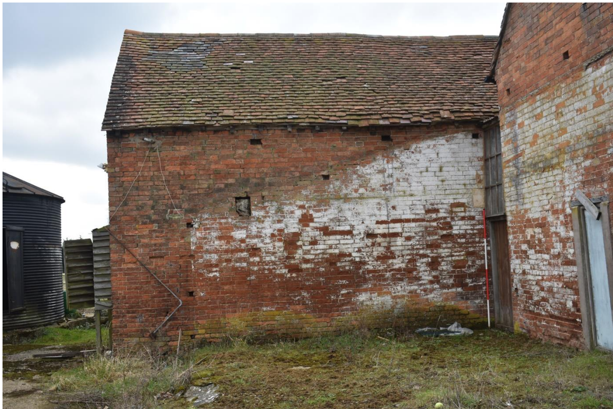
21: Building B, north side, paint and roof-scar of former lean-to
