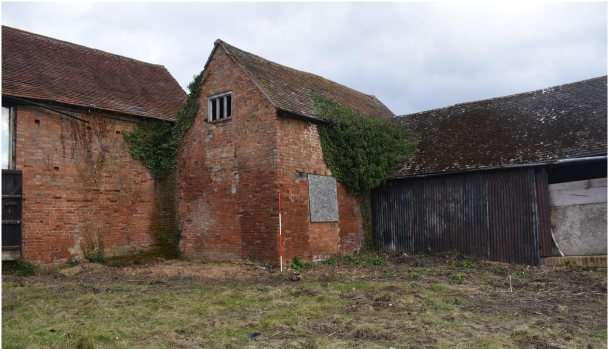
25: Building B, looking north-east
