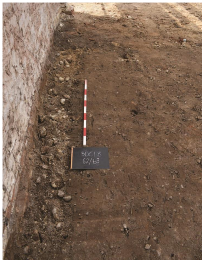
46: Footing 62/63 against south wall of barn
