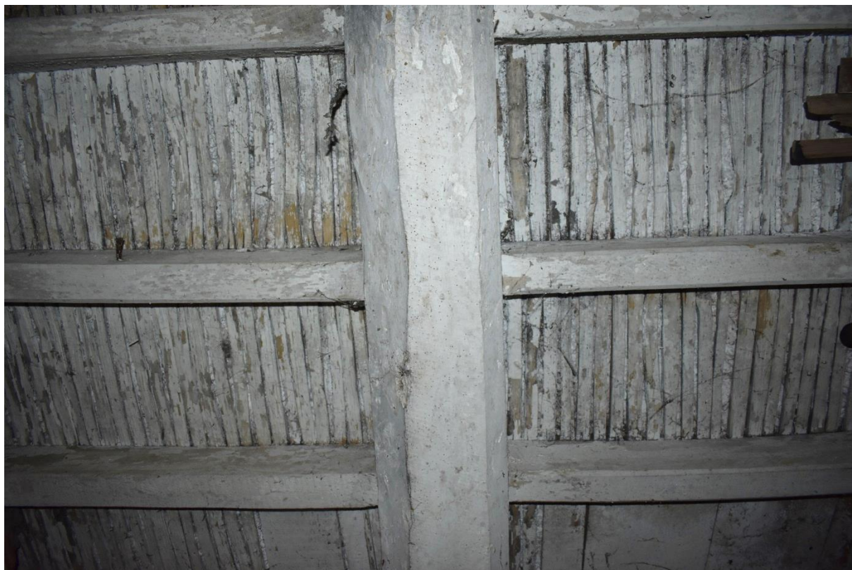
31: Ceiling of Room 4
