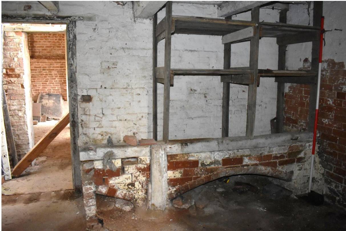
29: Building B, Room 4, looking north
