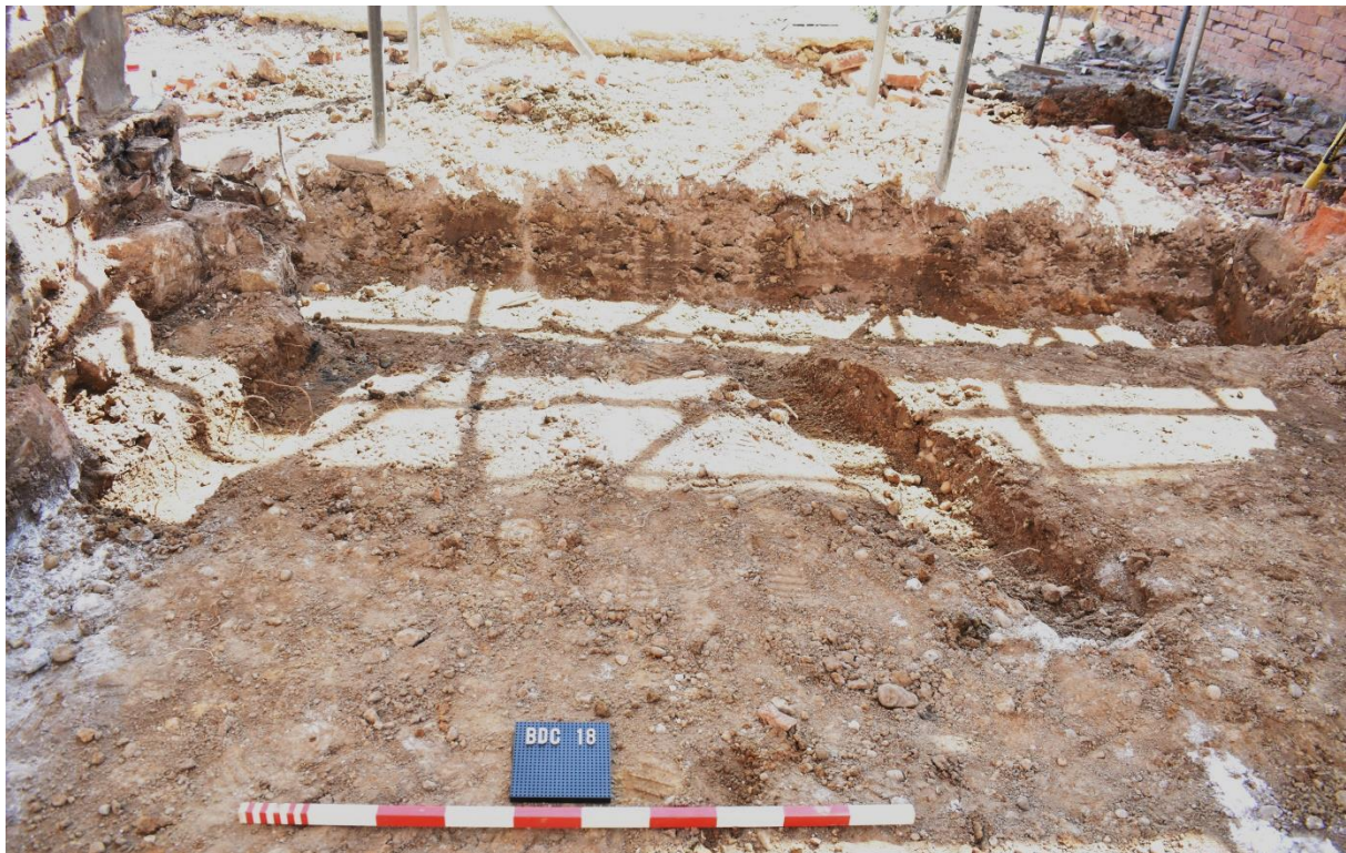
43: New foundation trench at west gable of barn and service trenches
