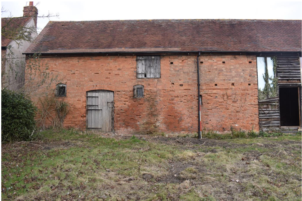
14: South wall of cow house
