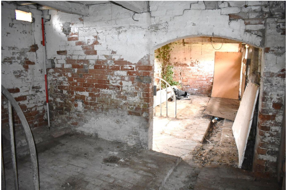
35: Building B, Room 5, looking south into Room 6
