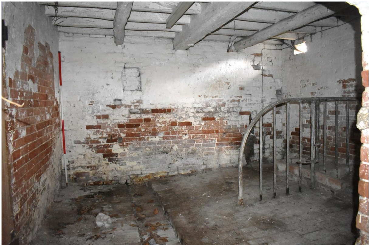
34: Building B, Room 5, looking north
