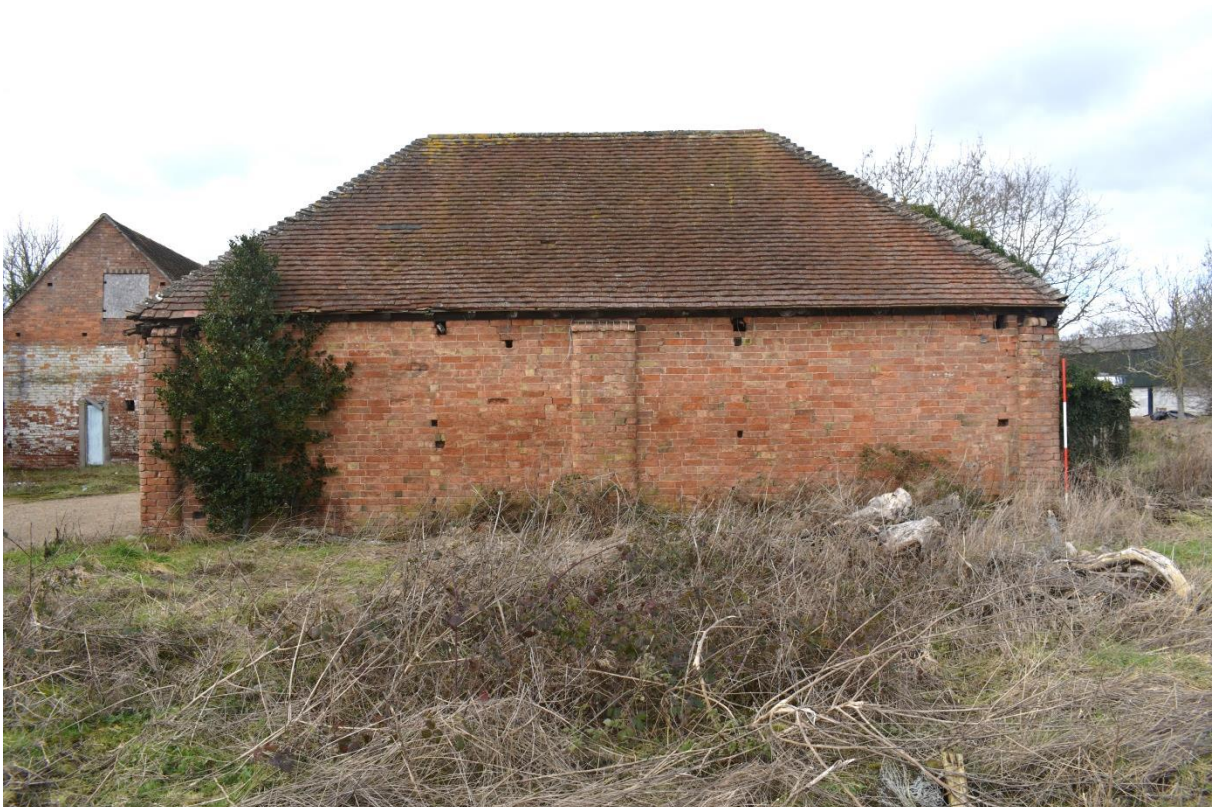
40: East side of Building C, note slight buttresses
