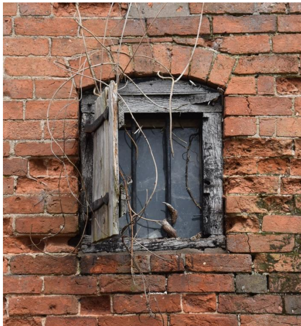
16: Detail of small, barred window
