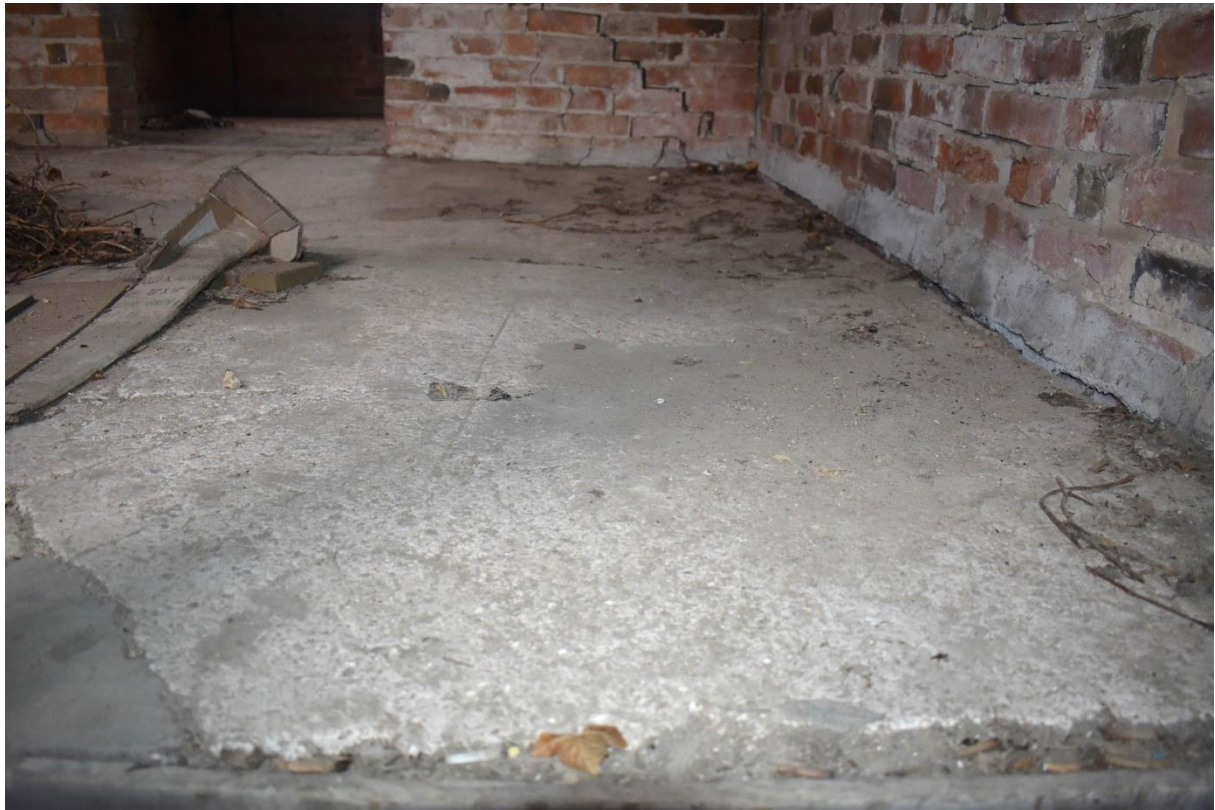
33: Building B, first-floor lime-ash floor
