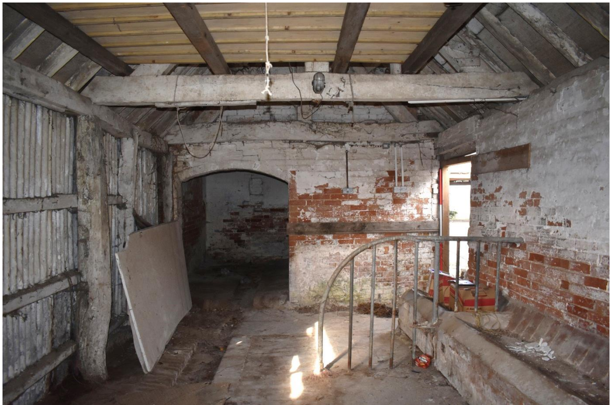
36: Building B, Room 6, looking north
