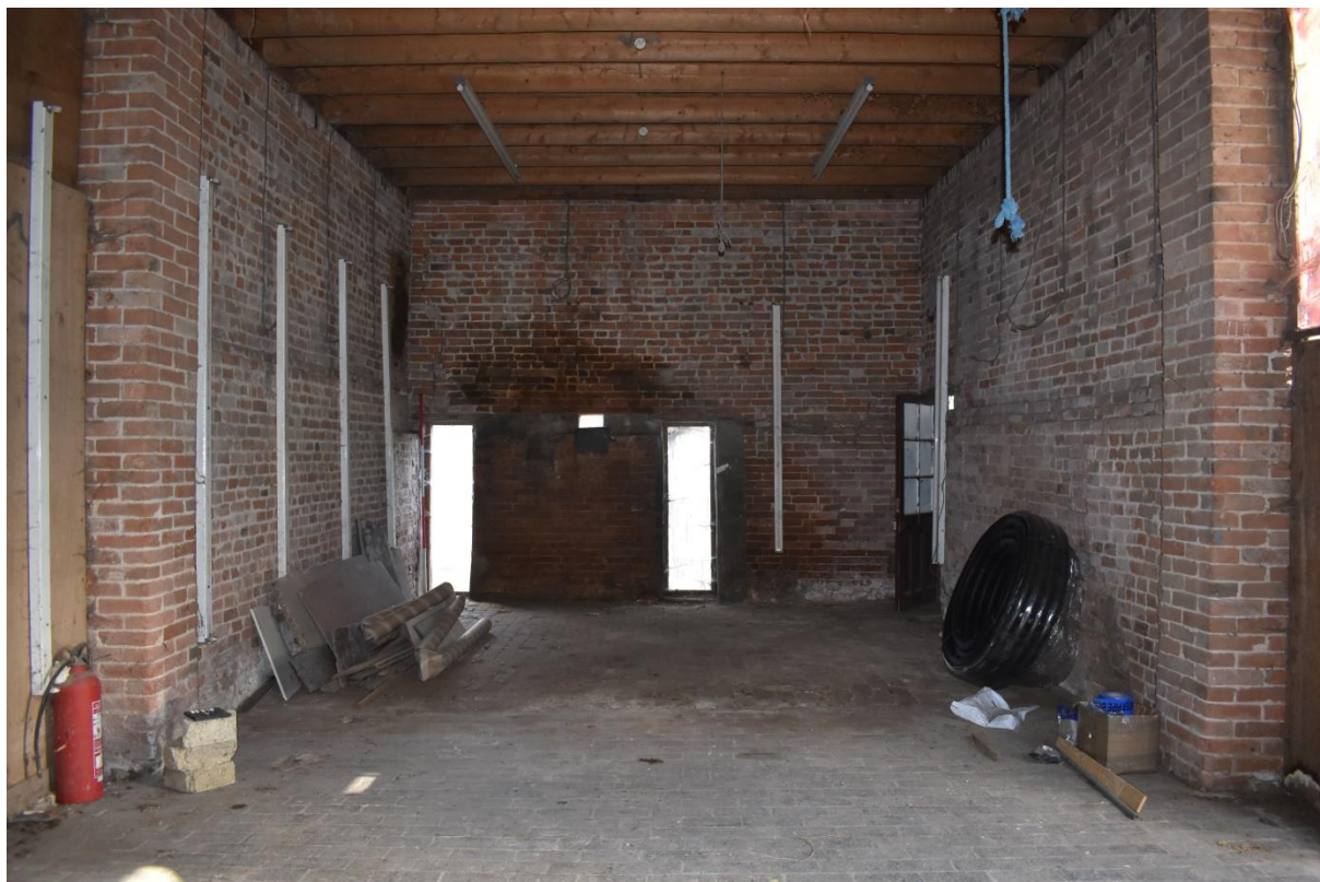
10: Interior of barn, looking east
