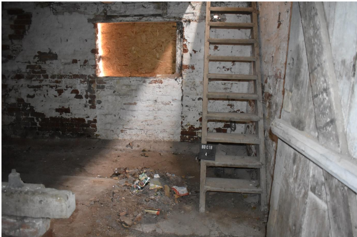
30: Building B, Room 4, looking south
