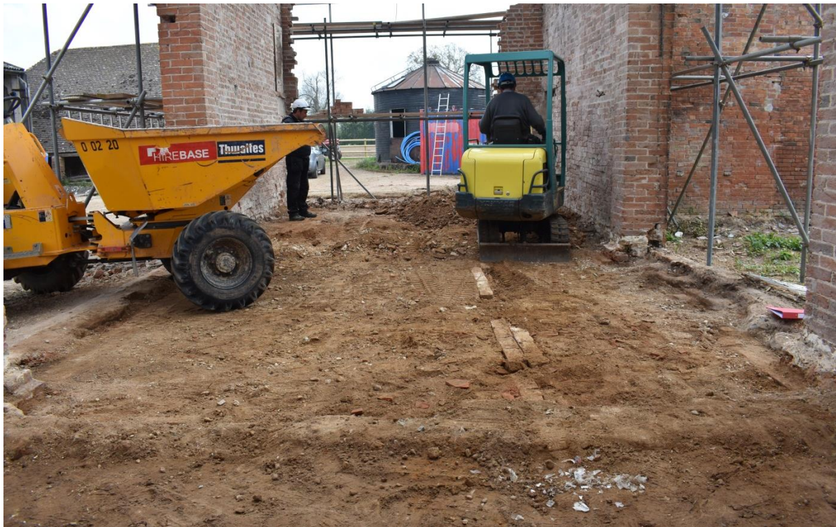
45: Wall 10 in foreground, brick wall 4 running east during initial ground reduction
