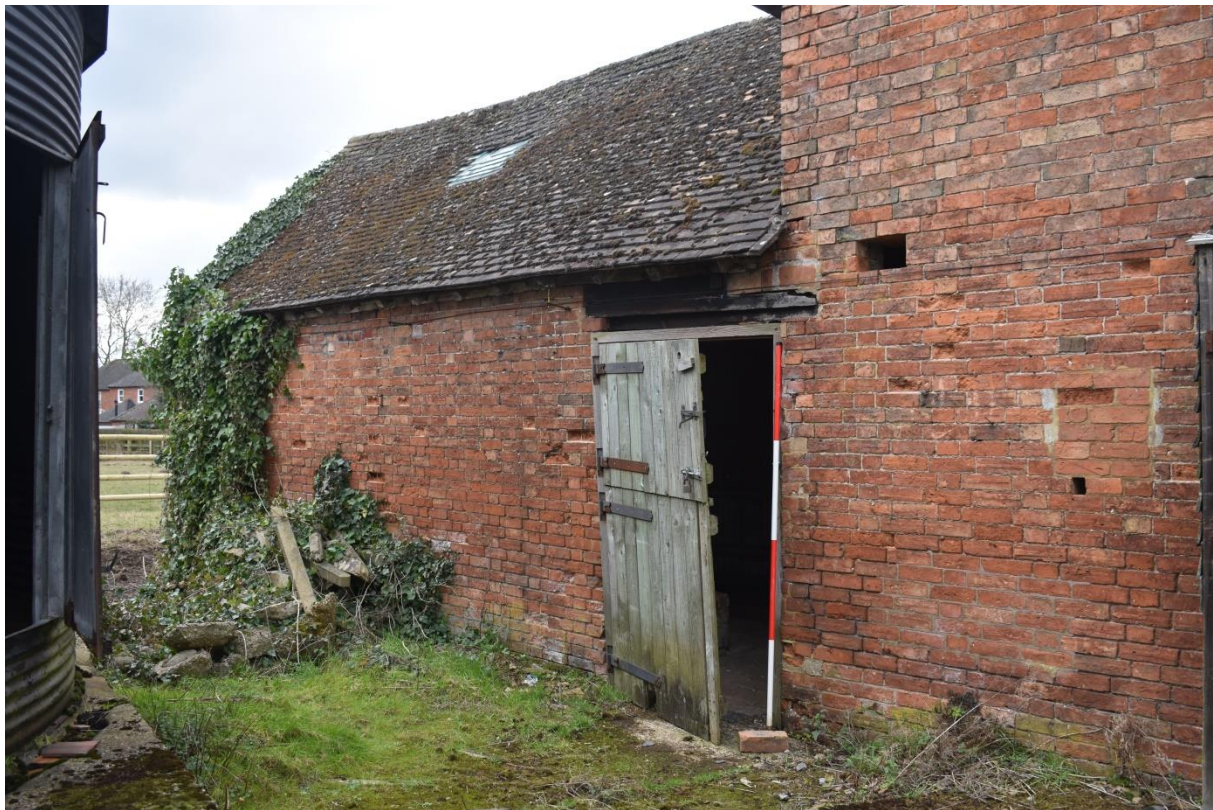
23: Building B, east wall of shelter shed
