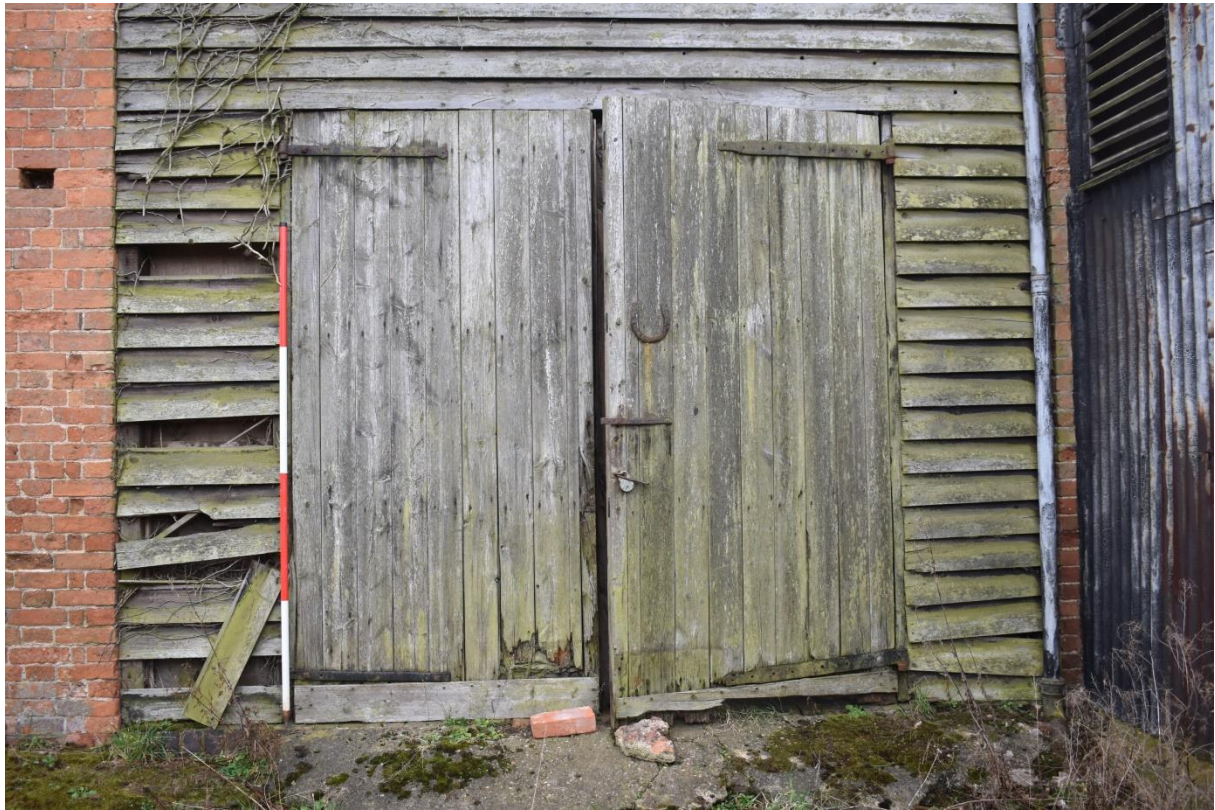
3: Detail of doors on north side, surrounded by weather-boarding
