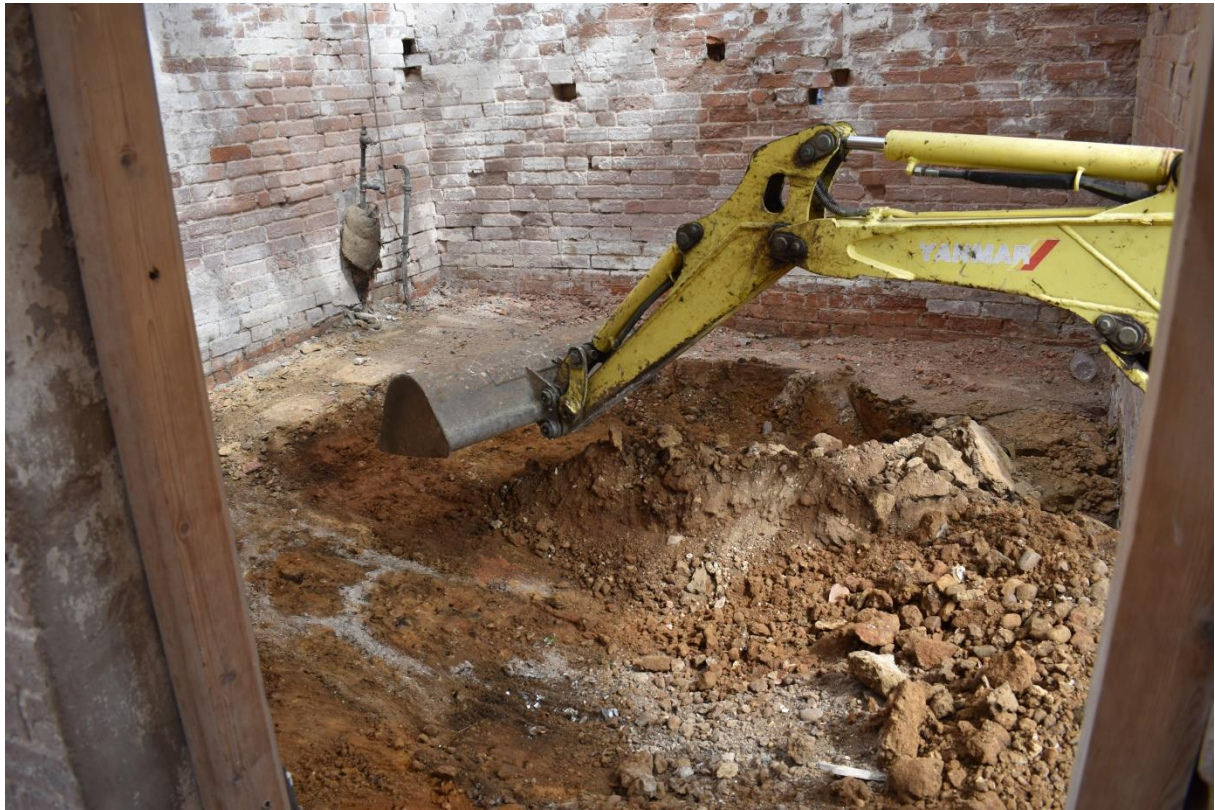
57: Ground reduction in Room 5
