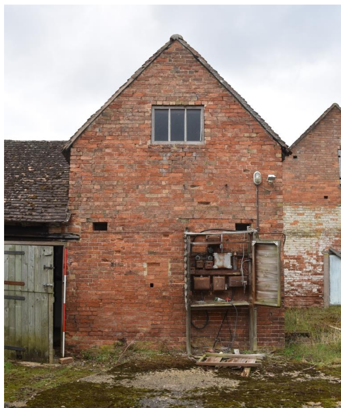
22: Building B, east gable
