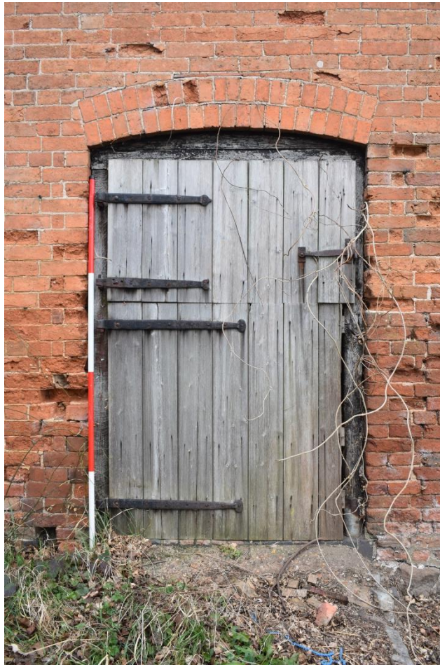
15: Detail of door to cow house
