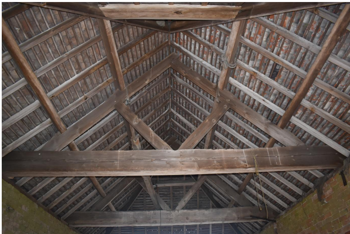
41: Roof trusses with V-struts in Building C
