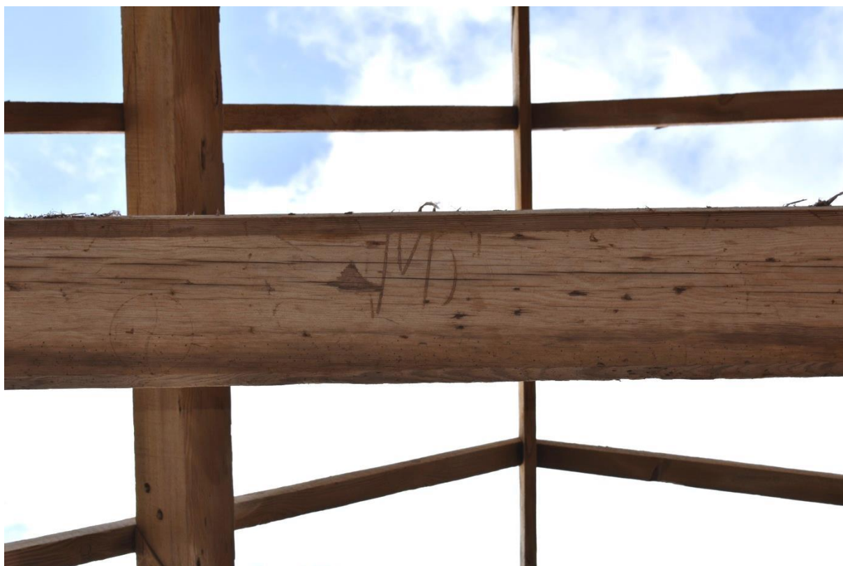
64: Incised marks on the underside of beam
