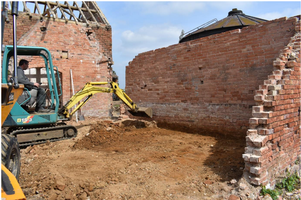
58: Ground reduction in Room 6
