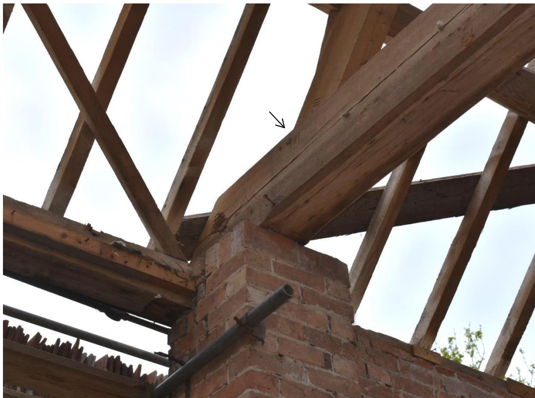
65: Carpentry mark (III) adjacent to wooden peg on tie beam
