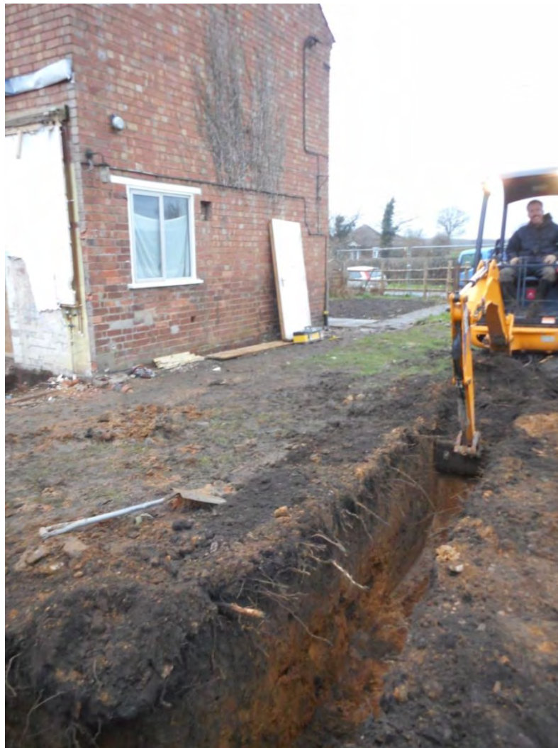
1: Excavation of foundation trench
