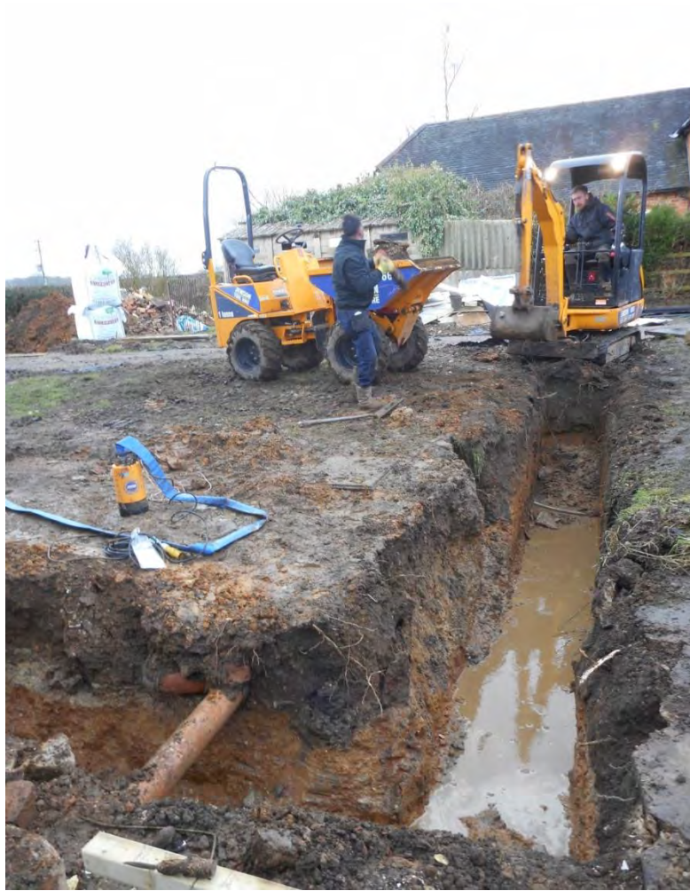
2: Excavation of trenches showing services and deposit sequence
