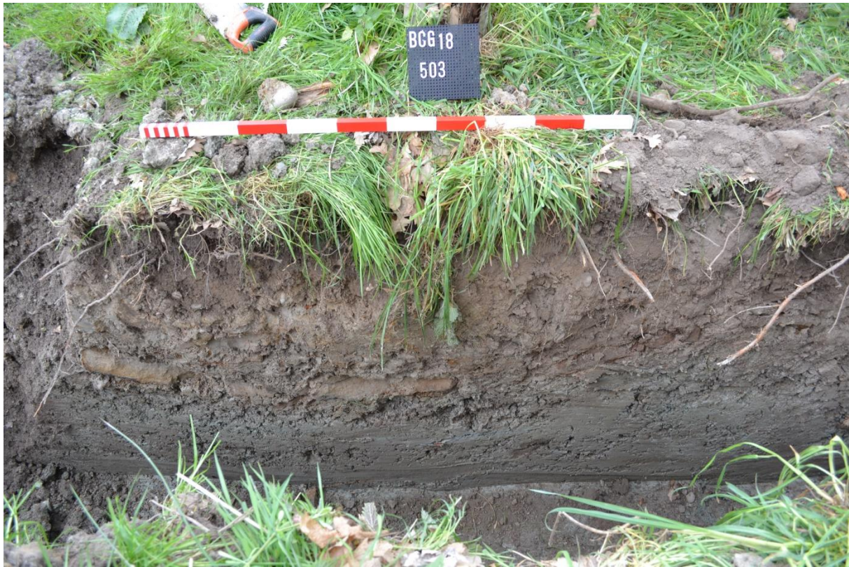
19: Culvert 503, looking west-north-west
