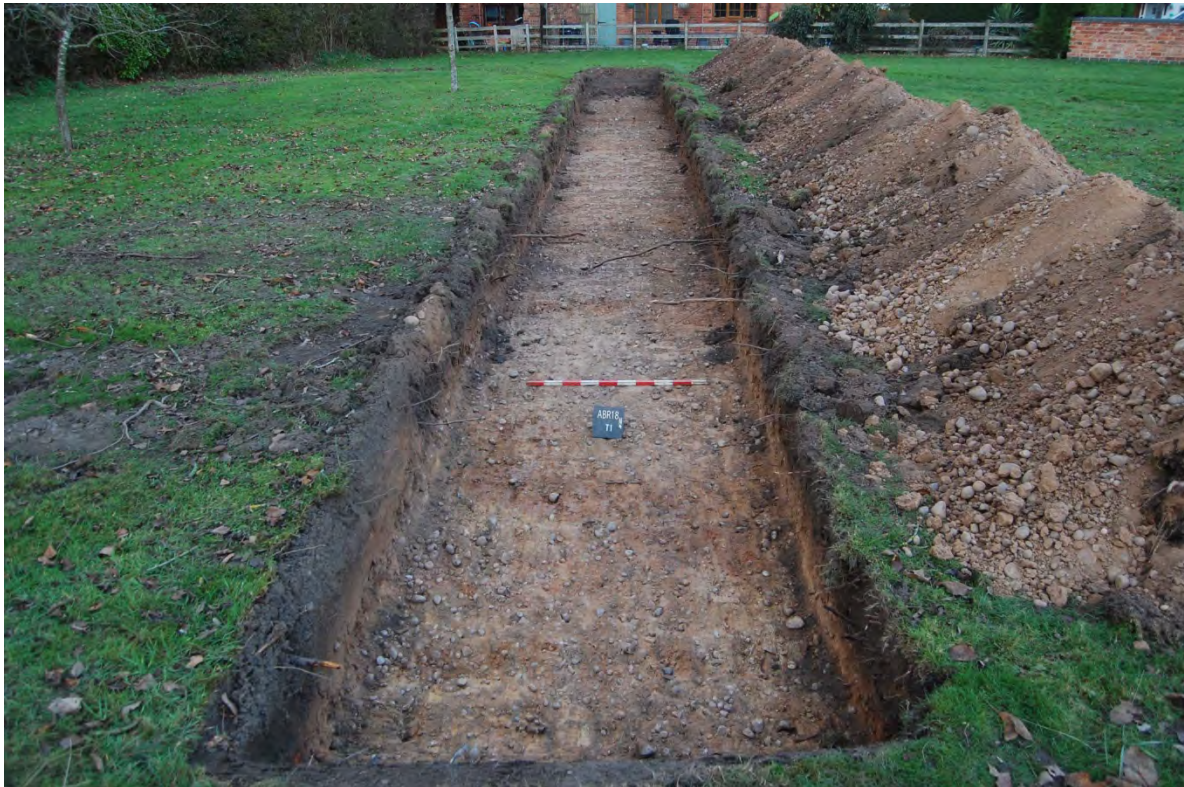
1: Trench 1, facing north east
