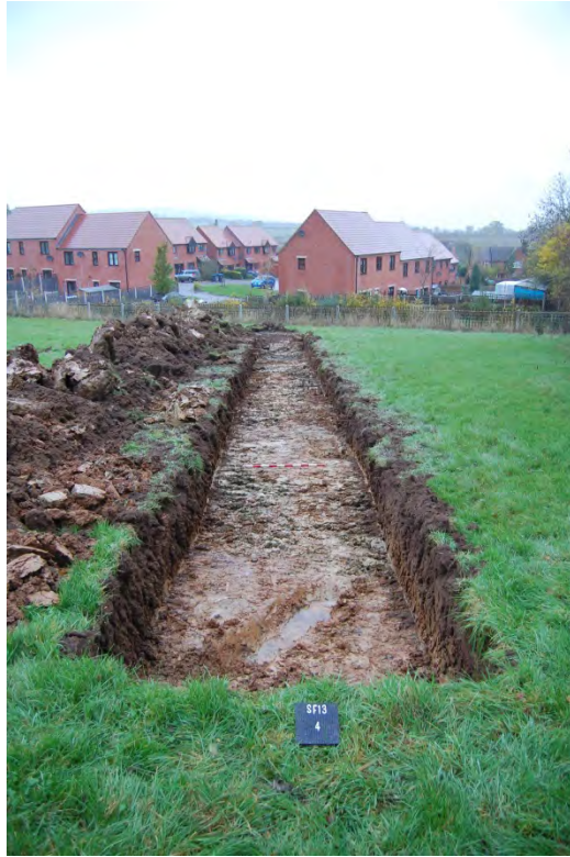
Fig 6: Trench 4 viewed from the SE
