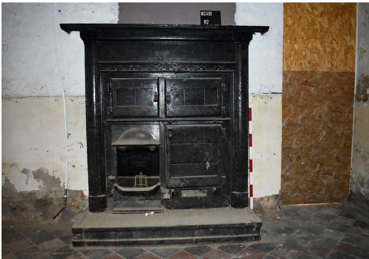
16: Cast iron fireplace and oven in rear wall of Room 2
