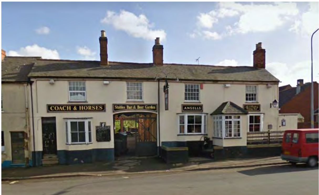
2: The front of The Coach and Horses, prior to work being undertaken (Google Streetview)
