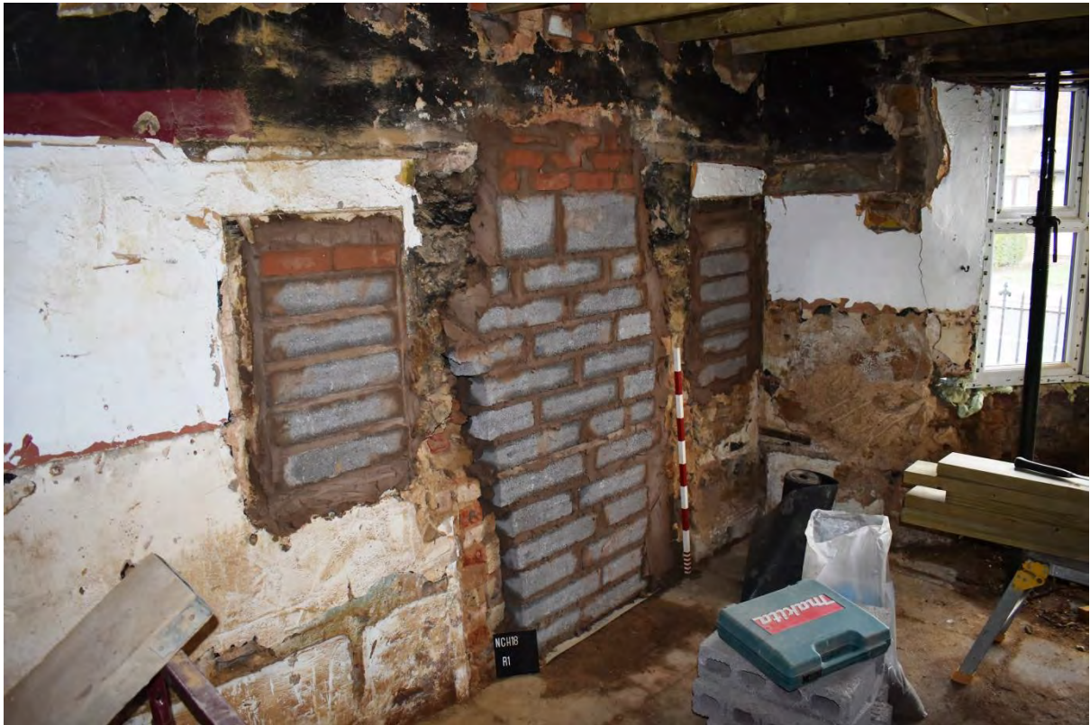
11: Blocked fireplace and alcoves in southern part of the bar (Room 1)
