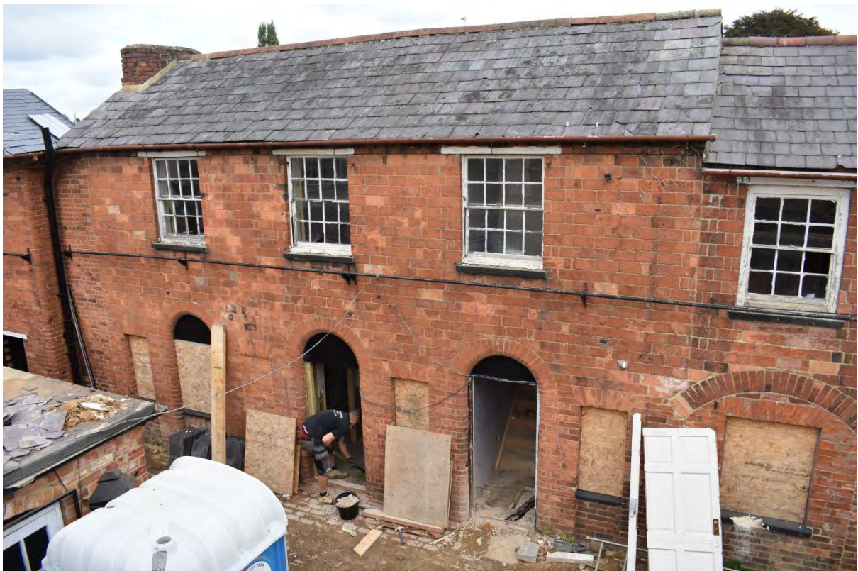
4: Phase 1 of the stables building
