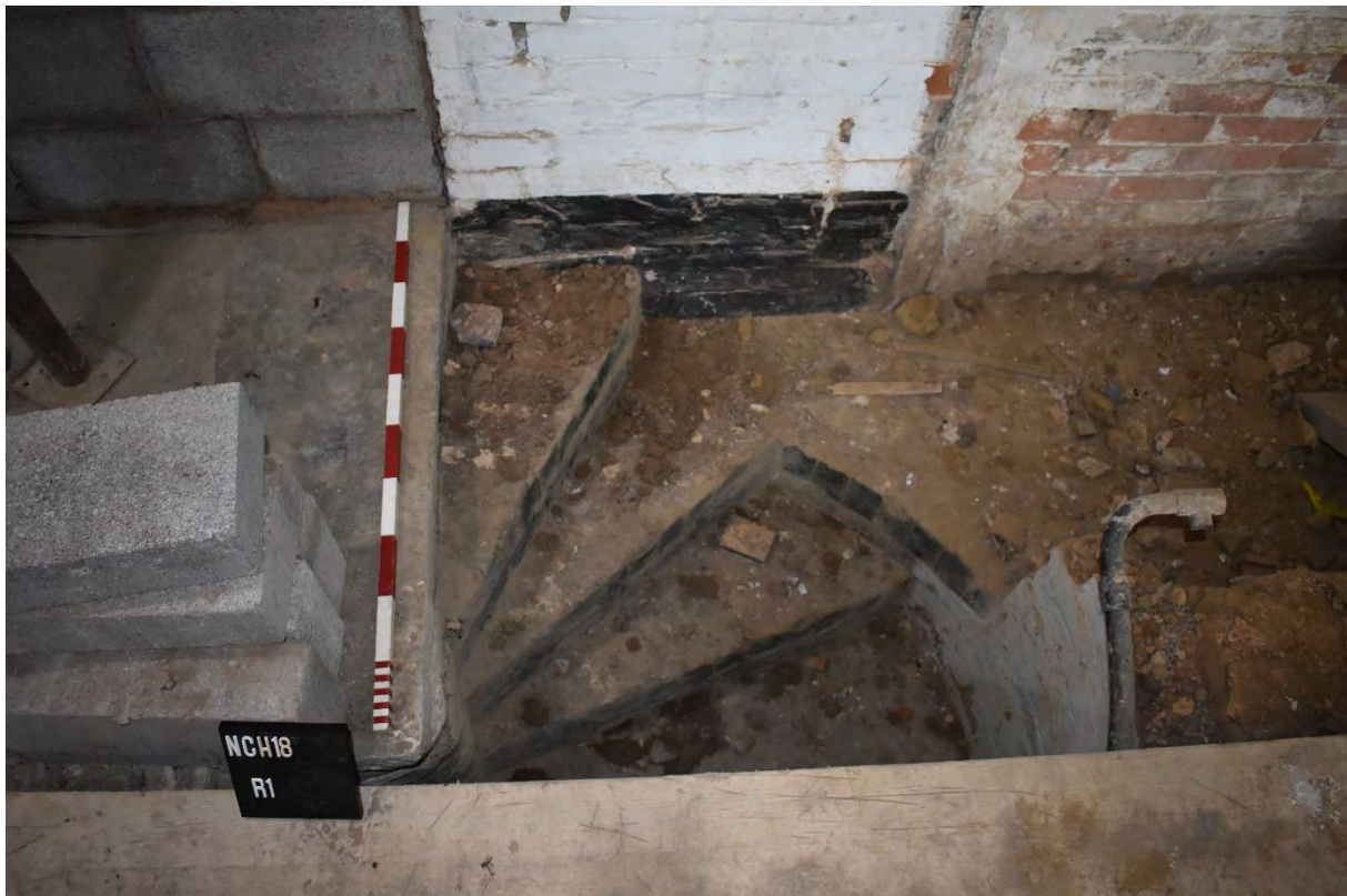
14: Upper part of spiral staircase into cellar
