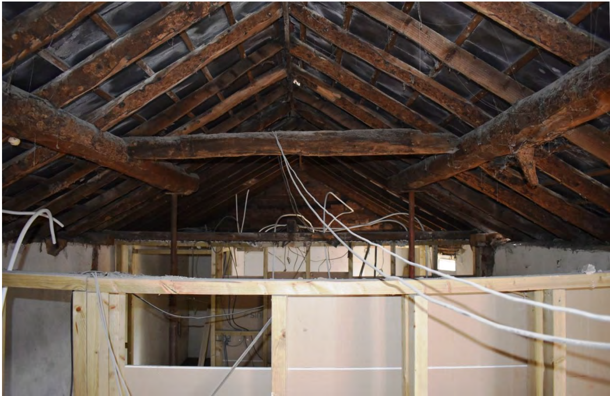
17: Roof structure of the stables
