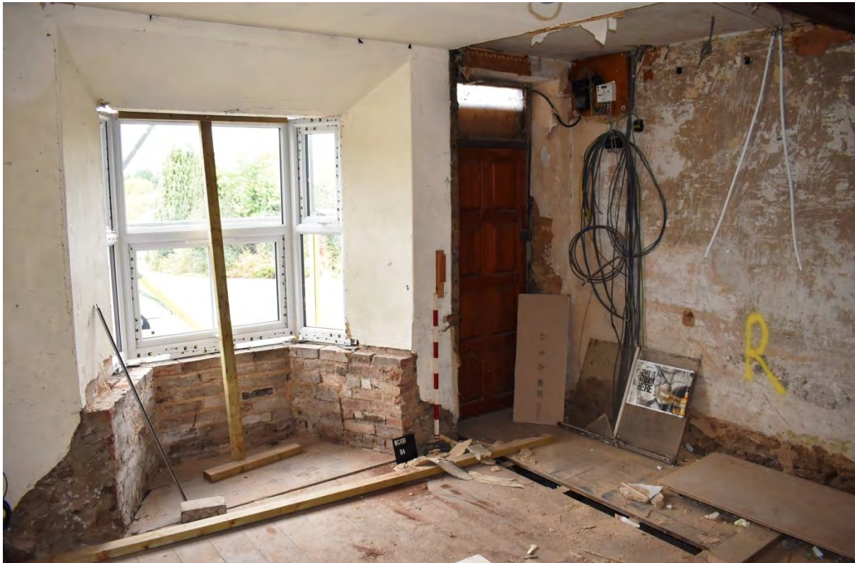
19: The replacement window and front door in Room 4
