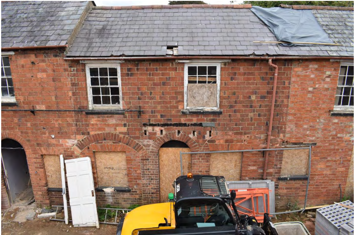
5: Phase 2 stables building
