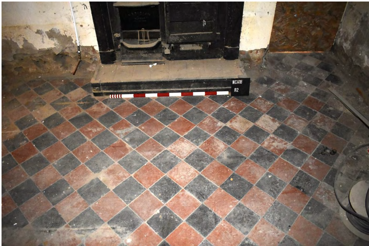
15: Tiled floor in the rear bar (Room 2)
