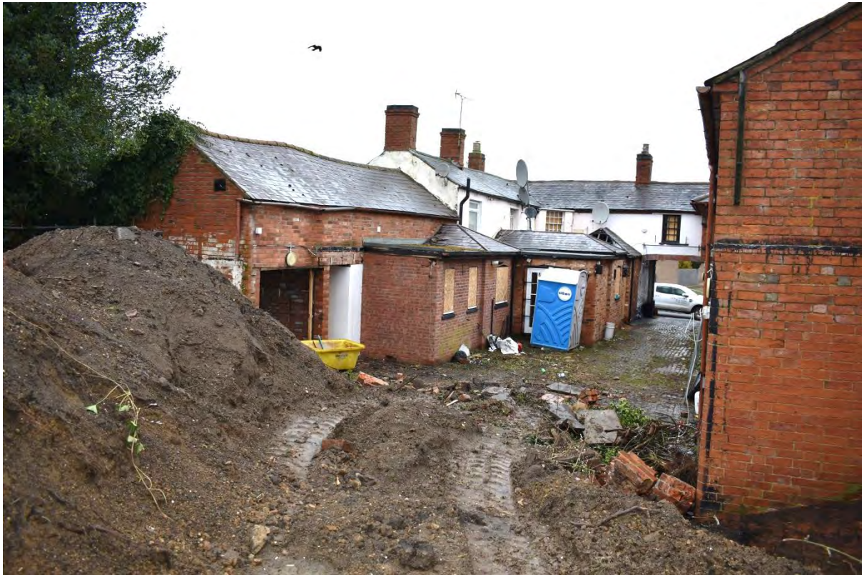
7: The south range showing the rear extension
