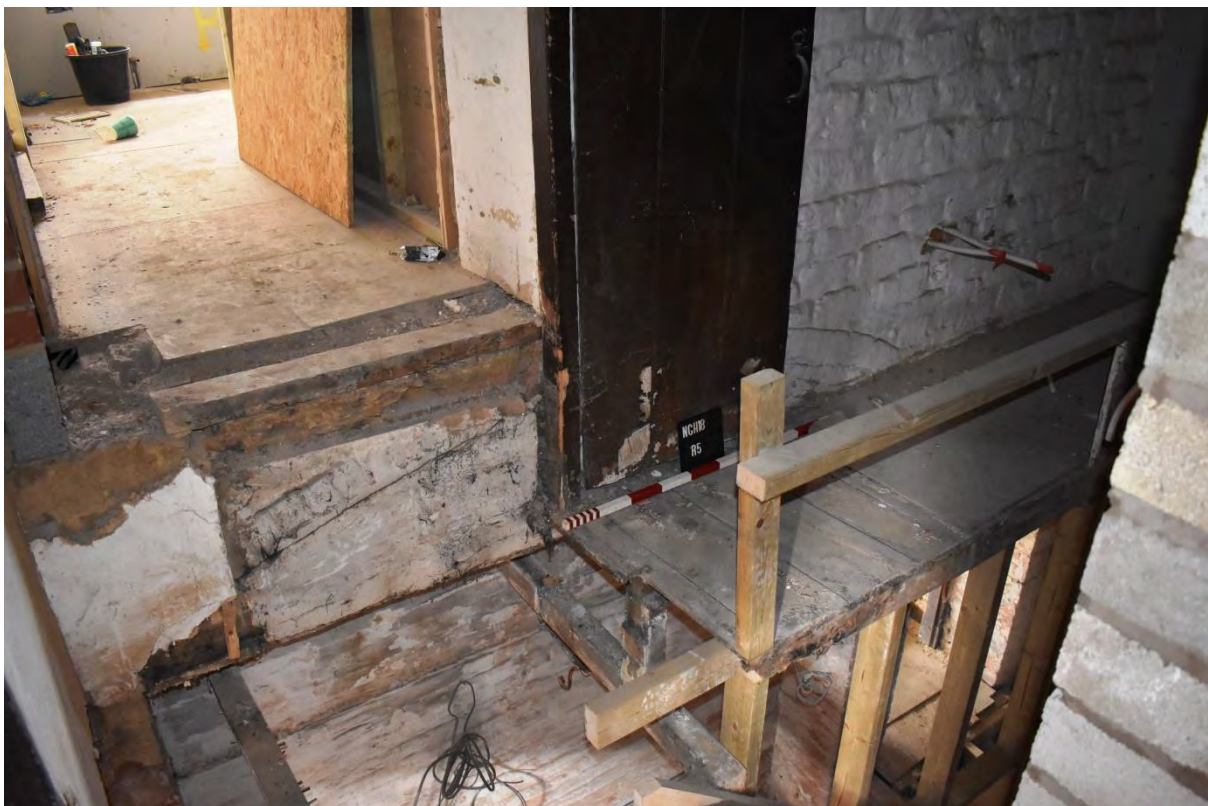
20: Original rear stone wall of the adjacent building and blocked archway visible on the half landing (Room 5)
