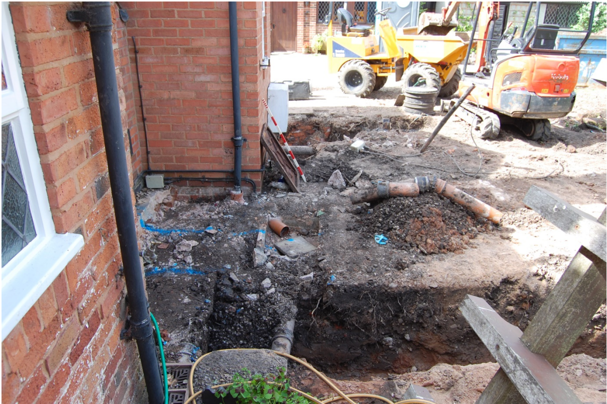
1: General view of trenches, looking north
